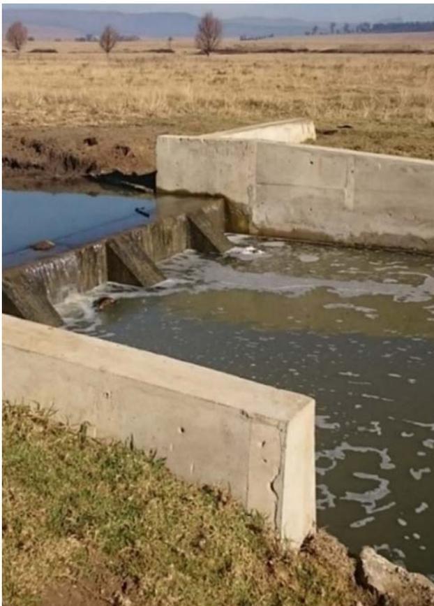
*Concrete butress weir built during phase 1 of Working for Wetlands construction cycle.*
