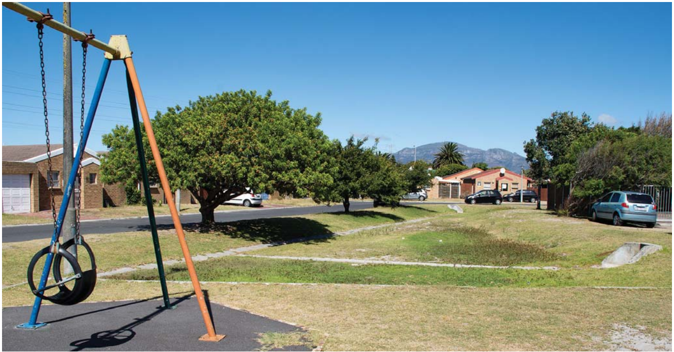
Most of the stormwater ponds in Cape Town are detention ponds that hold water for short periods during rainstorms but are dry for most of the year. Many are used as play-arks or informal sport grounds.
