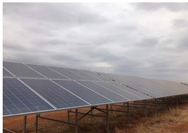
Some of the 768 solar panels at Becker Farm, which generate energy for a direct pump irrigation system.
