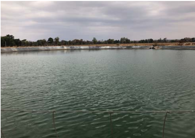
A storage dam on Becker Farm Limpopo supplies centre pivot irrigation to potatoes, onions, lucerne and pecan nuts.
