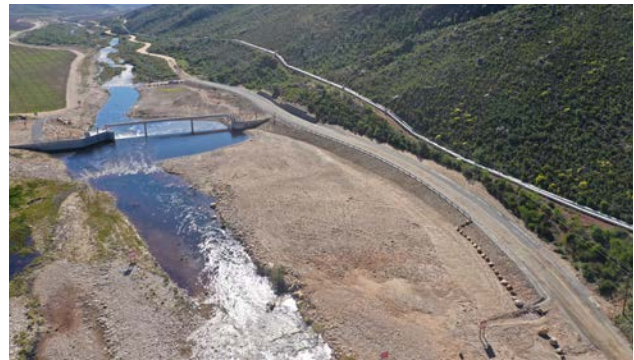
The Holsloot weir in July 2021, two months after the handover ceremony. At far right is the pipeline that conveys water from Stettynskloof Dam to Rawsonville and Worcester.
