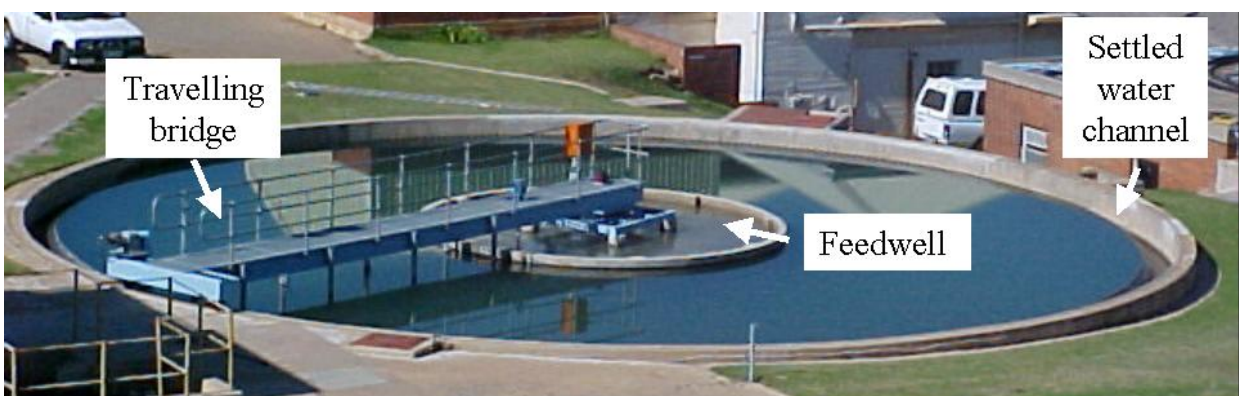
(c) Radial flow clarifier with travelling bridge.
