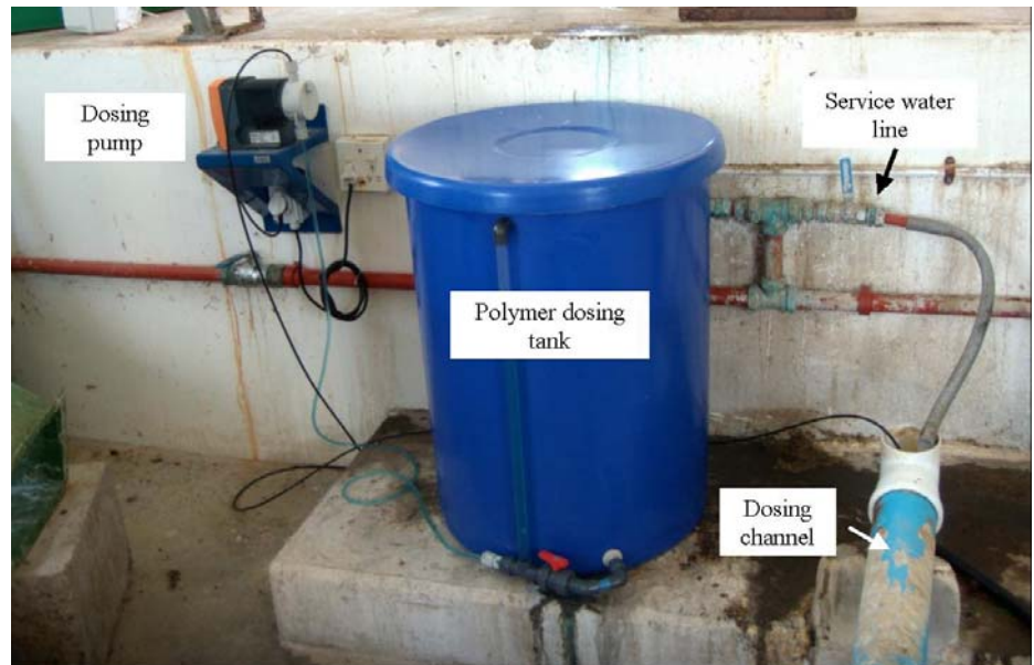
(b) Polymer dosing system with dosing pump.
