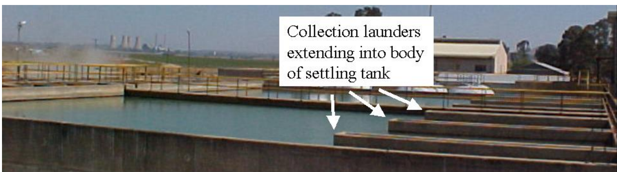
(b) Horizontal settling tank with collection launders extending into the main body of the tank
