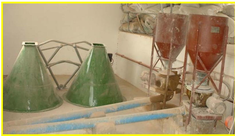
Fig. 2.1 Photo showing dry chemical feeders for alum and lime (from left to right, the green conical units lying on the floor were bought but never used because they were inappropriate ).
