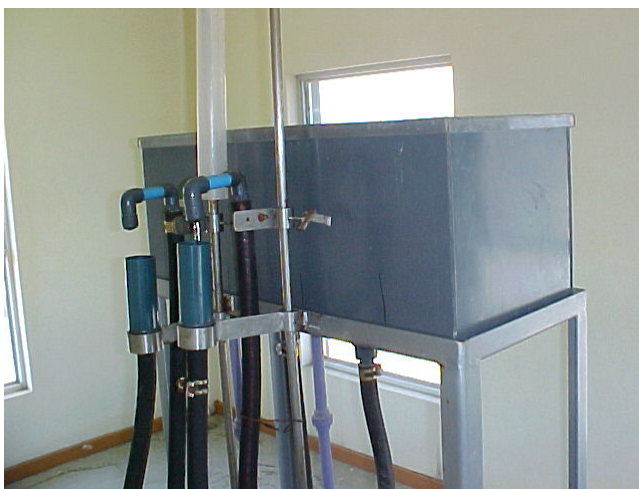
Fig. 4.5 Coagulant dosing systems
