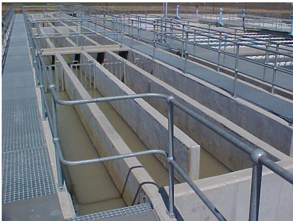
Fig.4.8 Flocculation channels
