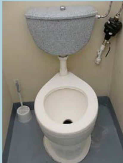
Low flush system installed in a school setting.
