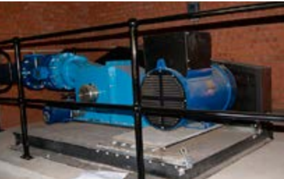
Crossflow turbine and generator installed for the Bloem Water project.
