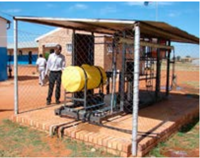
A nanofiltration plant provides clean water to the small village of Madibogo, in North West.
