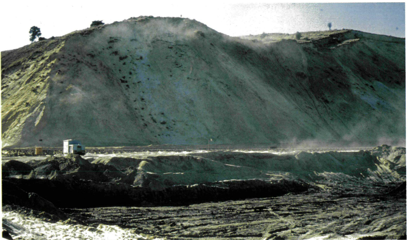
Soils contaminated with toxic substances can have a direct influence on human health if houses are built and gardens are established on land affected by mine tailings.
