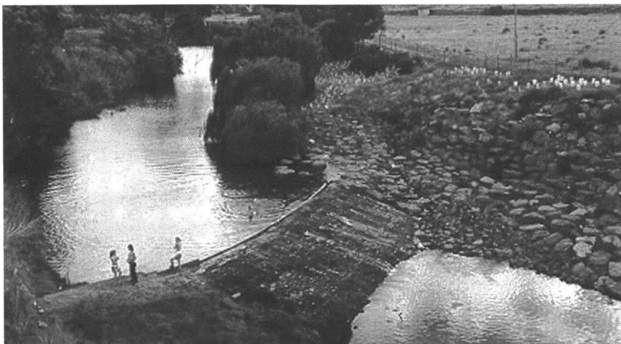
A weir on the Maribyrnong river, in Australia. A rock ramp fishway (on the right) was recently created to overcome the weir.
