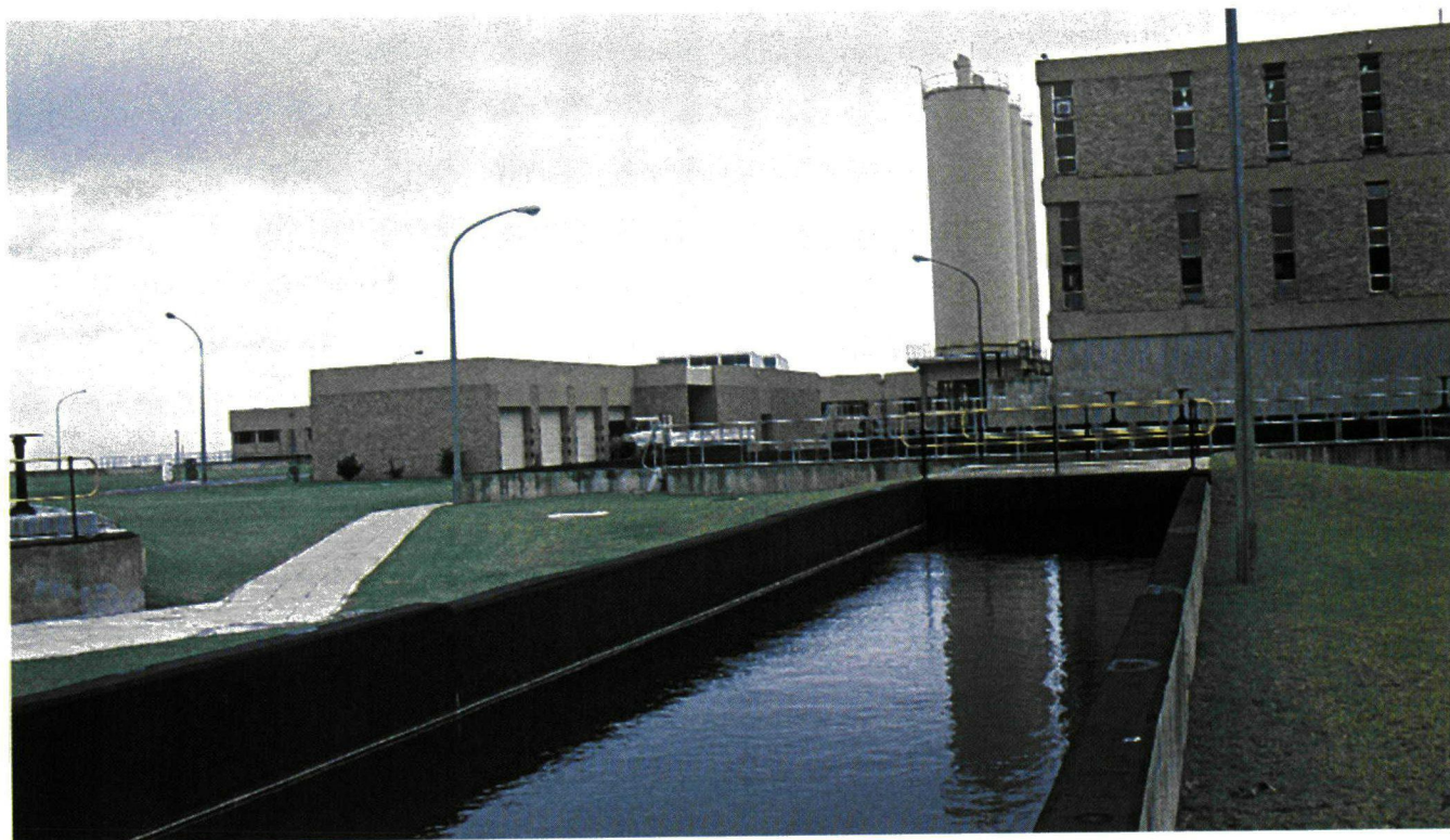
The Blackheath Water Treatment Works in the Western Cape.
