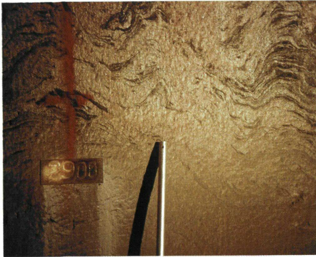
Banded Gneiss in the Emolweni tunnel
