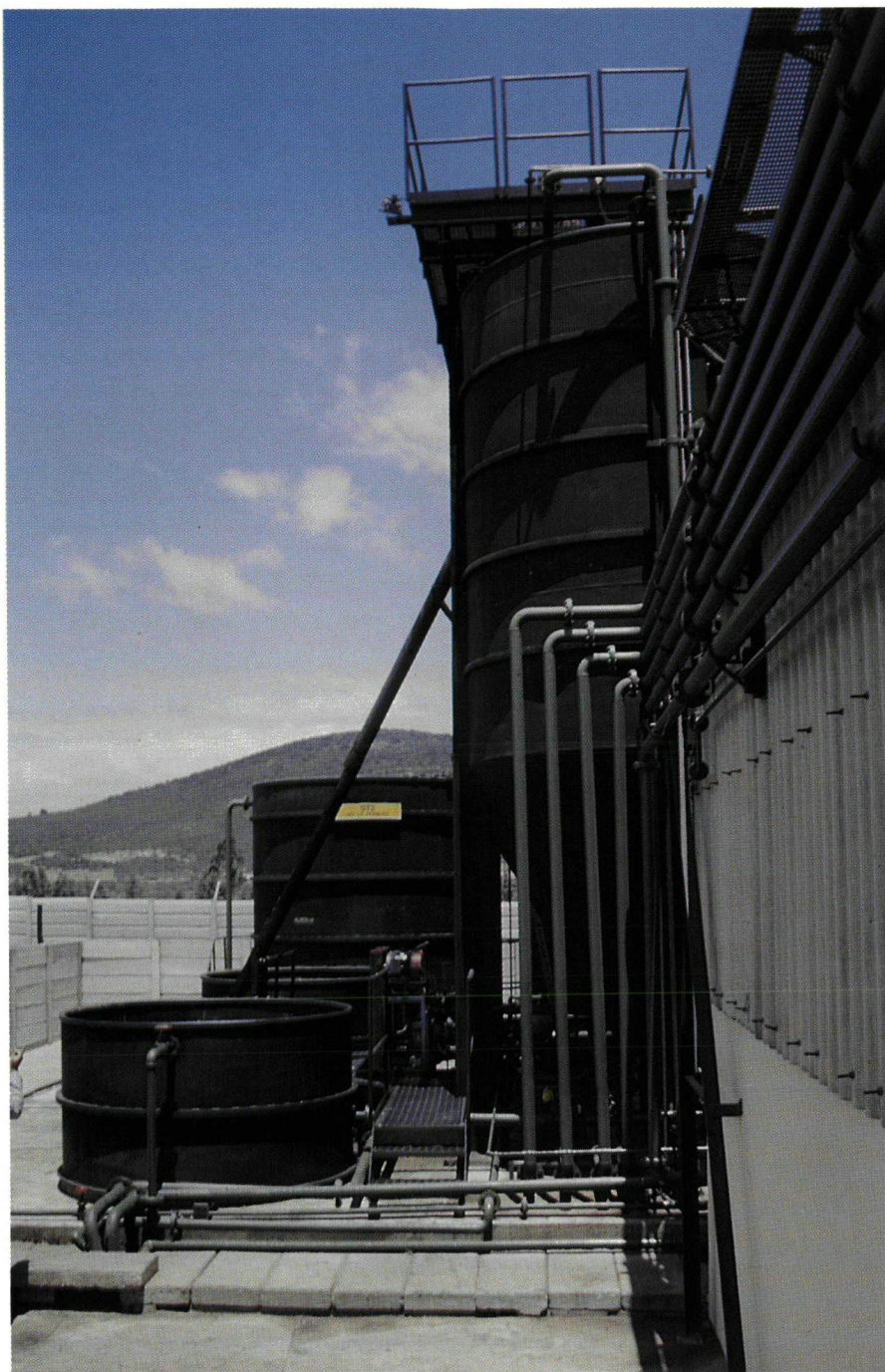
Part of the demonstration plant for the treatment of wool scouring effluent and rinse water at Gubb & Inngs in Uitenhage.
