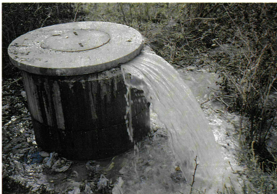
Surcharging sewers resulting from poor design, misuse and lack of maintenance may introduce large volumes of faecally contaminated effluent into the water environment with attendant health risks.
