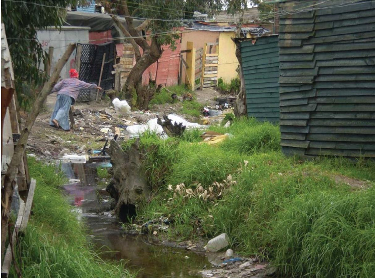
**Figure 3.2** An example of a drainage channel being used as a conduit for solid waste in Masiphumelele settlement, Cape Town
