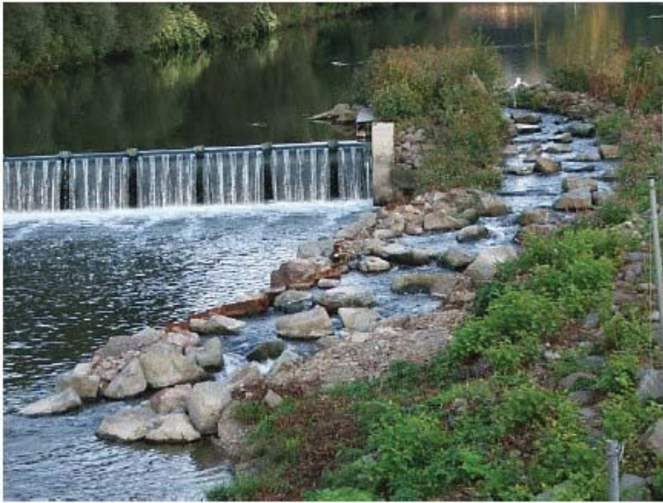
Figure 7.7 Rock-ramp bypass channel on a low weir in the Lenne River, Germany (from Bok et al. 2007).
