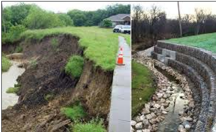
Figure 7.13 Bank stabilisation using the gabion-terrace approach. A lower slope angle and greater terrace width is advised.
