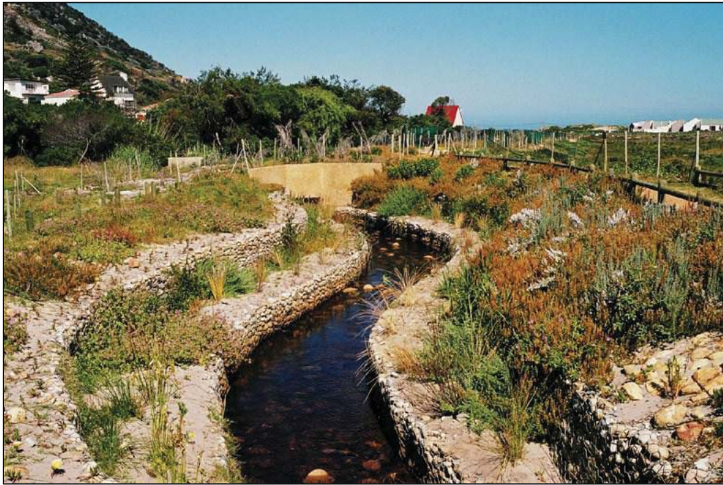
Figure 7.14 An example of cutting back and gabion-terracing the eroded right bank of the river, and armouring the bed with rock to create instream habitat. Constructed for flood management purposes at Silvermine Reserve (African Gabions Gallery)
