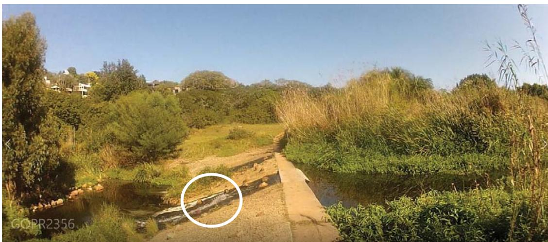
Figure 5.5 The large weir at Dodd's farm, upstream of the sample site. At the time of sampling raw sewage was discharging from a pipe on the downstream wall (circled).
