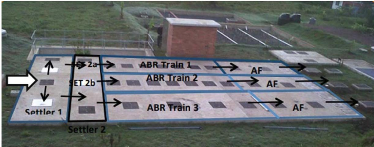
**Figure 2.2: The Decentralised Wastewater Treatment System (DEWATS) constructed at Newlands Mashu, Durban, South Africa (ABR: anaerobic baffled reactor; AF: anaerobic filter; SET: settler).**
