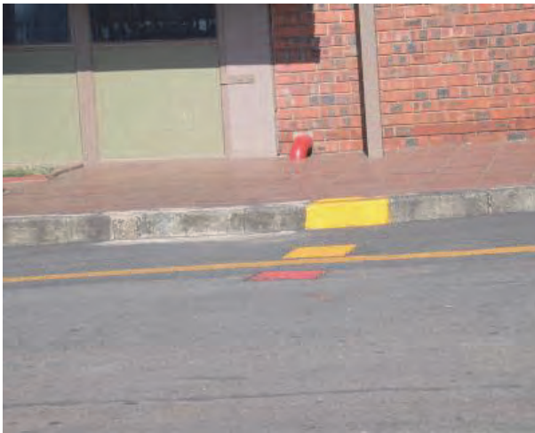
Figure 124: Example of an Un-metered fire connection
