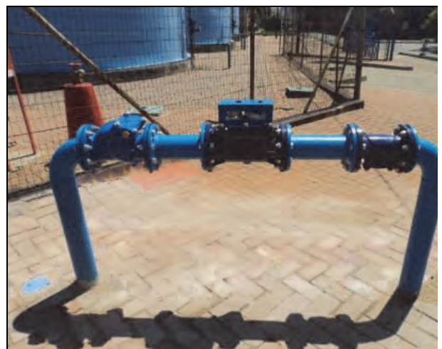
Figure 135: Complete meter installation
