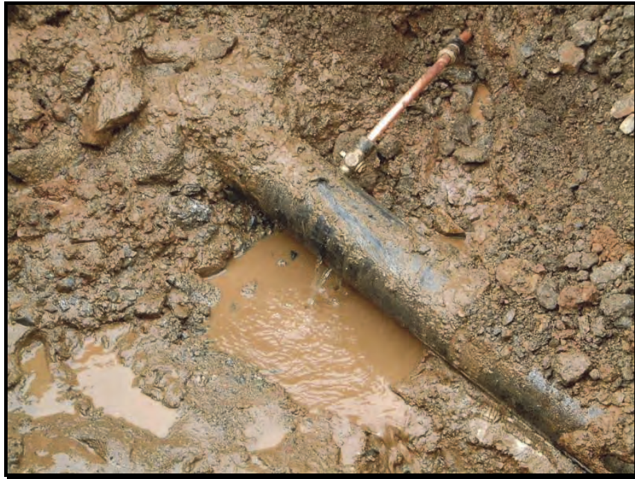
Figure 10: Underground leak running at low pressure (Ken Brothers)
