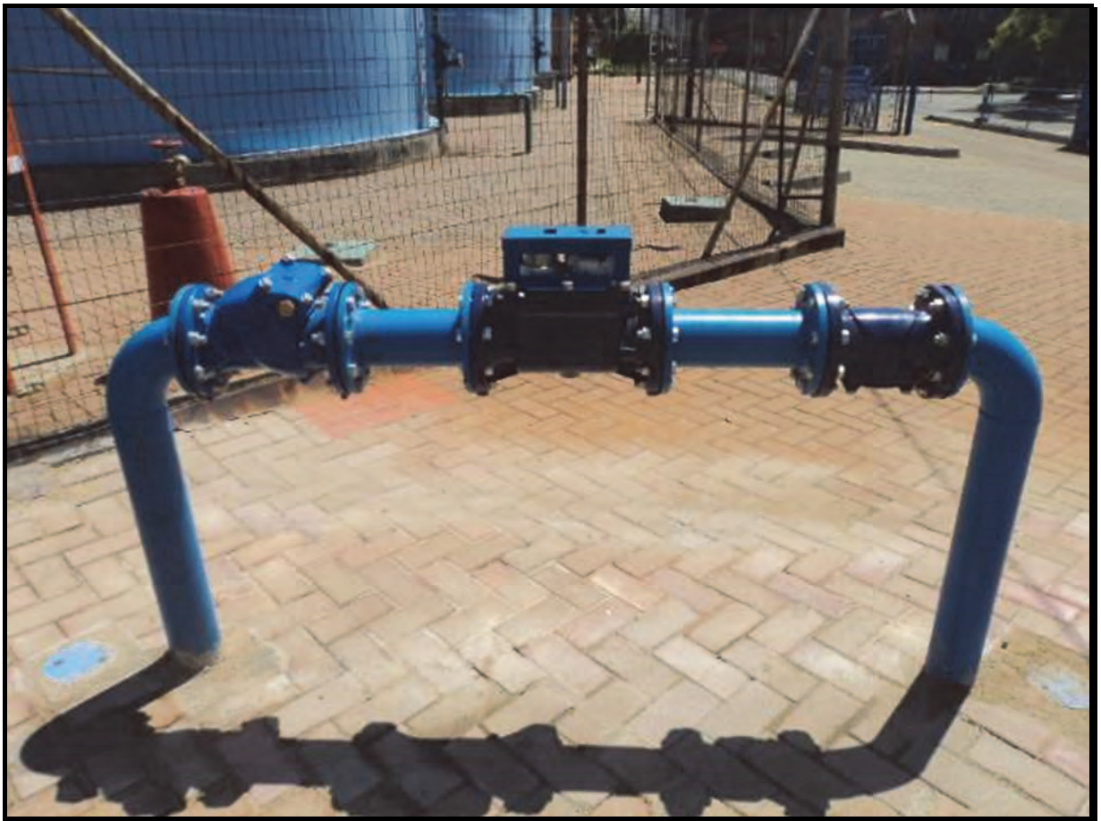
Figure 16: Typical bulk industrial meter in Ekurhuleni
