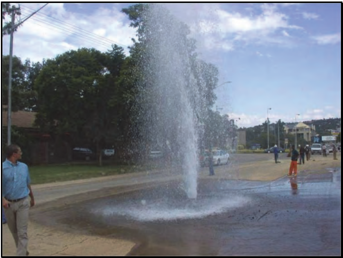
Figure 25: Typical mains burst
