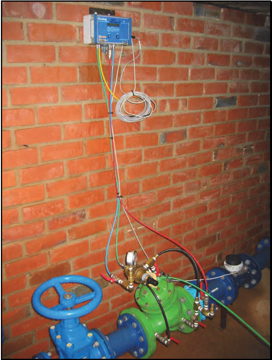
Figure 89: Typical PRV with time-control (photo Niel Meyer)
