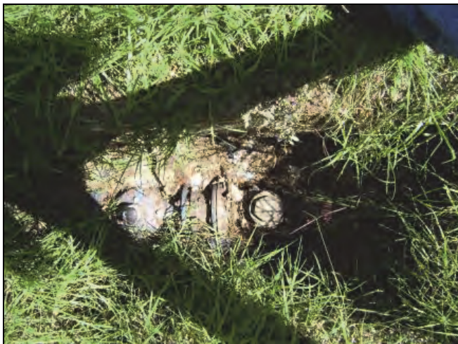
Figure 122: Meter buried in ground
