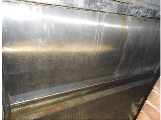
Figure 160: leaking urinal in school
