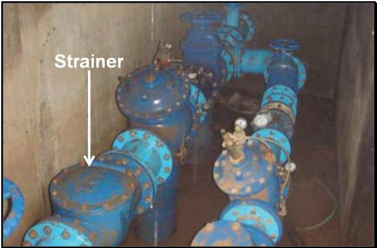
Figure 41: Typical strainer before a PRV
