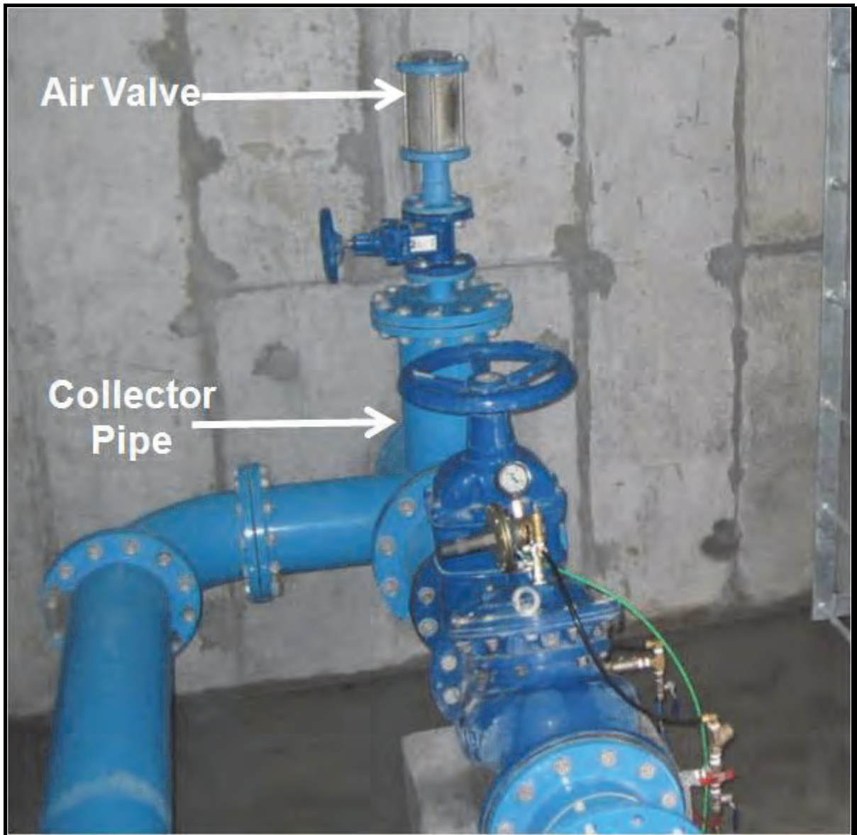
Figure 45: Typical air-valve and collector pipe
