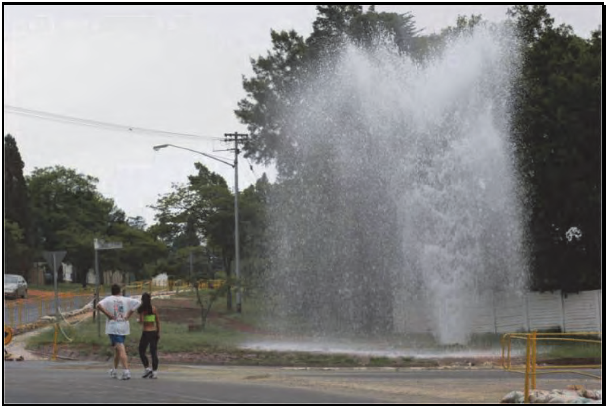
Figure 57: Mains leak on 315mm-diameter uPVC pipe at \pm 50\text{m} pressure
