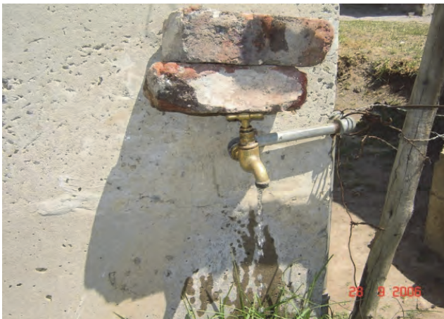
Figure 157: Leaking tap in school
