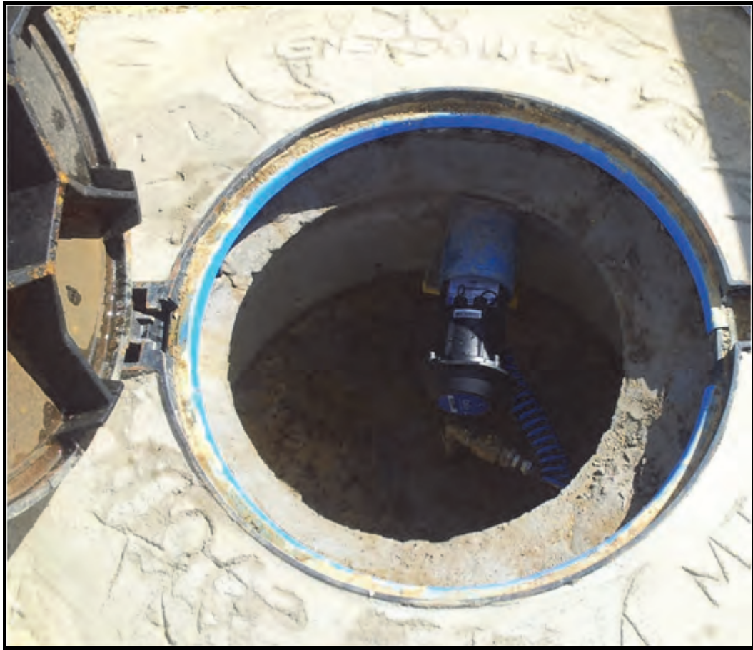
Figure 139: Typical pressure logging point in Drakenstein (Courtesy A Kowalewski)
