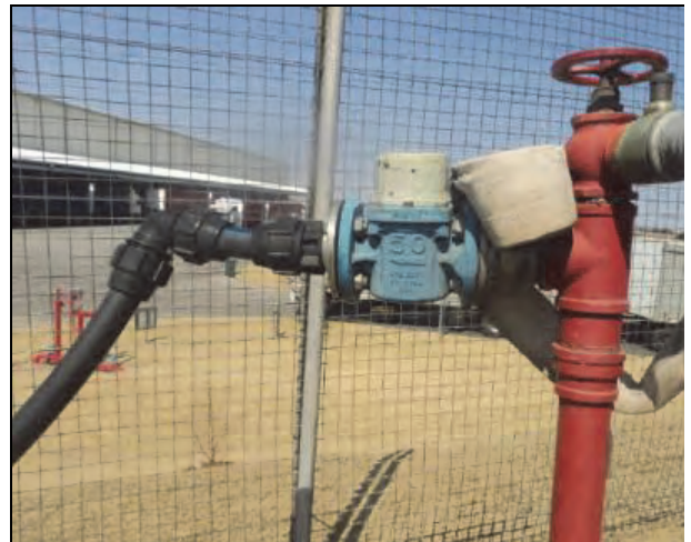
Figure 125: Example of illegal connection to un-metred fire supply by consumer
