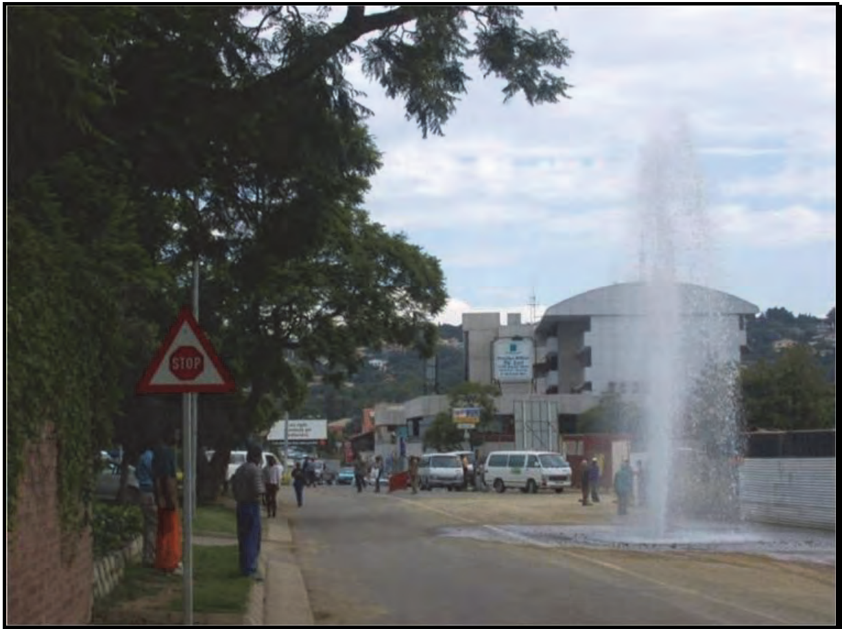
Figure 56: Leak on 110mm-diameter uPVC main at \pm 60\text{m} pressure
