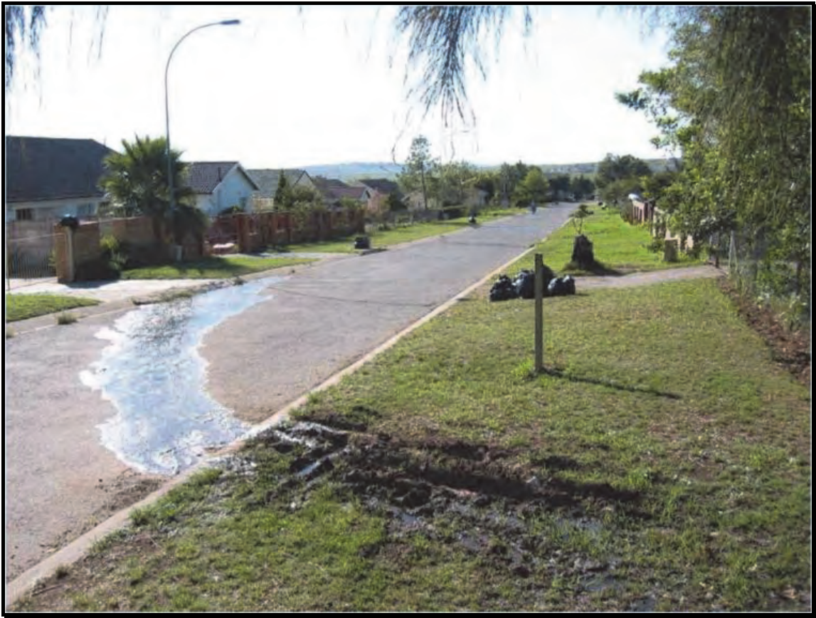
Figure 27: Typical connection leak before the meter
