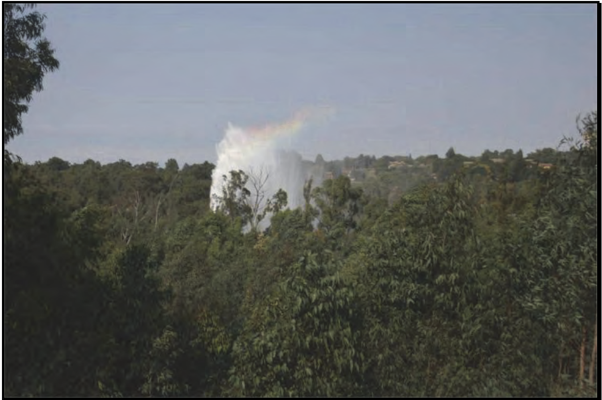
Figure 54: Large mains leak on 600mm-diameter main at 260m pressure
