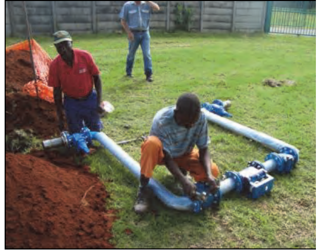
Figure 131: Preparing meter pipework
