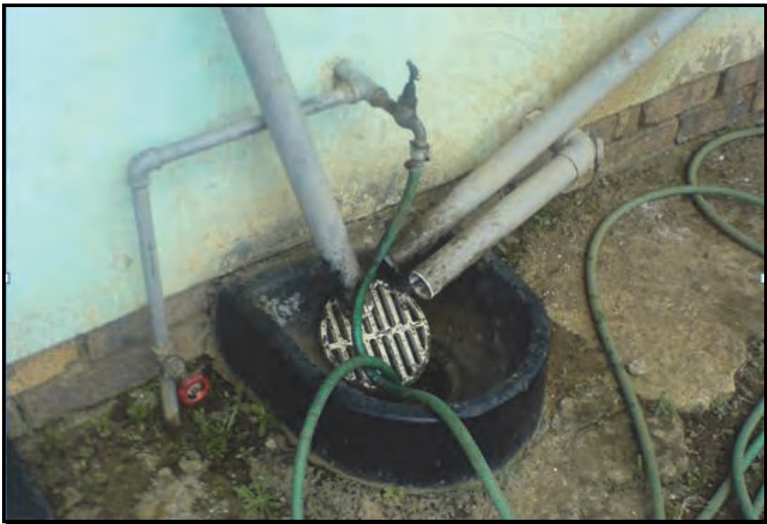
Figure 172: Leaking tap "repair" at one property (courtesy Zama Siqalaba)
