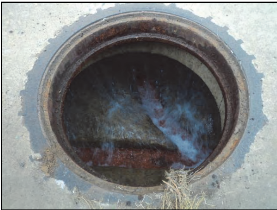
Figure 62: Leak on 63mm uPVC pipe flowing into stormwater manhole
