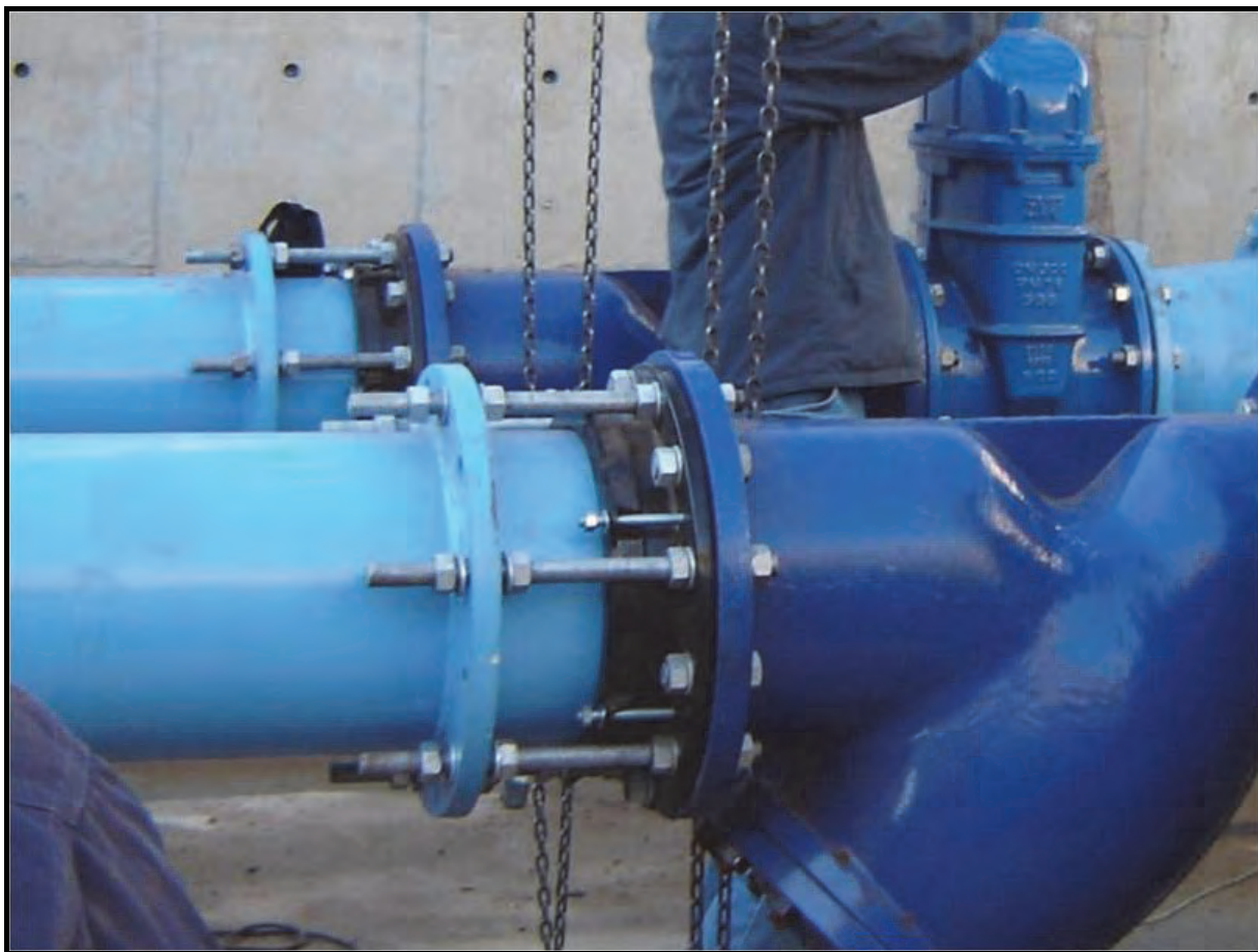
Figure 52: Flange adaptor with restrained dismantling joint (bolts not tightened)
