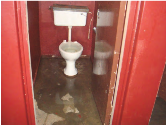
Figure 155: Leaking toilet in school
