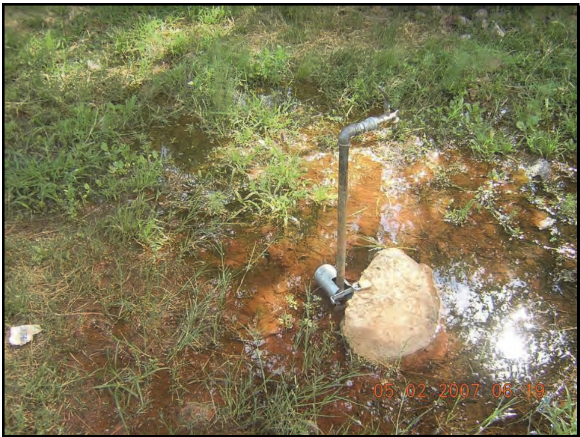
Figure 28: Property leak after the meter (Courtesy Niel Meyer)
