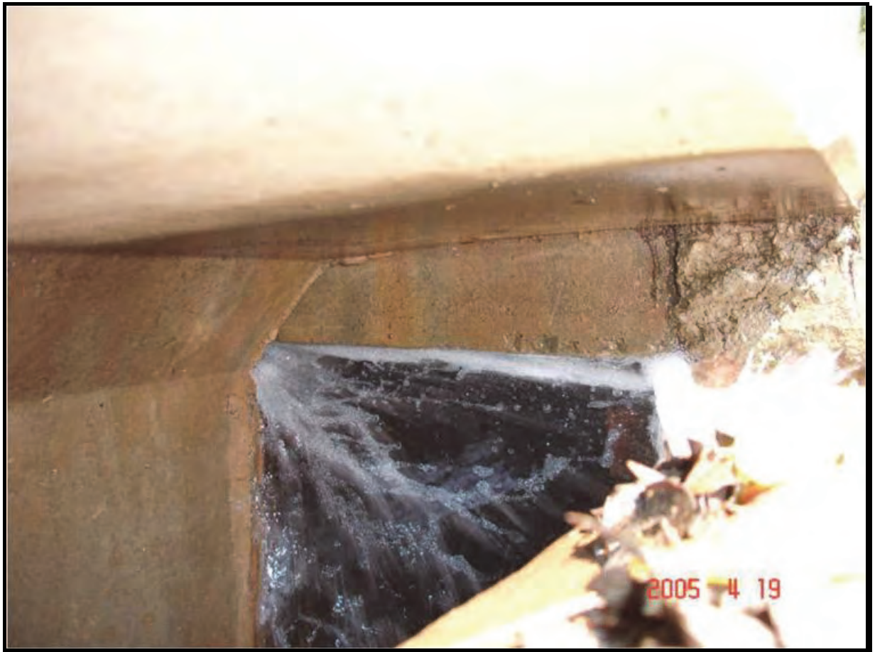
Figure 59: Hidden connection pipe burst on 25mm uPVC pipe at \pm 60\text{m} pressure
