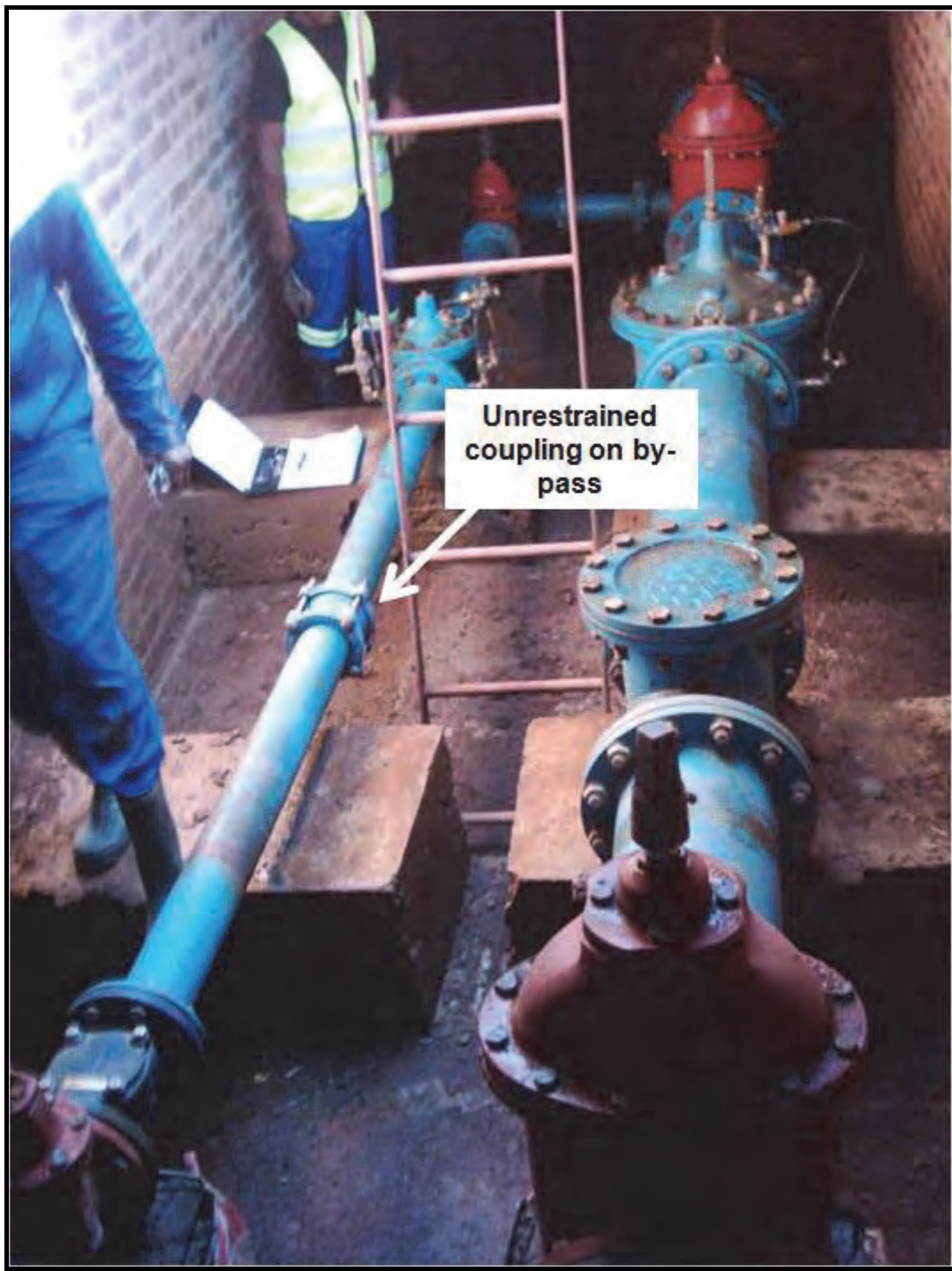
Figure 53: installation with unrestrained coupling on by-pass
