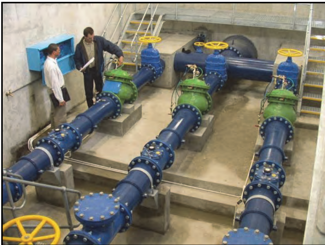
Figure 107: Khayelitsha pressure management installation
