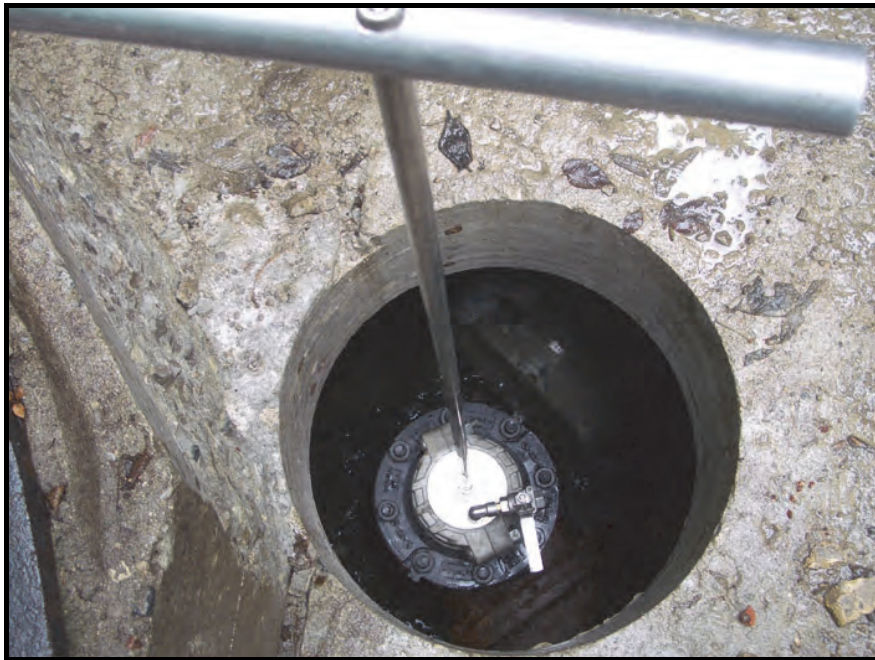
Figure 78: Smart Ball insertion equipment (courtesy S Hamilton)
