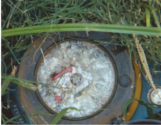
Figure 161: Leaking school meter
