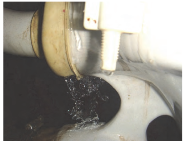
Figure 158: Leaking toilet fitting in school
