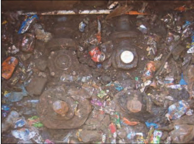
Figure 120: Buried and broken meters
