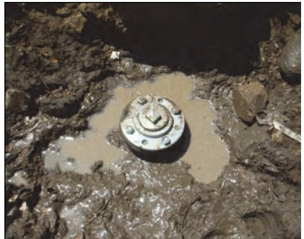
Figure 133: Capping of old connection
