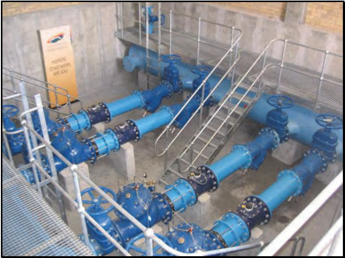
Figure 115: Mitchells Plain pressure management installation
