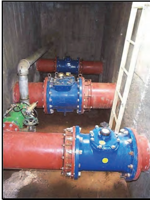
Figure 15: Some bulk meters in Johannesburg
