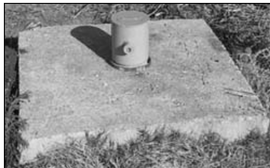
Figure 4.6. Borehole construction must prevent local surface contamination entering the aquifer.
