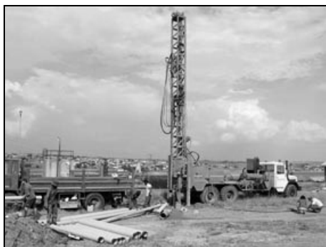
Figure 4.6. Borehole construction must prevent local surface contamination entering the aquifer.
