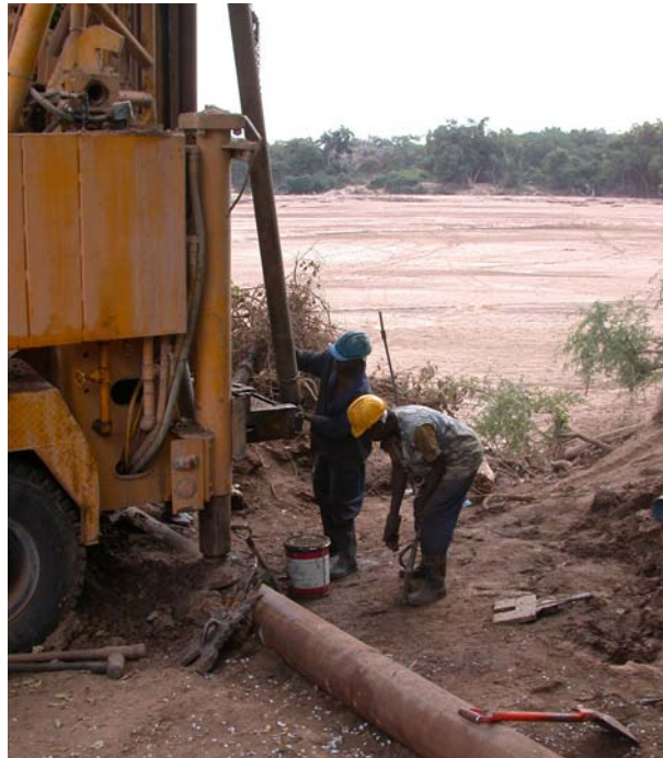
Figure 3.7: Drilling water supply boreholes on the banks of the seasonal Limpopo river. The view looks north from the South African bank to the riparian vegetation on the Zimbabwean bank in this trans-boundary ADE.
