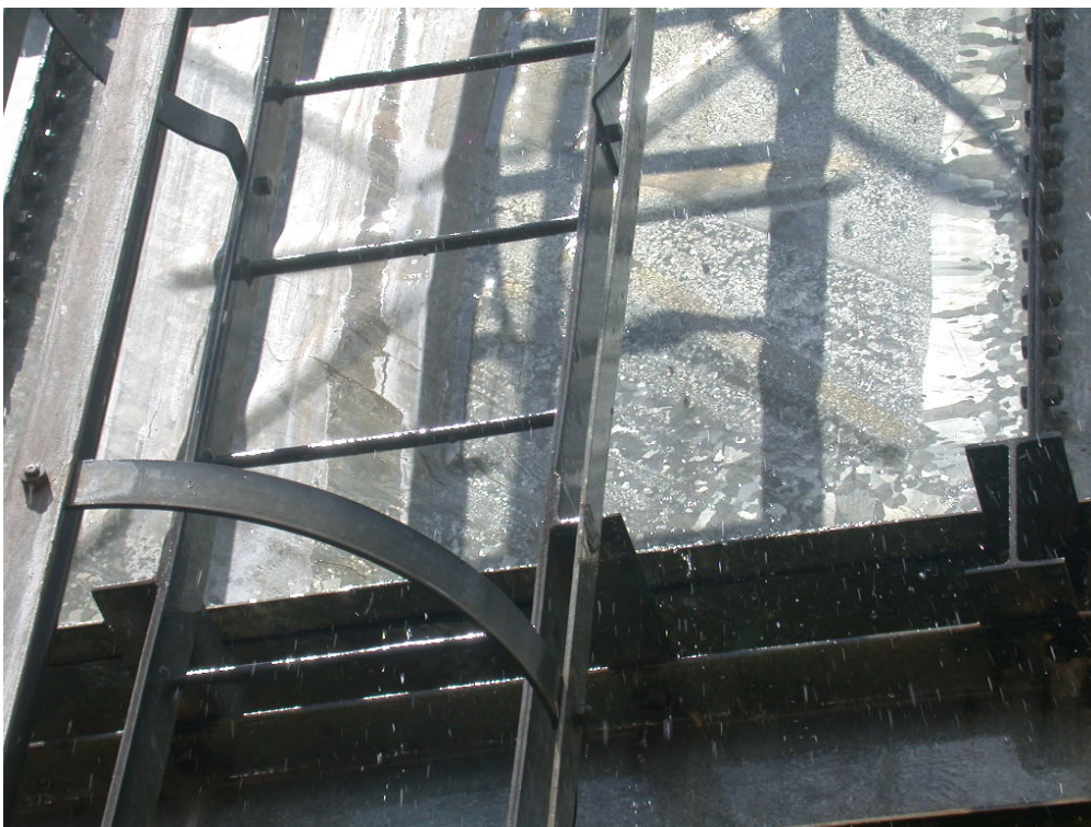
Figure 31: Overflow at a steel reservoir structure
