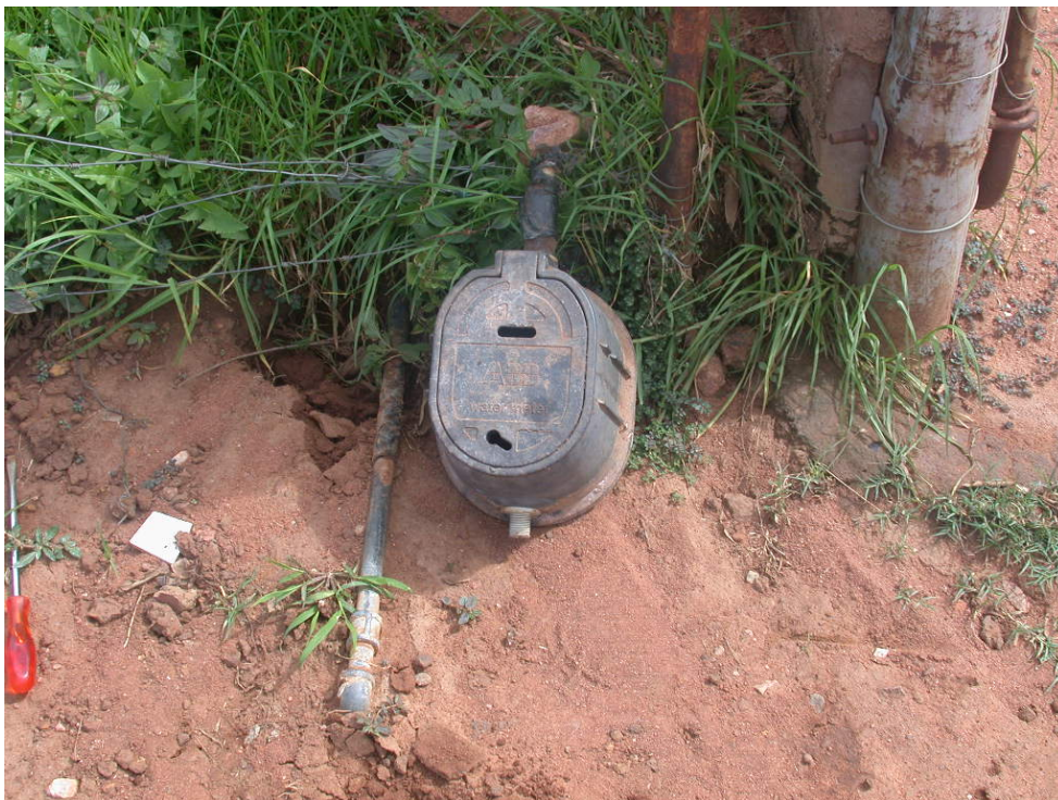
Figure 28: An illegal connection where a consumer meter has been bypassed
