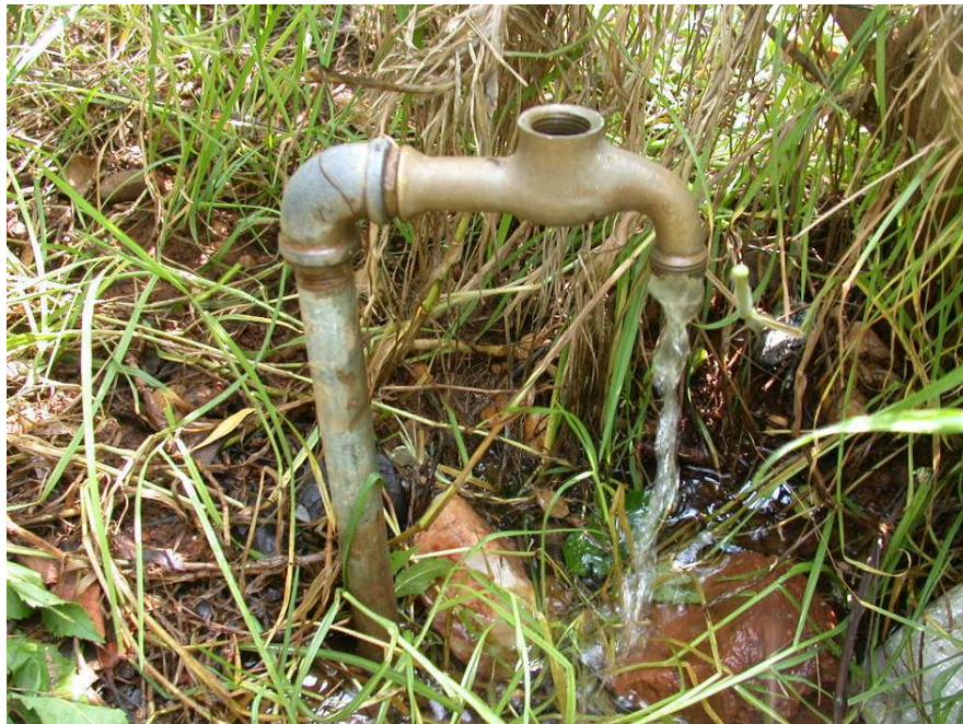
Figure 26: Standpipe left running after spindle was removed
