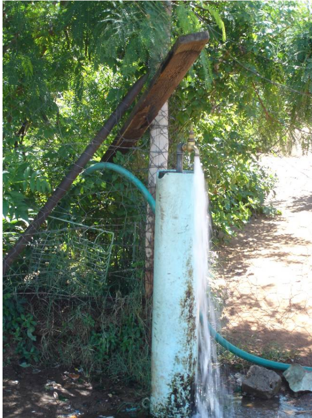
Figure 27: Pressure at a standpipe which can not be turned off
