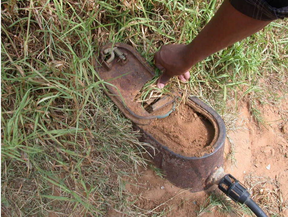
Figure 23: A customer meter which can not be read
