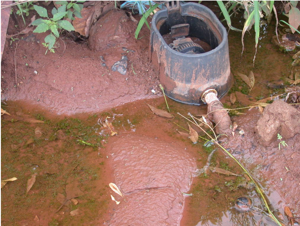
Figure 32: A leak at a service connection
