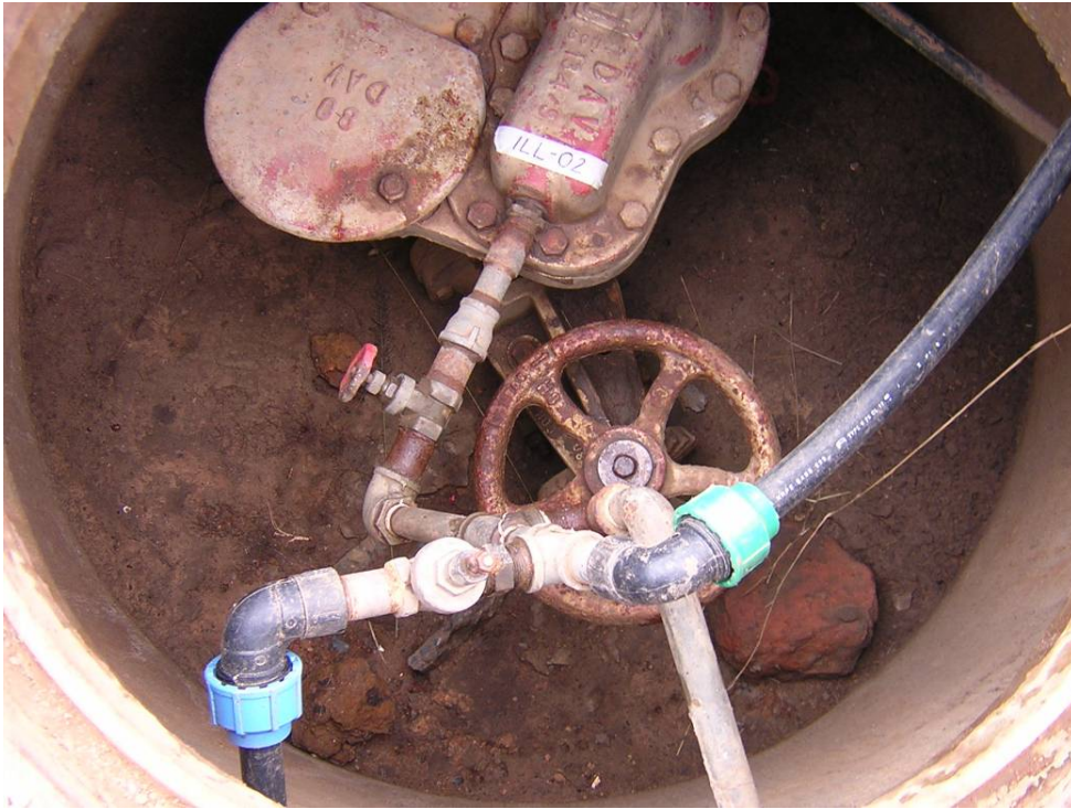
Figure 29: An illegal connection on an air valve
