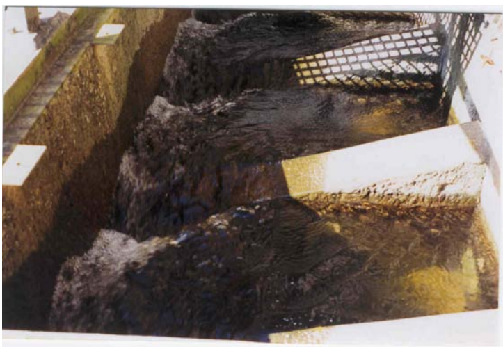
Plate 6-26 : Haga-Haga River Pool and Sloping Weir fishway designed for small (<120 mm long) fish.
