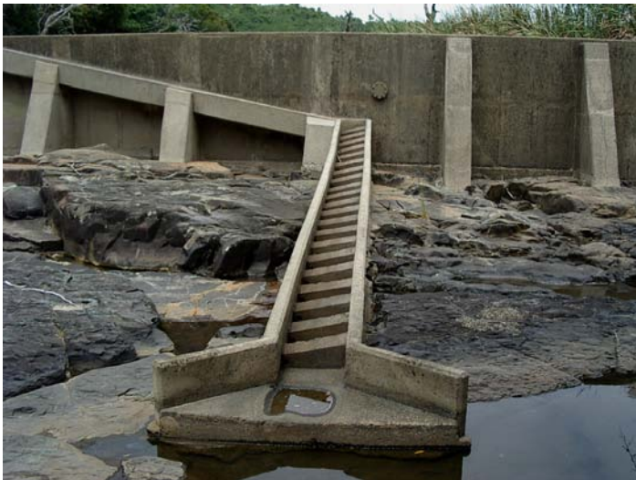
Plate 6-25 – Pool and slot fishway on Crocodile River.
