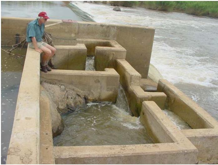
Plate 6-27 Close-up of sloping weir of the Nhlabane Pool and Weir fishway at low flows, looking up-stream. Note the wetted splash zone on sloping baffle at the edge of the main flow.
