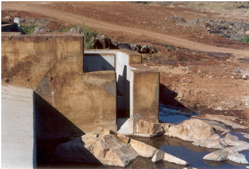
Plate 6-31 View of most down-stream slot of the "Pool and Slot" Ten Bosch fishway on the Crocodile River KNP, during low stream-flow conditions.
