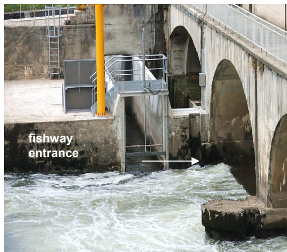
Plate 6-4 The fishway entrance at Mauzak, France, is situated adjacent and at 90 degrees to one of the outflows from the power station.
