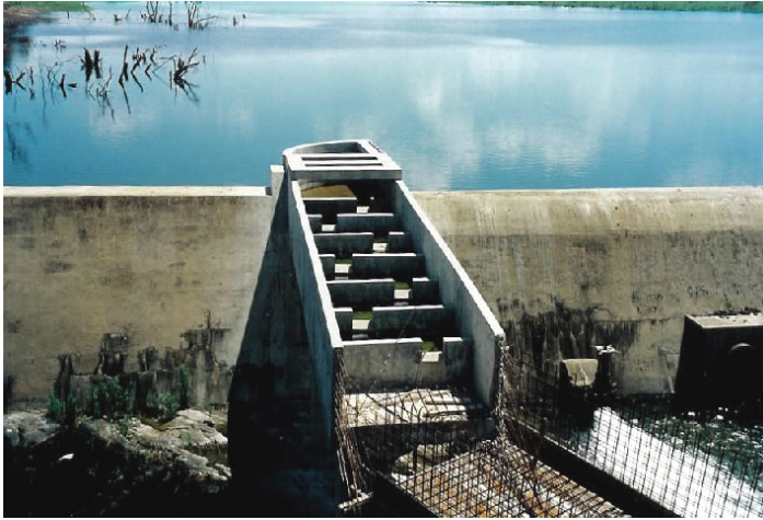
Plate 6-24 – Pool and notched-weir fishway on the Lebombo gauging weir on the Komati River.
