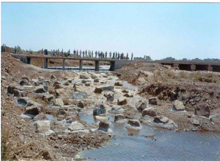
Plate 6-12 Bypass Rockramp fishway on the Lower Sabie River in KNP under low-flow conditions at commissioning in October 2001 showing placement of rocks.
