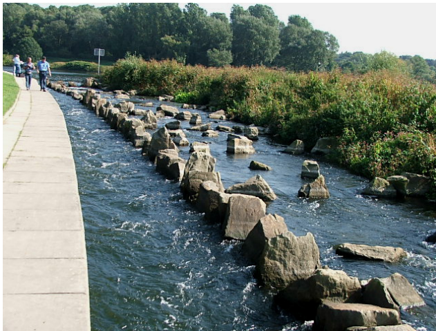
Plate 6-17 A fishway bypass channel (2) combined with a canoe pass (1) at Hattinghe in Germany. In practice fish use both channels, with larger, stronger-swimming fish using the canoe pass. Fish can move freely between rocks separating the two channels.
