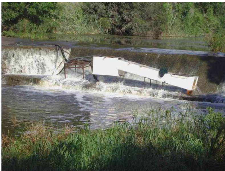
Plate 9-3: Fishway set up on the lower shelf at the base of the Kowie River weir.
