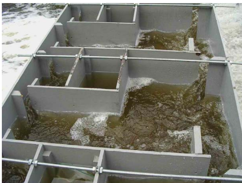
Plate 9-5: Fishway channel at high flow (18.9 l/s)
