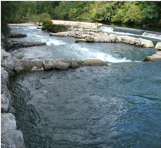
Plate 6-20 Typical vertical slot fishway in France, at the Barrage de Chatellerault.
