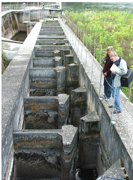
Plate 6-21 Large vertical slot fishway at Mauzak, France
