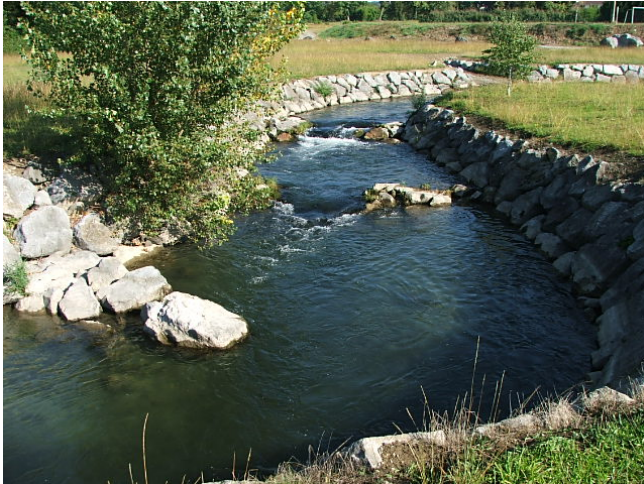
Plate 6-16 Gently sloping bypass channel at Meillon, France
