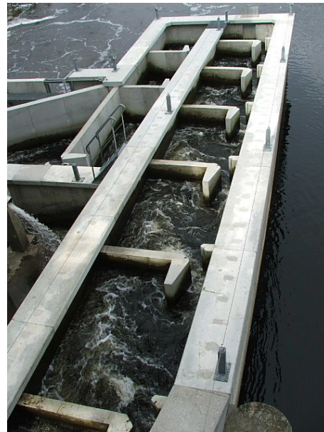
Plate 6-20 Typical vertical slot fishway in France, at the Barrage de Chatellerault.
