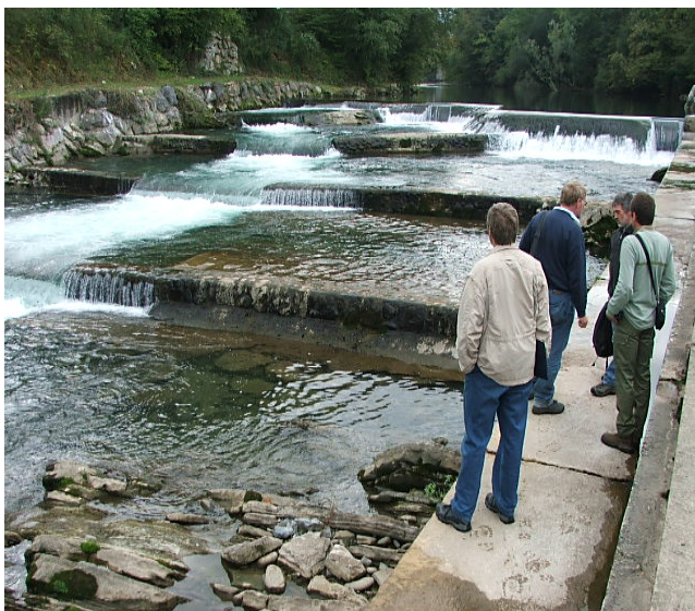
Plate 6-18 A series of pre-barrage walls below a weir at Gava de Oron, France.
