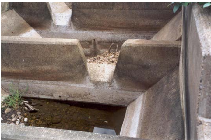
Plate 6-29 Close-up view of weir notch in the Kanniedood fishway, KNP during low-flow conditions with no water flowing down the fishway.
