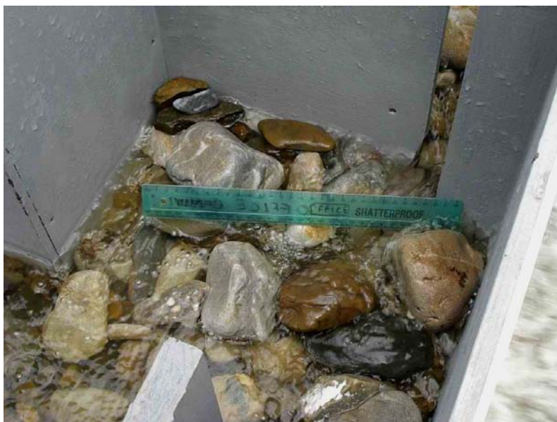
Plate 9-4: Fishway channel showing stones on bottom at low flows (large fishway channel).
