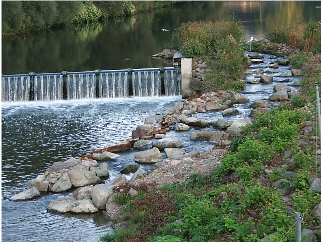
Plate 6-13 Bypass channel on the Lenne River fishway, Germany
