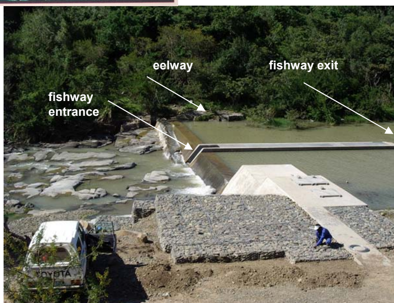
Plate 6-6 Fishway on the Nqabara River (Transkei). The entrance is at the base of the weir and the channel extends upstream, with the exit away from the spillway. Note the eelway/prawnway with entrance next to the fishway entrance, thus providing additional attraction water.
