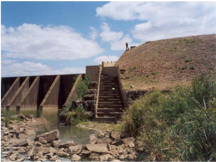
Plate 6-30 Close-up of "Pool and Slot" baffle at Riverside Weir Fishway in the KNP under low flow conditions.
