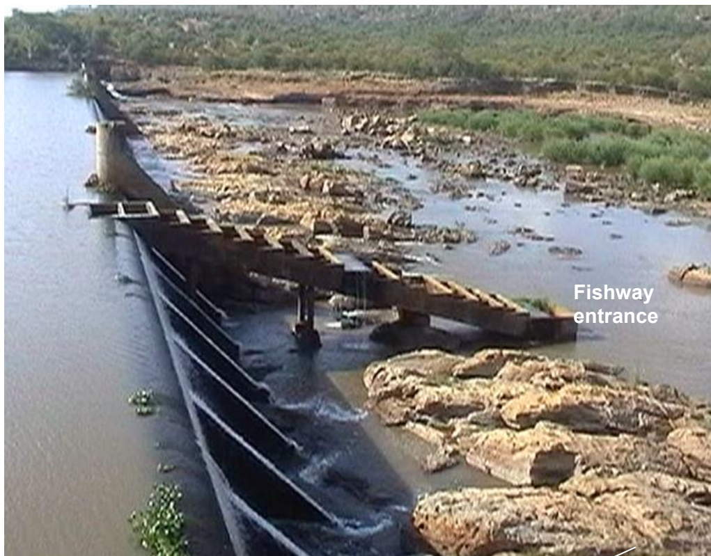
Plate 6-1 The Engelhardt Dam fish ladder on the 13 m high Letaba Dam, Kruger National Park, built in 1970. The entrance to the fishway is located too far downstream of the barrier to be easily found by upstream migrating fish. The submerged fishway exit is located near the crest of the weir, allowing tired fish leaving the fishway to be swept downstream.
