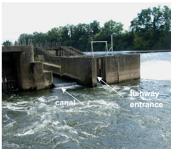
Plate 6-3 This fishway at Bergerac, France, has its entrance at the foot of the weir, and which also receives attraction water through an adjacent canal.
