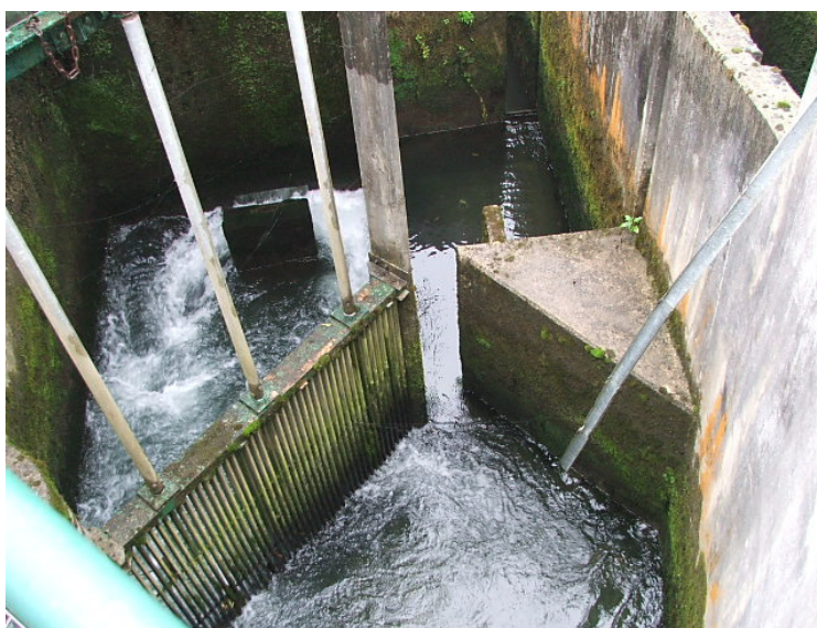
Plate 6-7 View of up-stream section of the Nhlabane Fishway showing the series of manually-operated sluices for letting water into the fishway and providing an exit for fish leaving the fishway.
