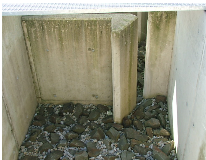
Plate 6-22 Rocky stratum on the bottom of a vertical slot fishway pool at the Raffelberg II fishway in Germany.
