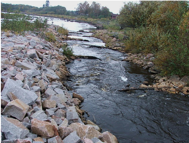
Plate 6-14 Bypass channel on the Siika Joki - White Fish River, Finland
