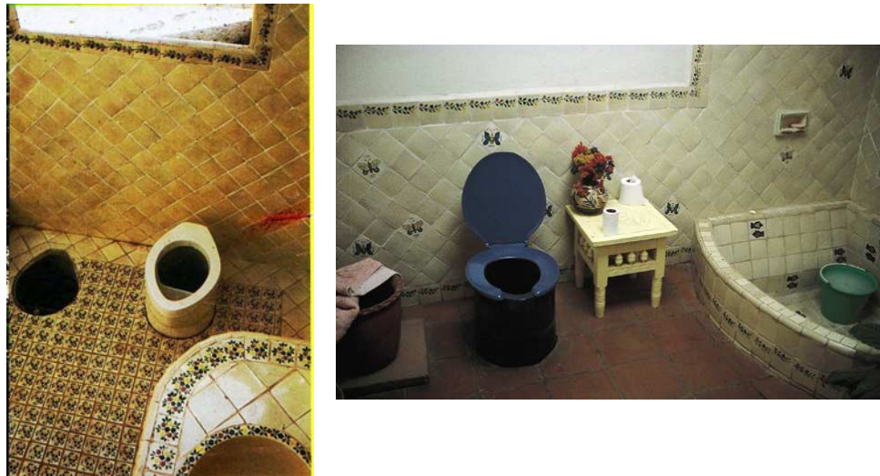
Figure 2.5: The Mexican version of the Vietnamese double-vault toilet, installed in the bathrooms of modern houses in the city of Cuernavaca. The toilets have movable urine-diversion pedestals. The processing chambers below the bathroom floor are accessible from outside the house (César Añorve, CITA, A.C., Mexico)
