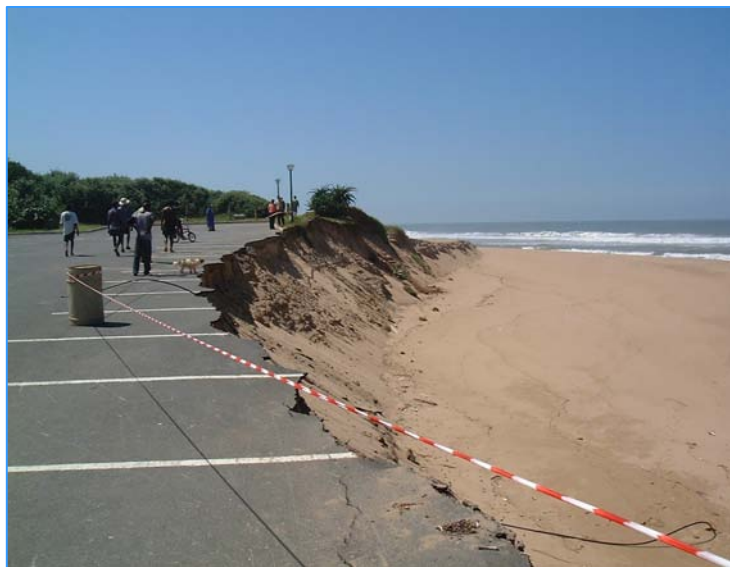
The consequences of attempting to stabilize sand at an estuary mouth – Mdloti Estuary (Ken Breetzke)
