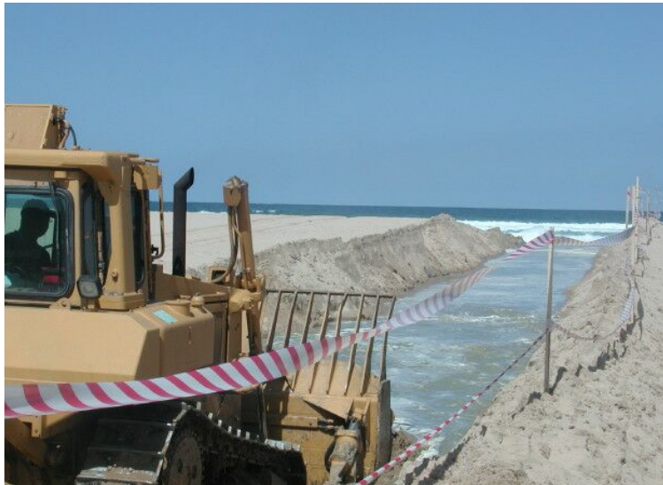
Artificial breaching of an estuary mouth (Piet Huizinga)
