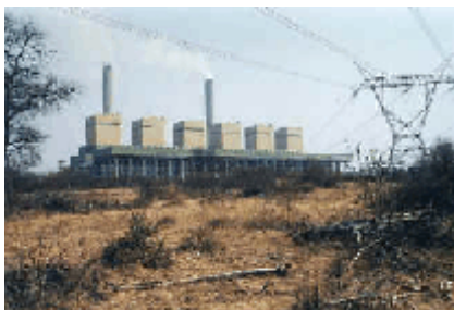
FIGURE 5 : The Matimba and Kendal Power Stations using the direct and indirect dry-cooled technology respectively.
