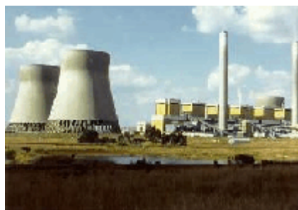
FIGURE 5 : The Matimba and Kendal Power Stations using the direct and indirect dry-cooled technology respectively.
