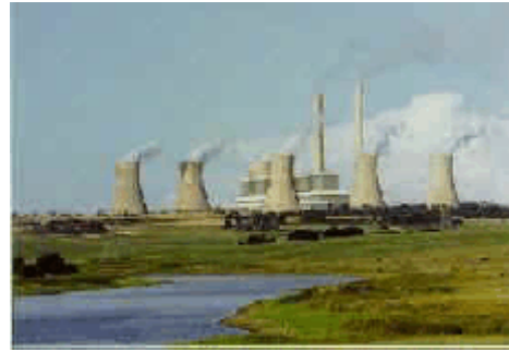
FIGURE 4 : Wet cooling towers at the Lethabo and Duvha Power Stations
