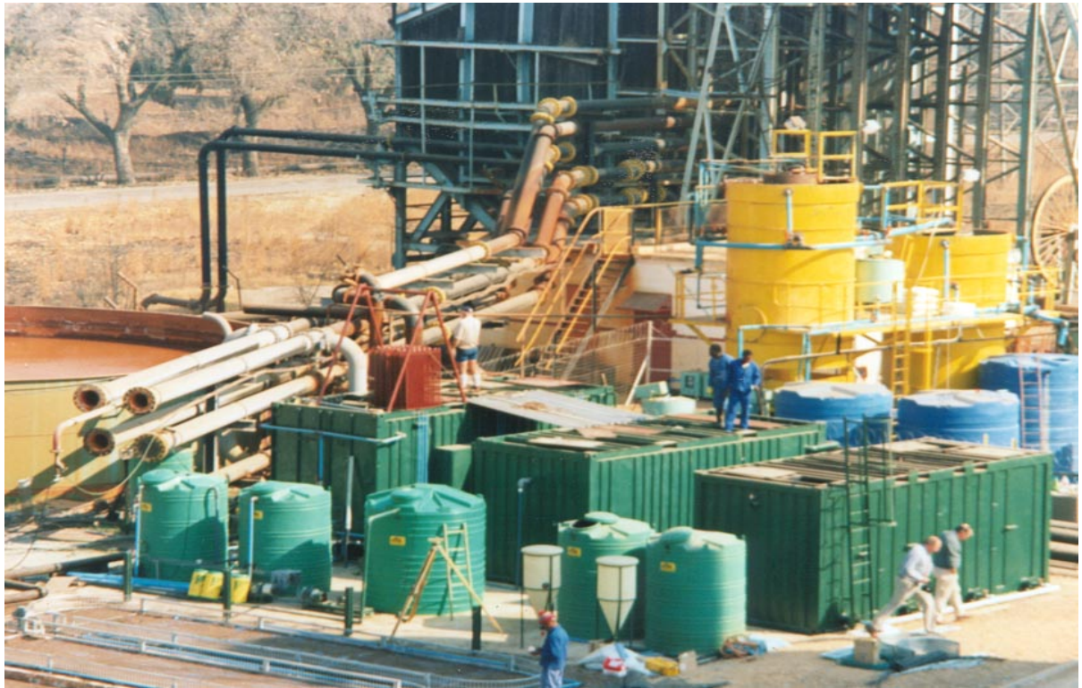
Figure 1.3 The Rhodes BioSURE Process Pilot plant located at Grootlvei Gold Mine No 3 Shaft in Springs.
