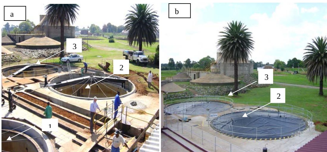
Figure 4.4 Photograph of the Dortmund tanks that were converted into components of the Technical-scale Multi-stage Reactor constructed at Ancor Works, Springs (a) reactor under construction (b) completed reactor sealed to minimise escape of sulphide and to maintain anaerobic conditions. 1= Dortmund-type Upflow Recycling Sludge Bed Reactor (RSBRd); 2= Continuous Stirred Tank Reactor (STR); 3= Clarifier.
