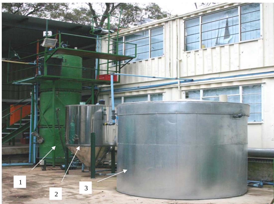
Figure 4.2 Photograph of the Pilot-scale Multi-stage Reactor at Environmental Biotechnology Research Unit (EBRU), Grahamstown South Africa. 1= Column Upflow Recycling Sludge Bed Reactor (RSBRc); 2= Continuous Stirred Tank Reactor (STR); 3= Clarifier.
