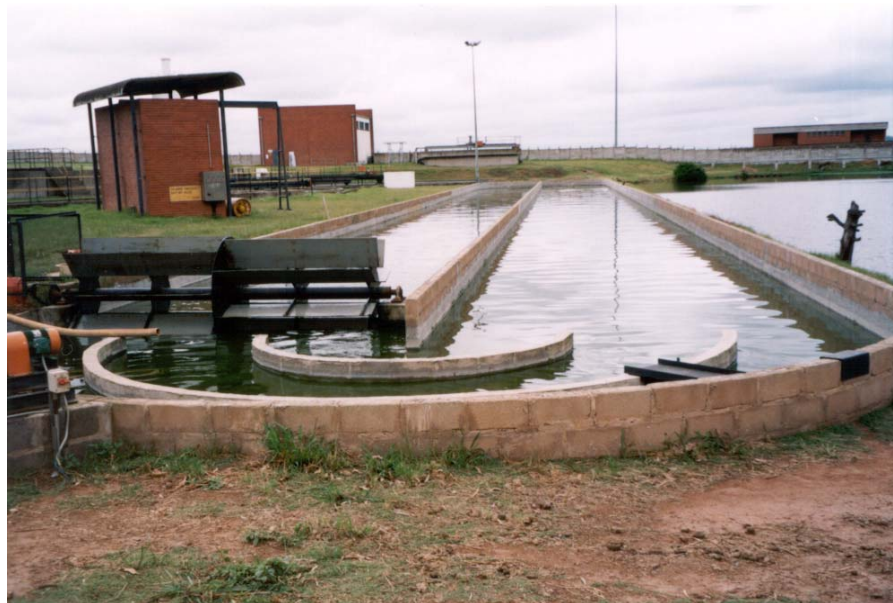
Figure 1. The HRAP unit operation of the IAPS pilot plant constructed at the Cato Ridge Abattoir.
