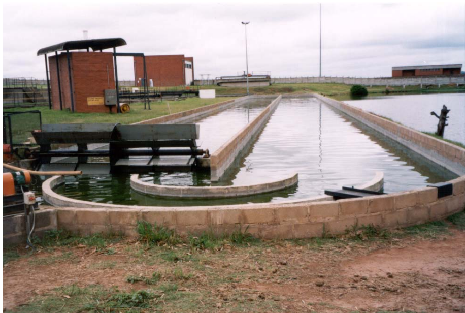
Figure 4.2 The High Rate Algal Pond unit operation of the IAPS pilot plant constructed at the Cato Ridge Abattoir.
