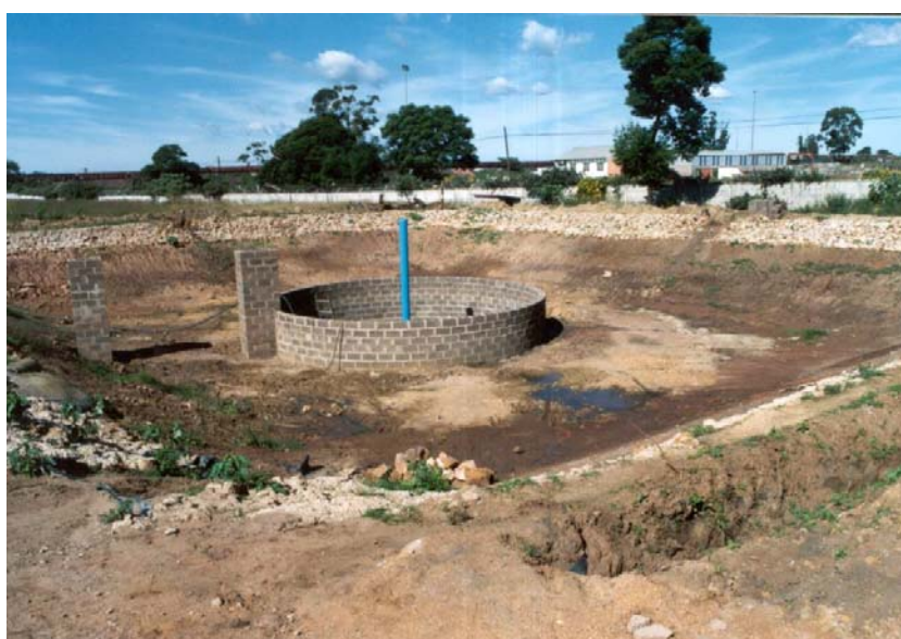
Figure 4.1 The Fermentation Pit and Facultative Pond of the IAPS abattoir wastewater treatment plant was constructed in a pre-existing balancing dam available on-site at the Cato Ridge Abattoir.
