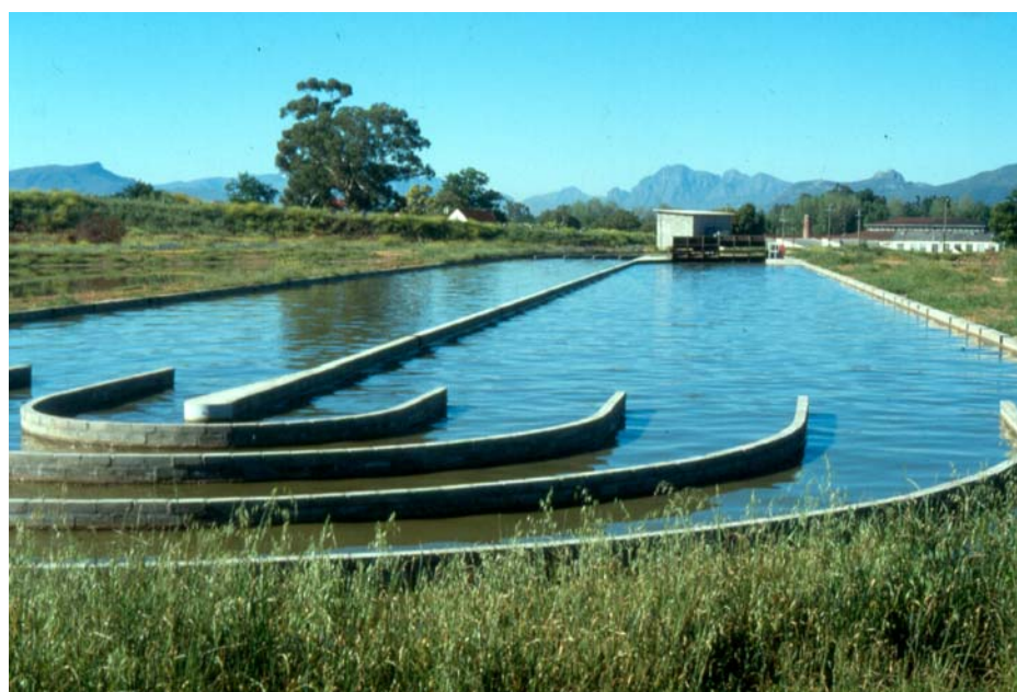
Figure A9.1 The 2 500 m 2 Spirulina -HRAP (S-HRAP) raceway, a component unit operation in the IAPS system treating tannery effluent at the Mossop Western Leathers Co., Wellington.
