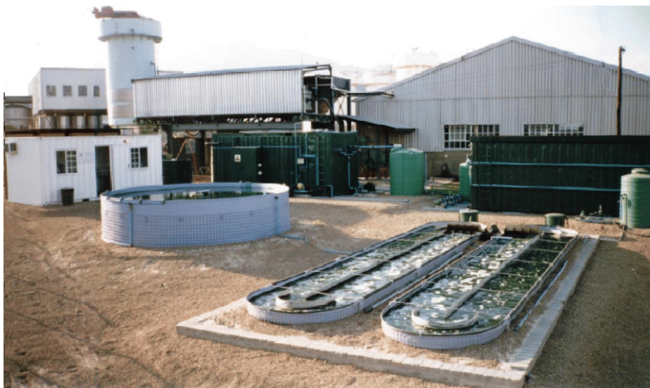
Figure A 9.5. Pilot plant at Brennoken Co., in Worcester, South Africa, evaluating the IAPS in the treatment of wine lees and distillery wastewaters.
