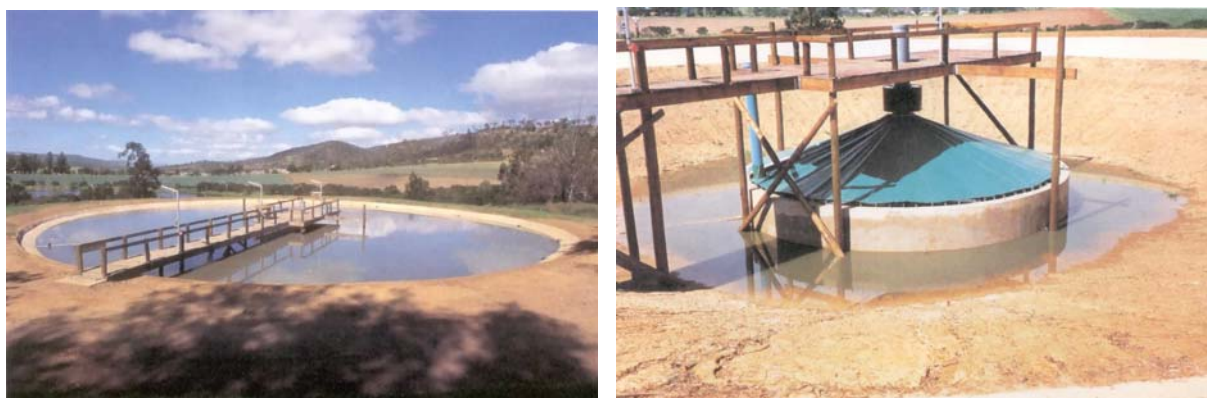
Figure 2. Primary Facultative Pond of the AIWPS Plant, at the Rhodes University Environmental Biotechnology Experimental Field Station, before and after filling. The access bridge leads to the gas collection unit.
