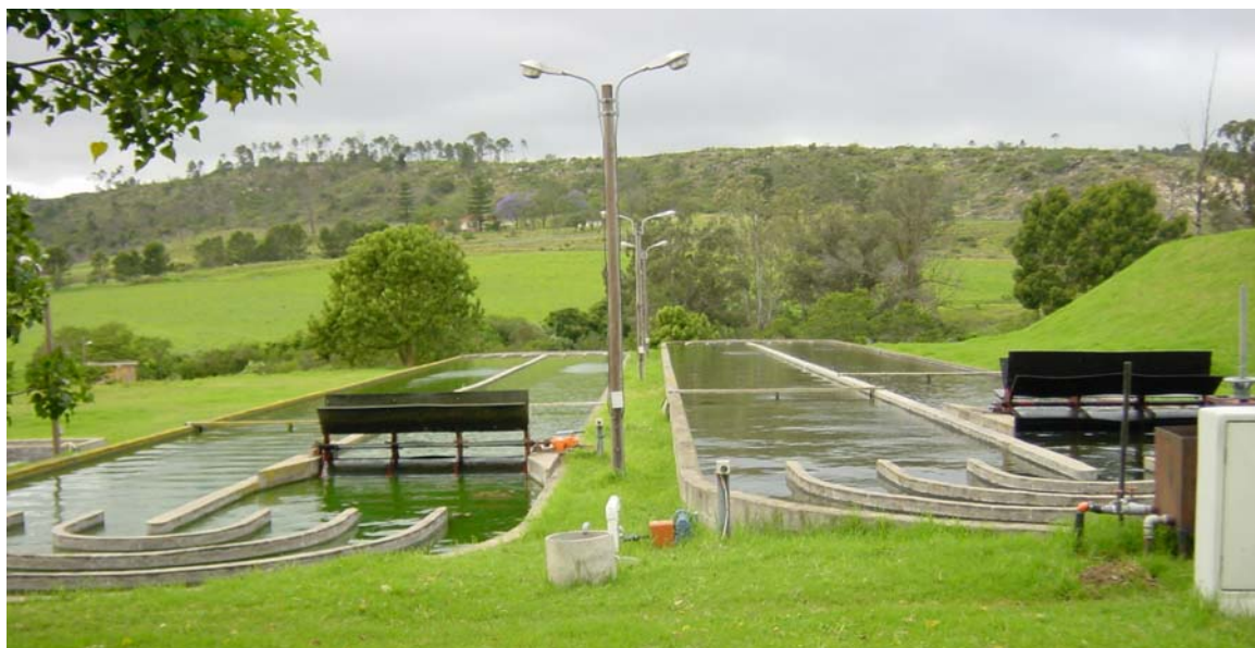
Figure 6.3 High Rate Algal Pond of the AIWPS Plant, at the Rhodes University Environmental Biotechnology Experimental Field Station, showing paddle wheels and the flow path dividing walls.
