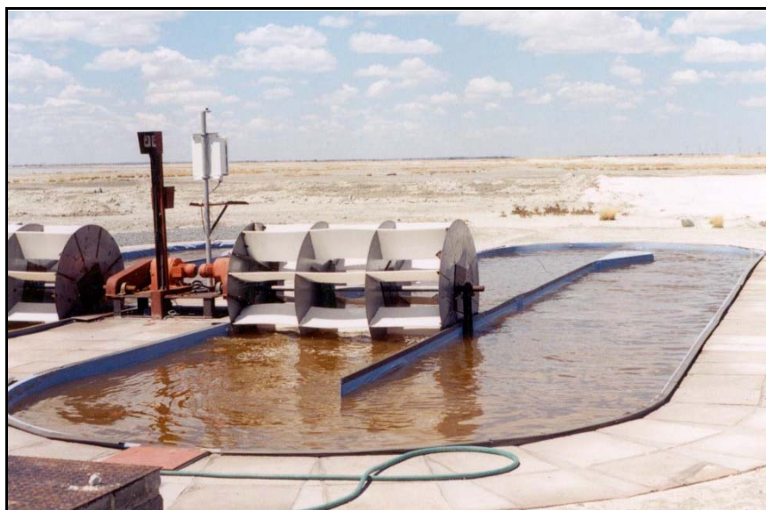
Figure A9.2. The Dunaliella -HRAP pilot plant treating saline carbonate brines at Botswana Ash Co. Sua Pan, Botswana.
