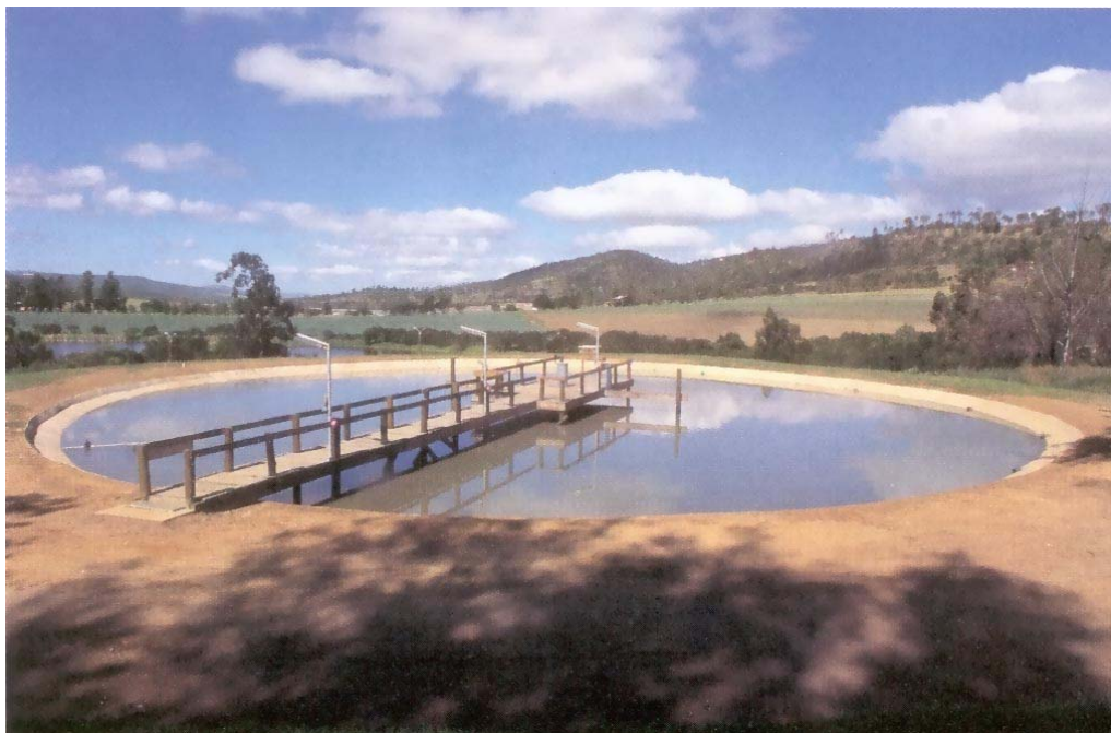
Figure 6.1 Primary Facultative Pond of the AIWPS Plant, at the Rhodes University Environmental Biotechnology Experimental Field Station. The access bridge leads to the gas collection unit.
