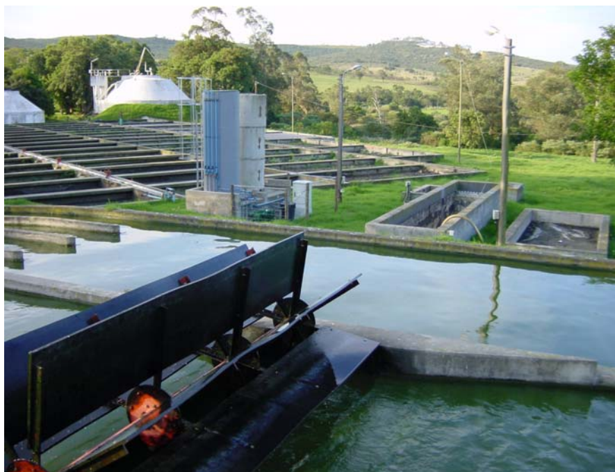
Figure A 9.3. Pilot plant of the Independent High Rate Algal Pond (I-HRAP) unit operation for tertiary treatment and the renovation of raw water at the Environmental Biotechnology Field Station, Grahamstown.
