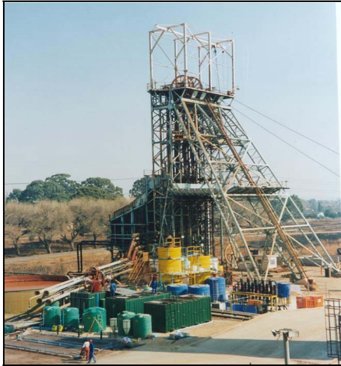
Figure A 9.6 Headgear at the No.4 shaft Grootvlei Mine with the Rhodes ‘BioSURE’ Process pilot plant and I-HRAP raceways in the foreground.
