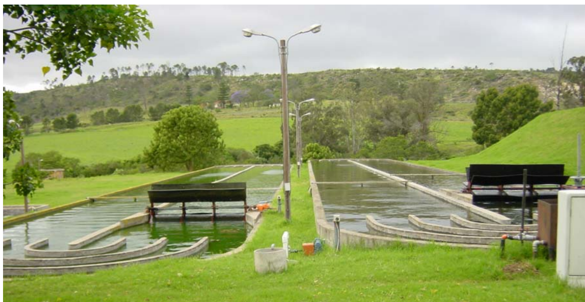
Figure 3. High Rate Algal Pond of the AIWPS Plant, at the Rhodes University Environmental Biotechnology Experimental Field Station, showing paddle wheel and the flow path dividing walls.
