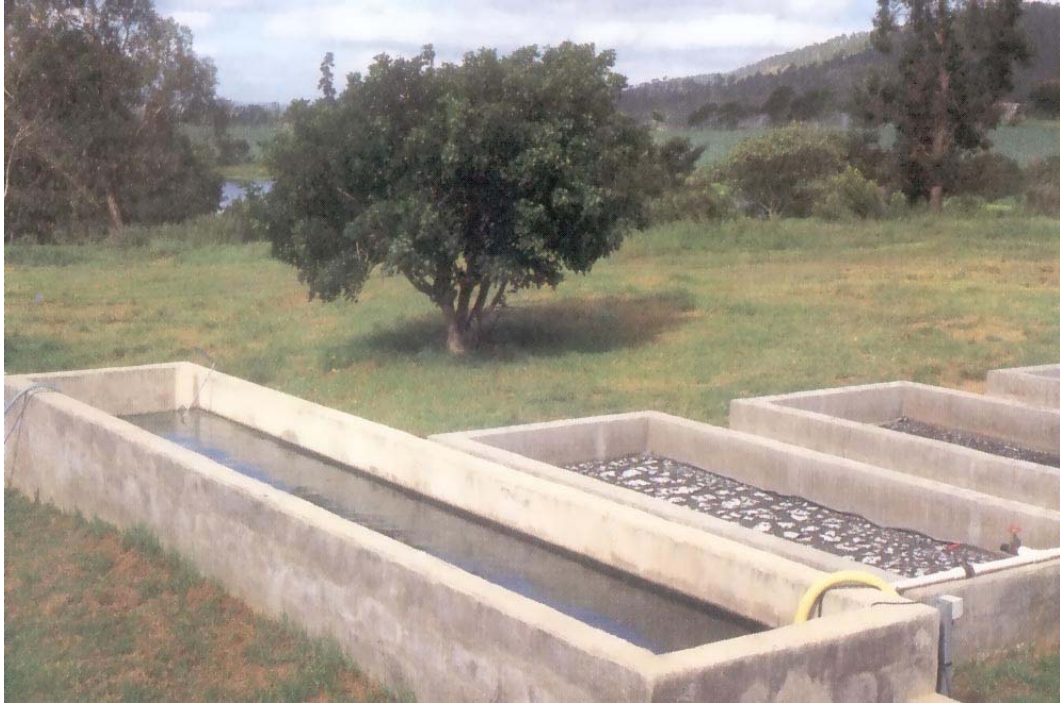
Figure 6.4 Algal Settling Unit in the foreground with three of the four Algal Drying Beds visible behind this unit.
