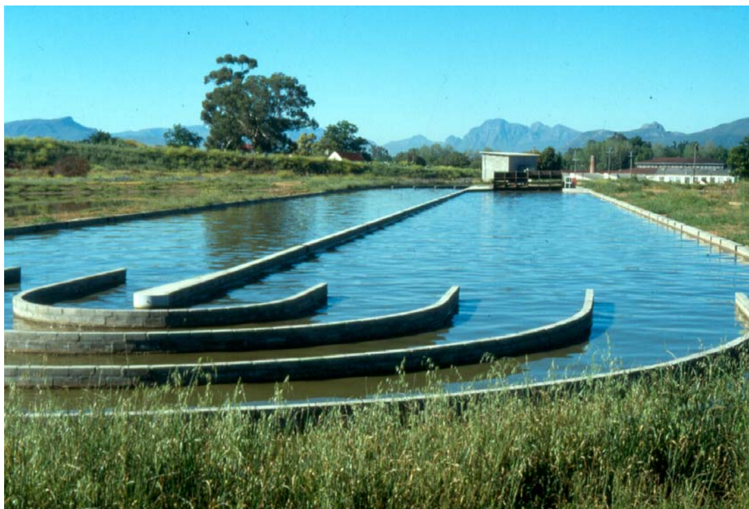
Figure 5.6 The 2 500 m 2 high rate oxidation pond at Mossop-Western Leathers Co., in Wellington, South Africa.
