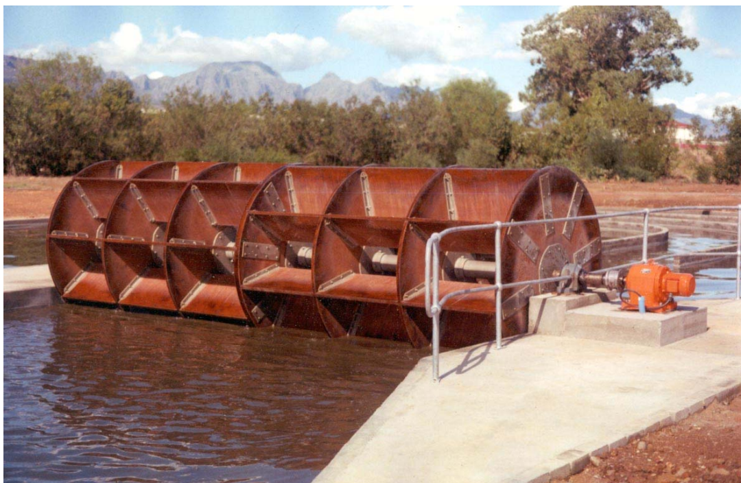
Figure 5.7 Paddle wheel of the High Rate Algal Pond at Mossop-Western Leathers Co., in Wellington.
