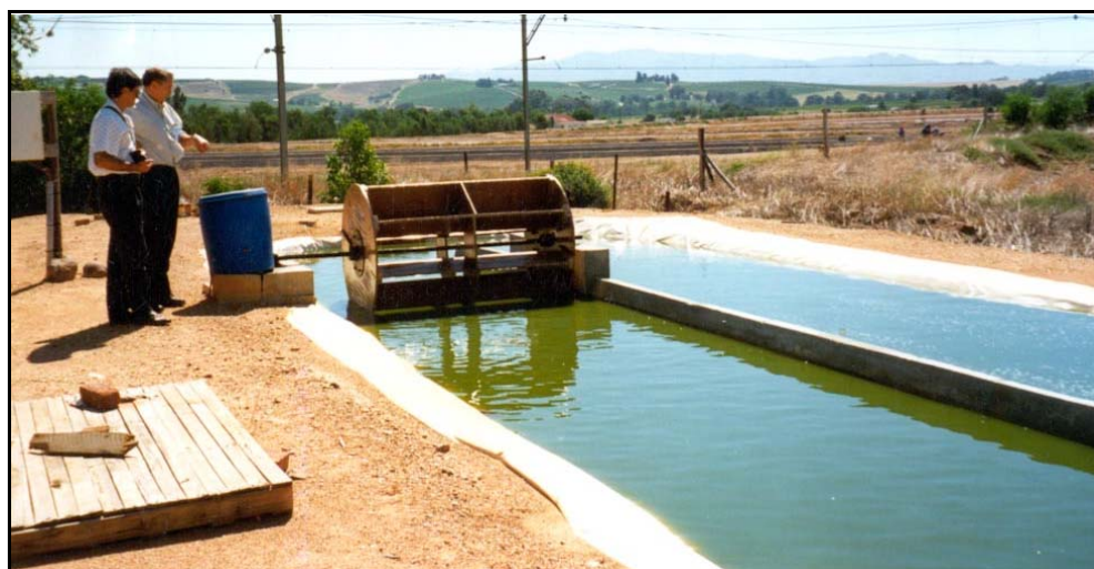
Figure 5.3 The S-HRAP pilot plant constructed at Mossop-Western Leathers Co., Wellington, showing one of the 80 m 2 High Rate Algal Ponds.
