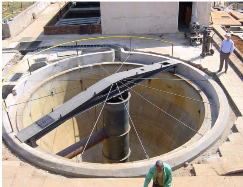
Figure A 4.7. The 2 ML scaled-up Recycling Sludge Bed Reactor in the BioSURE ® sewage sludge solubilisation technical-scale plant constructed at Erwat's Ancor Works in Springs. Surface struts provide supports for a covering membrane.
