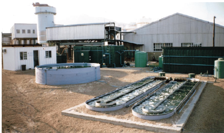
Figure A 4.5. Pilot plant at Brennokem Co., in Worcester, South Africa, evaluating the IAPS in the treatment of wine lees and distillery wastewaters.
