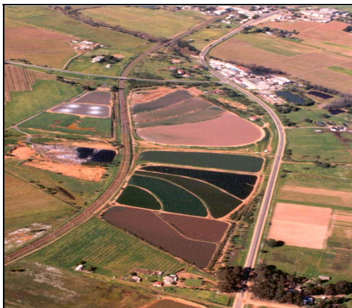
Figure 1.1 The Waste Stabilisation Pond evaporative disposal cascade treating tannery wastewaters at the Mossop-Western Leathers Co. Wellington.
