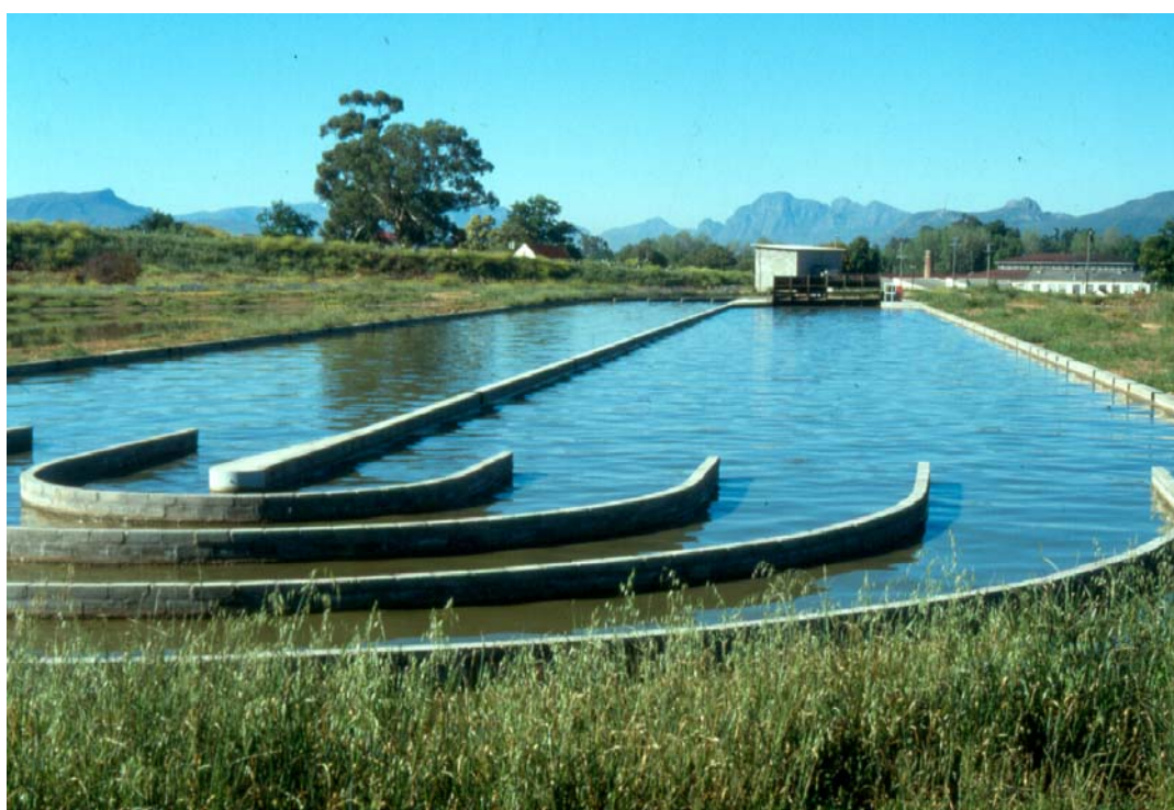
Figure 1. The 2 500 m 2 high rate oxidation pond at Mossop-Western Leathers Co., in Wellington, RSA.
