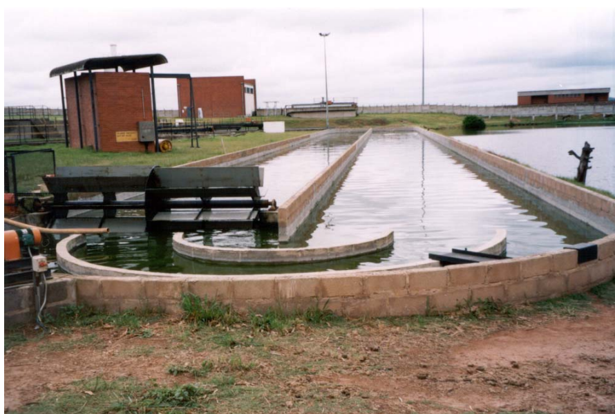
Figure A 4.4 The HRAP unit operation of the IAPS plant constructed at the Cato Ridge Abattoir.
