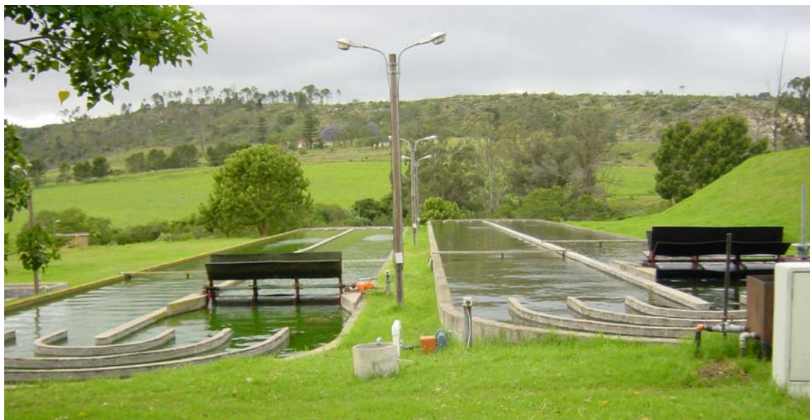
Figure 1.2 The High Rate Algal Pond showing paddle wheel and raceway. This system treating domestic wastewaters was constructed at the Grahamstown Disposal Works.
