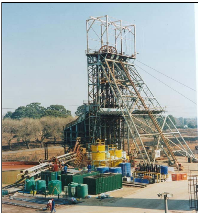
Figure A 4.6 Headgear at the No.4 shaft Grootvlei Mine with the Rhodes 'BioSURE' Process pilot plant in the foreground. Reactors were constructed in shipping containers in Grahamstown, and then transferred to site.
