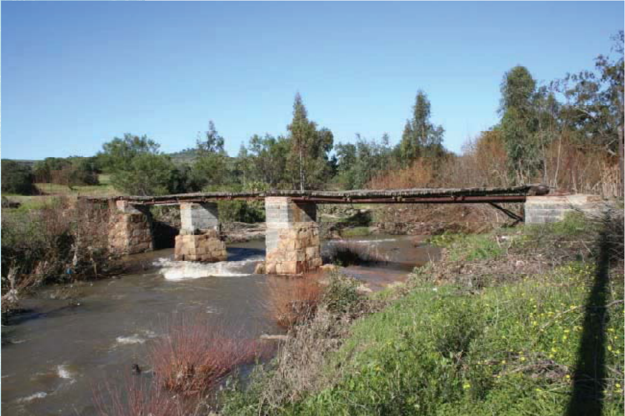
These remnants of the original sandstone foundation pillars of the first bridge built across the Eerste River in 1838 can be seen at Kompanjiesdrif, Welmoed, Lynedoch. (Photo: Charlie Boucher)
