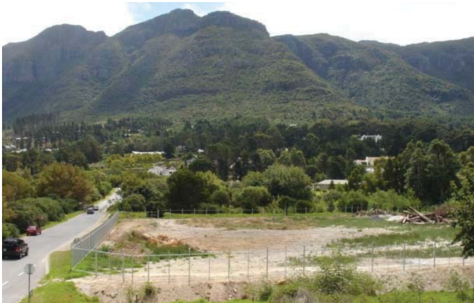
The land alongside the Hout Bay River has been infilled to ensure that it is above the level of the 1:50 year flood. This has had the effect of confining the river to its banks under flood conditions, which exacerbates the erosion problems. This photograph was taken at the corner of Main Road and Disa River Road in February 2008. (Photo: Rembu Magoba)
