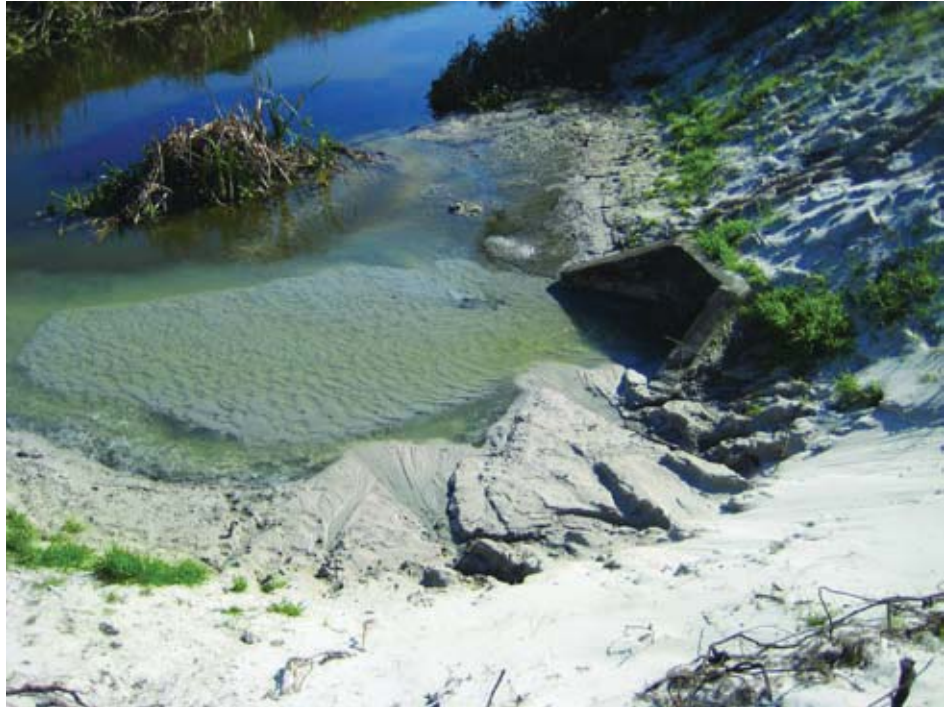
The exit of the cut-off drain that was installed in 2008 in an effort to reduce seepage into Zeekoevlei from the Cape Flats Wastewater Treatment Works (Photo: Roger Godwin)
