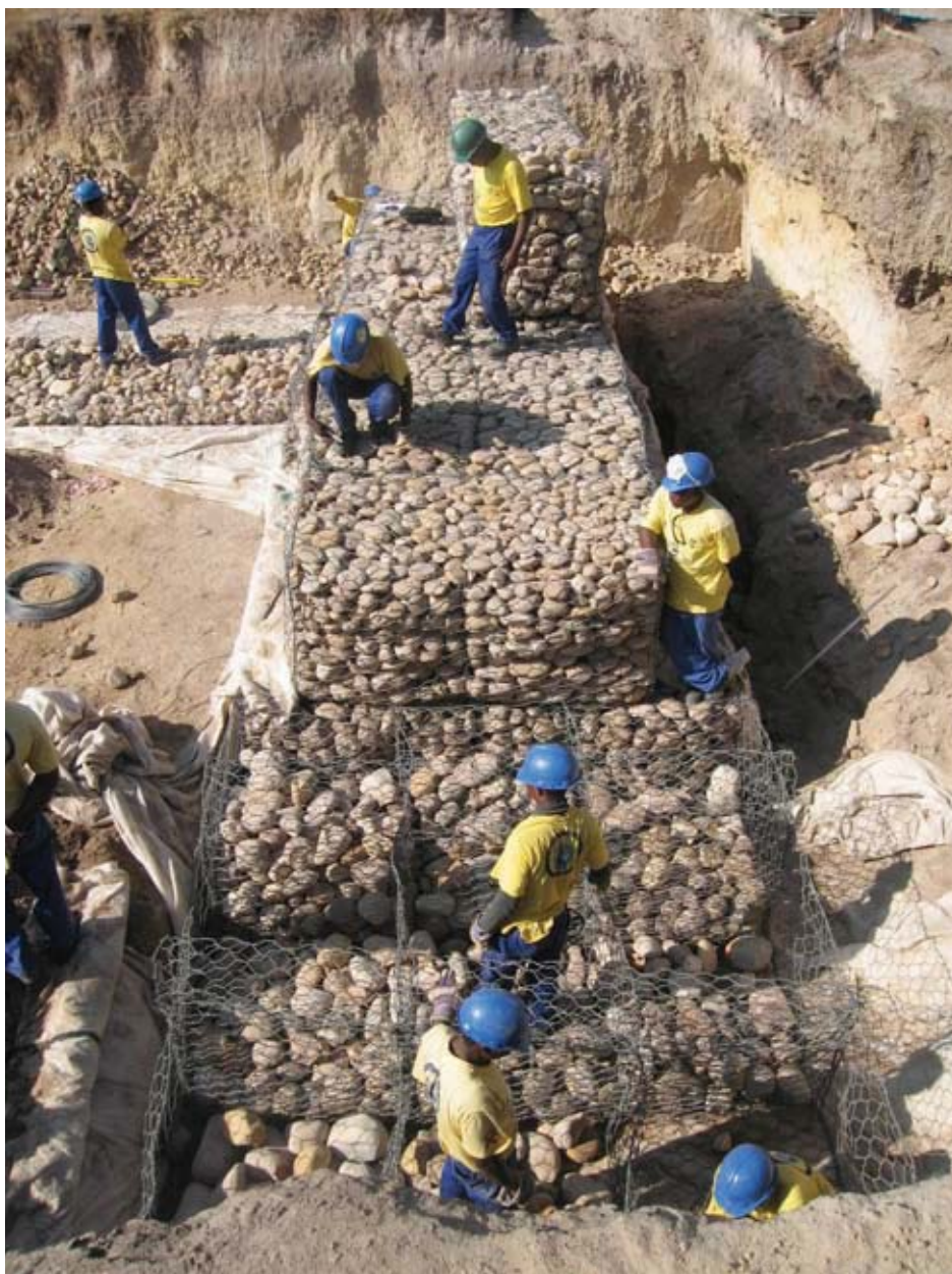
The Working for Wetlands team building gabions (rock baskets) to combat bed and bank erosion on the Princeskasteel River, April 2007 (Photo: Mandy Noffke)
