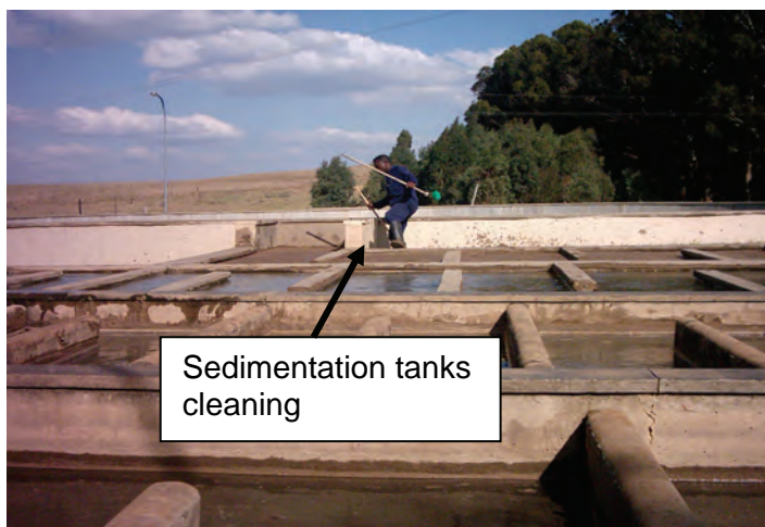
Figure 11: Illustration of sedimentation tanks cleaning
