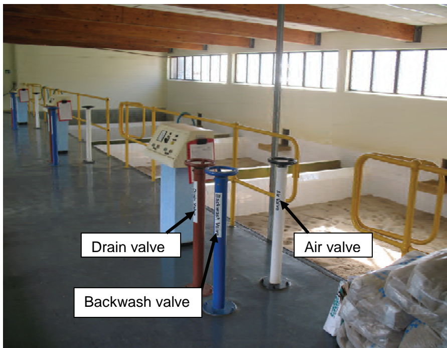
Figure 22: Equipment for rapid sand filters backwash
