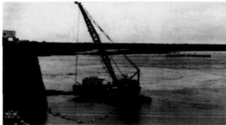
Figure 5.1: Grab dredger - Roseires Dam intake dredging
