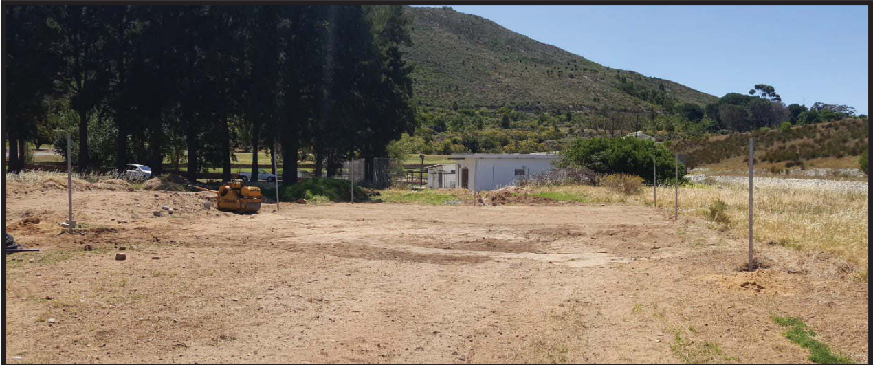
Figure 2.3.4 Site after ground was cleared and leveled by DCS
