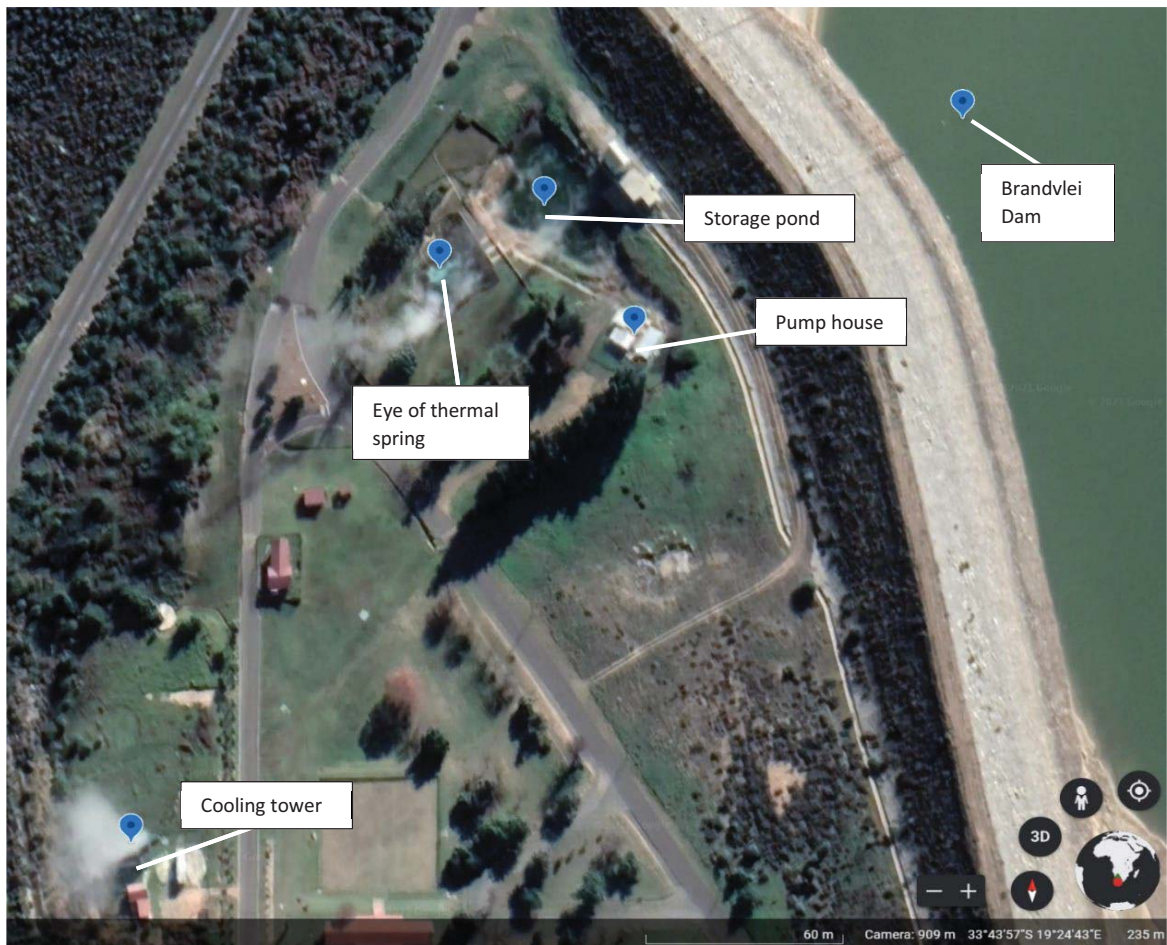
Figure 1.5.3 Aerial view indicating where the thermal water leaves the ground (Eye of Brandvlei thermal spring); the storage pond into which excess water from the eye flows; the pump house pumps water to the cooling towers which cool water for domestic use at the Brandvlei Correctional Facility.
