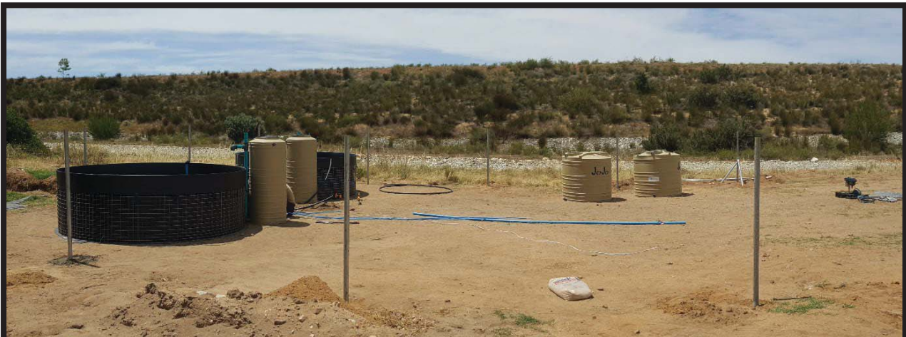
Figure 2.3.5 Site during system installation and cementing of fencing poles
