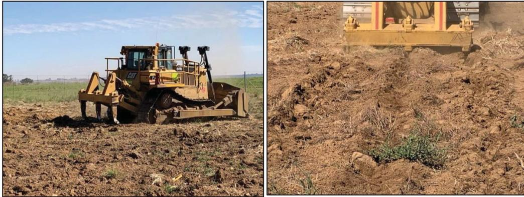
Figure 4.7: A bulldozer with a ripper reducing compaction to 300 mm
