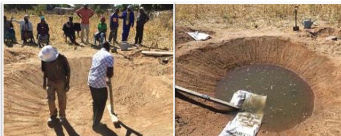
Figure 44: Above Left; tamping down the layer of bentonite which was added after the dam walls and bottom were dug out to provide a wall angle of around 45-60° and Right; careful filling of this pond for the first time to allow for the bentonite to swell evenly and seal the pond (Sedawa, Limpopo).
