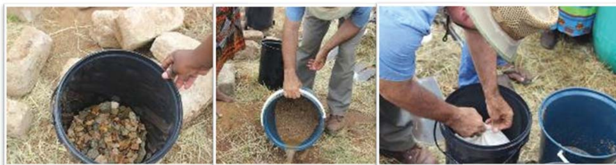
Figure 12: Above Left to Right; gravel and rinsed, clean sand wrapped in a muslin 'bag' make up the filter for the drip irrigation system.
