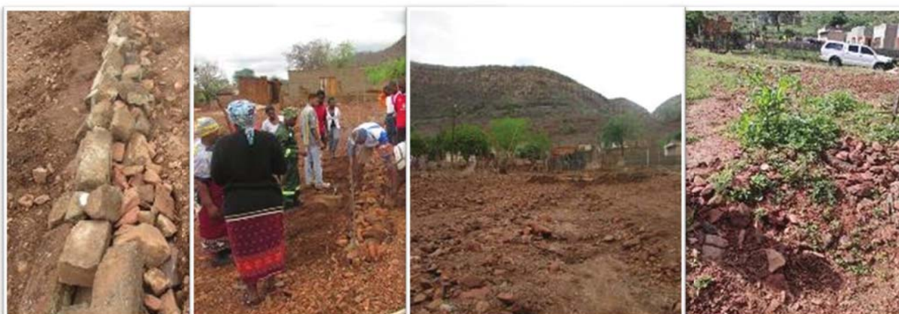
Figure 37: Above left; a close-up of a keyed in stone line,
