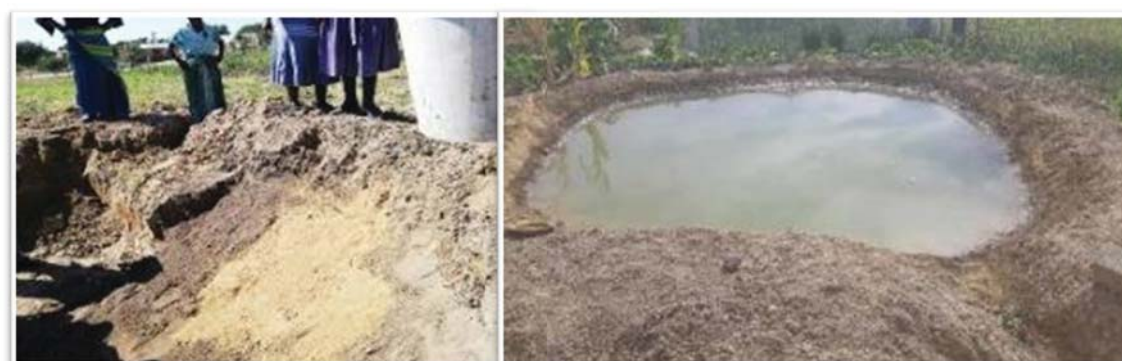
Figure 45: Above left; fixing the wall angles for a small dam in Turkey, Limpopo and Right; the pond filled after attention was also given to the inflow and overflow for the pond.
