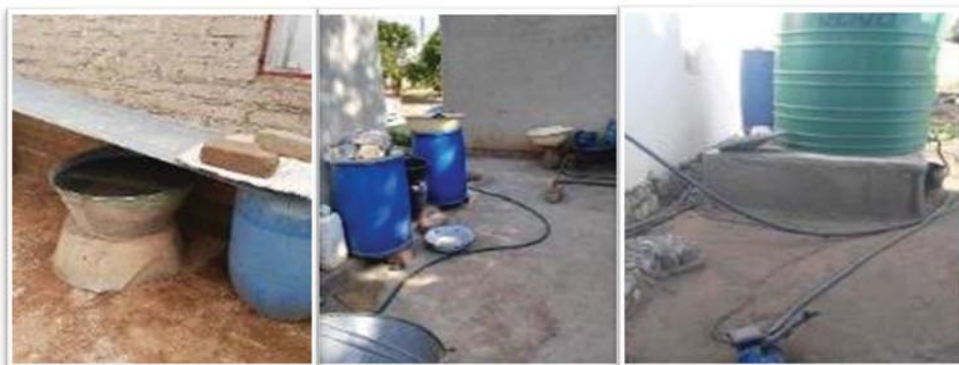
Figure 41: Above Left and Centre; examples of drums and basins used for RWH collection and Right; a 2200 litre Jo-Jo tank for roof rainwater harvesting (Limpopo).
