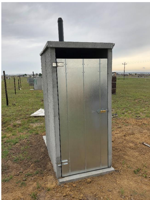
Figure 9: Newly constructed VIP and indicating ability to be connected to water supply (in future, if required)
