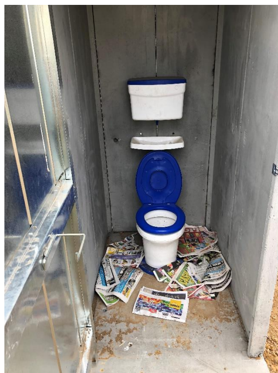
Figure 9: Newly constructed VIP and indicating ability to be connected to water supply (in future, if required)
