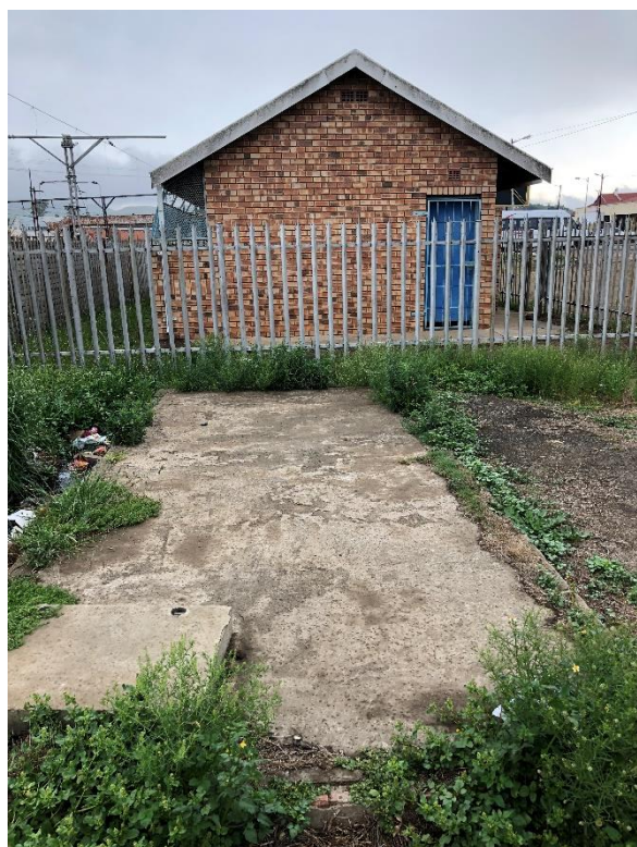
Figure 12: Evidence of leaking from taxi rank public toilet conservancy tank (Dannhauser)
