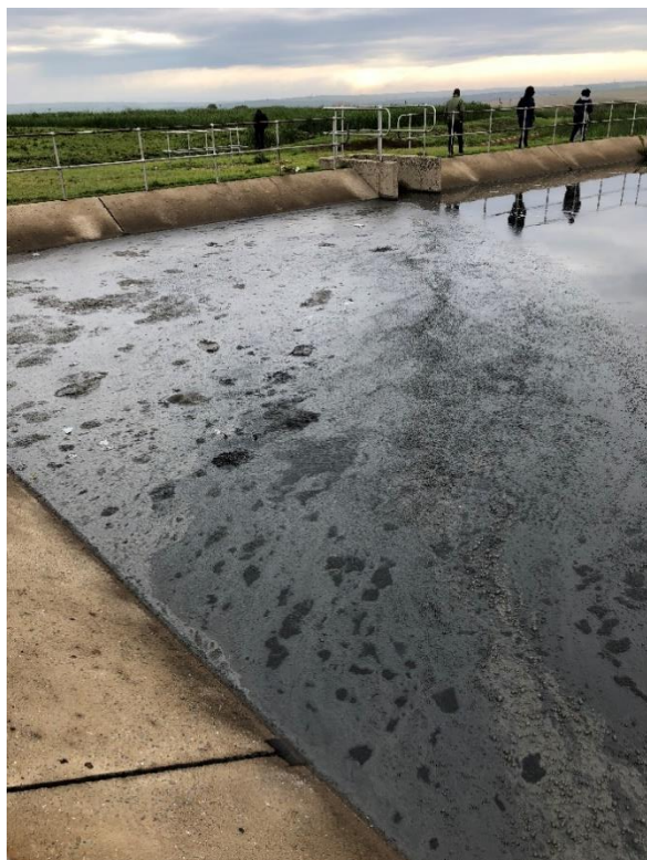
Figure 11: Pond showing accumulated sludge at Dannhauser WWTW (Tweediedale Ponds)
