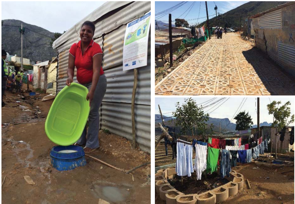
Figure 5. 2: Completed GOS Components (Permeable Paving, Disposal Points, Tree Gardens)
