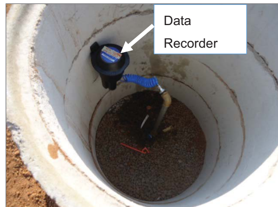
Figure 2: Typical data recorder installation at critical point
