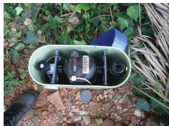
Re-installation of water meter (hiding the data recorder underneath)
