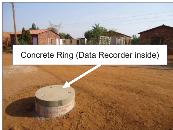
Figure 2: Typical data recorder installation at critical point
