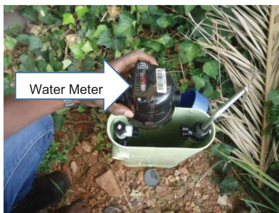
Temporary removal of water meter
