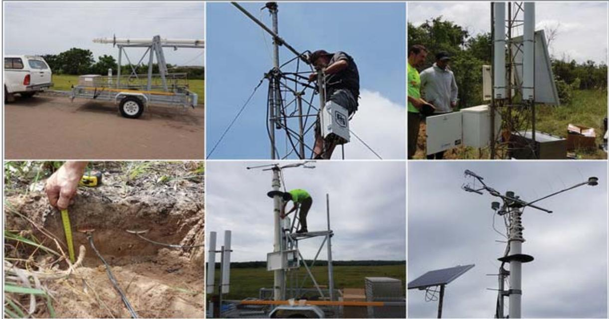
Figure 5.6 Transport and installation of a mobile Eddy Covariance system in the hygrophilus grassland and on a lattice mast in the indigenous forest
