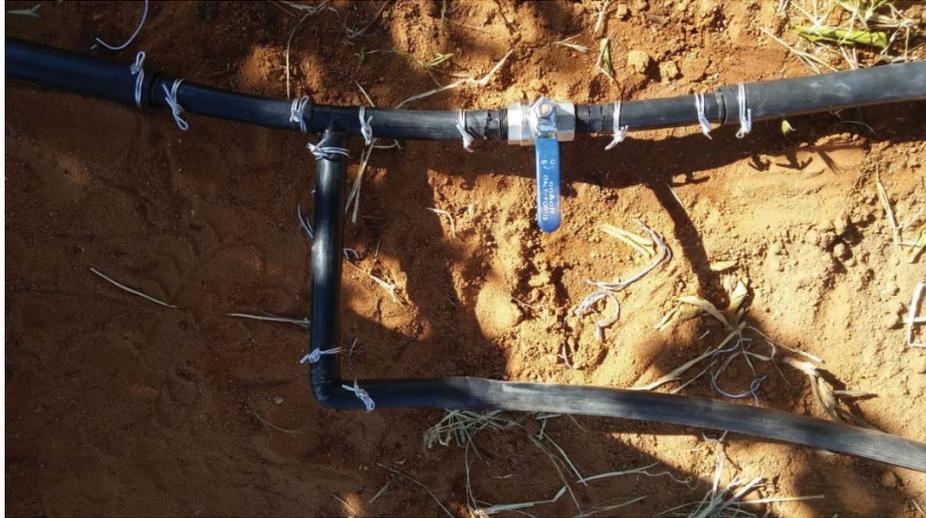
**Figure 3.18** Installation of the extra irrigation line
