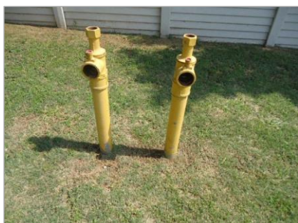
Figure 10: Double hydrant used to separate water management zones in the City of Tshwane
