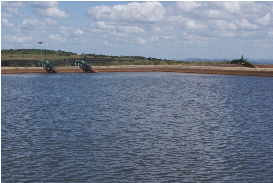
Figure 2-13: View of the balancing dam at the BRWTW
