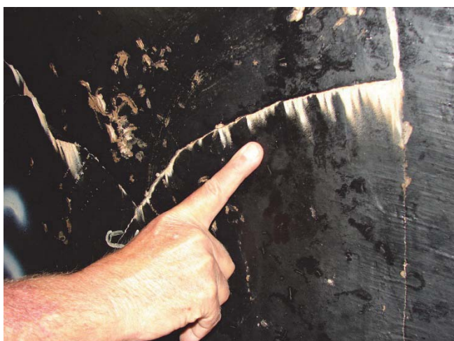
Figure 4-3: Typical view of the internal conditions of a pipeline with little or no biofouling (Option 1)
