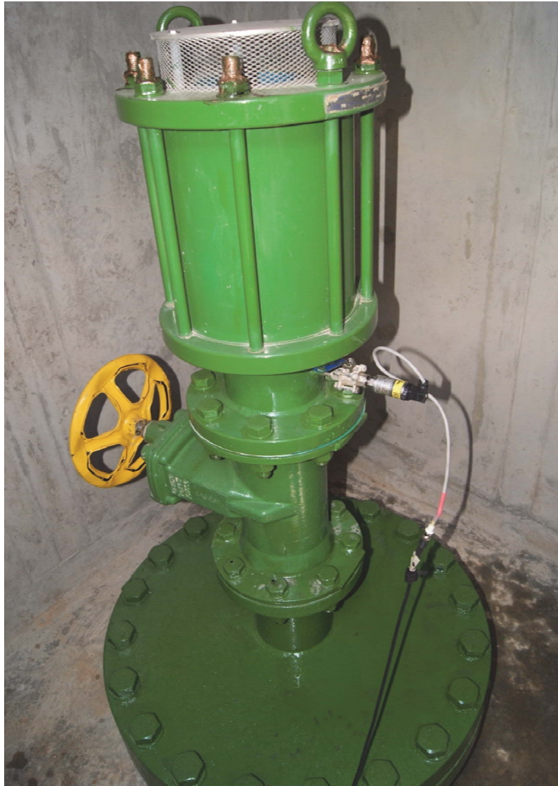
Figure 5-3: Pressure tapping position on an air valve body
