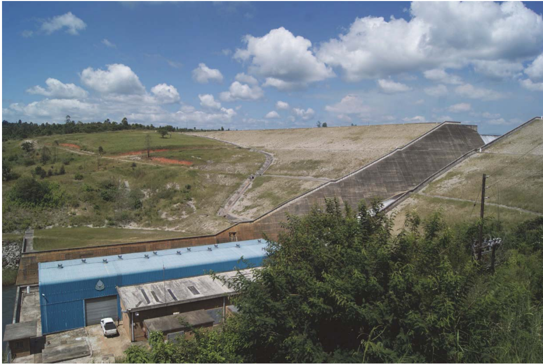
Figure 2-12: Pump Station at Inyaka Dam
