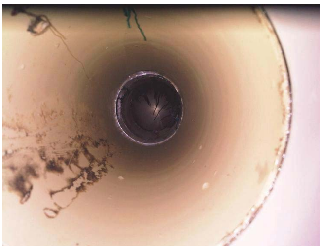
Figure 4-4: Typical view of the internal conditions of a pipeline with some biofilm growth but without residual material in the biofilm (Option 2A)
