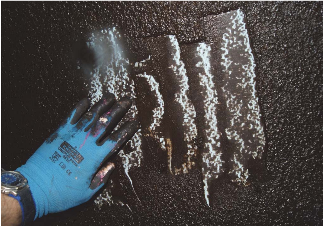
Figure 4-1 : Example of biofilm growth (MOB) in large diameter pipelines (Blyde River Irrigation System)
