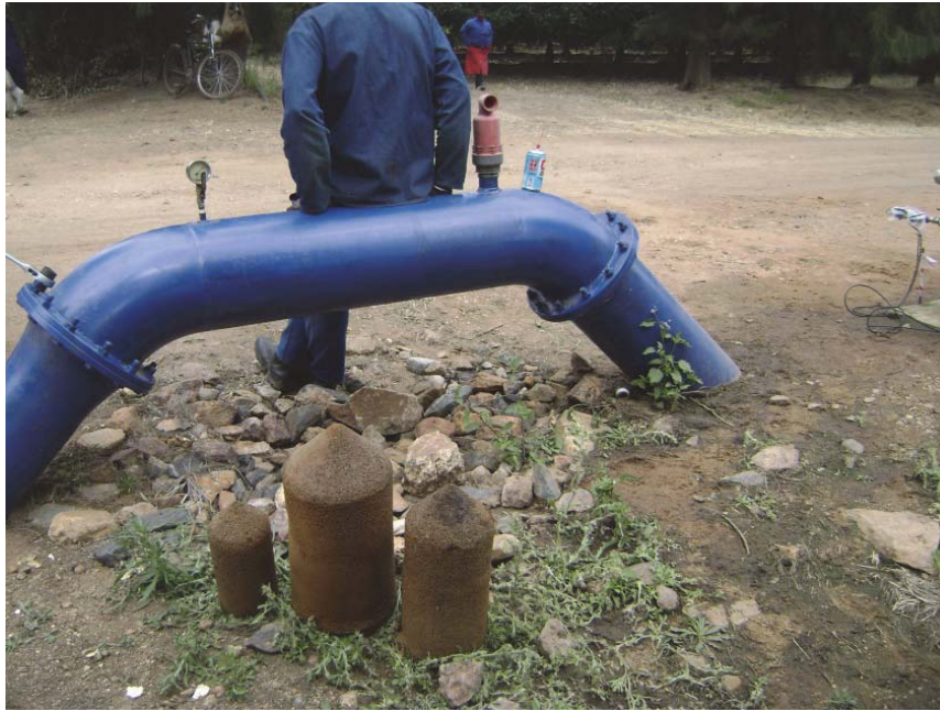
Figure 5-6: Examples of a pig station on a 250 mm pipeline
