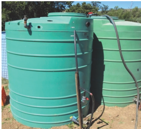
Figure C.2 Slow sand filtration as a tertiary treatment unit (TTU) to IAPS. Left: slow sand filter (SSF) contained inside a 1500 L Jojo ® tank. Right: schematic of the SSF comprising of a layer of fine sand overlaying a layer of gravel each separated by GeoFabric.
