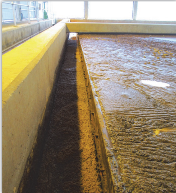
Backwash reservoir, water for cleaning the GAC, PAC and sand-filters
