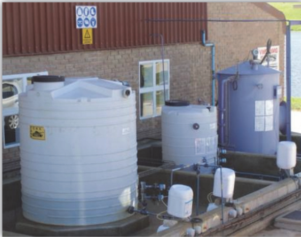
1000 l anti-scalant storage tank
