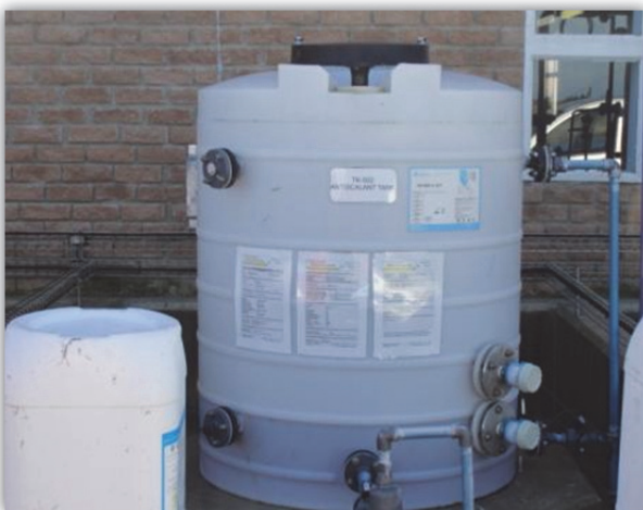
1000 l anti-scalant storage tank
