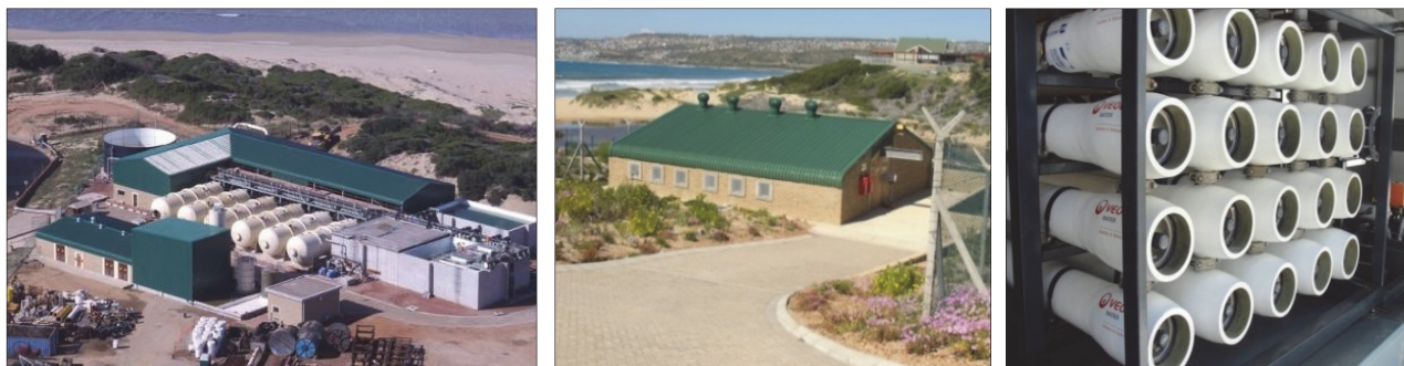
Figure 2.1: Mossel Bay SWRO plant
