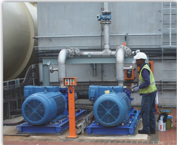
SMBS and Anti-scalant storage and dosing units
