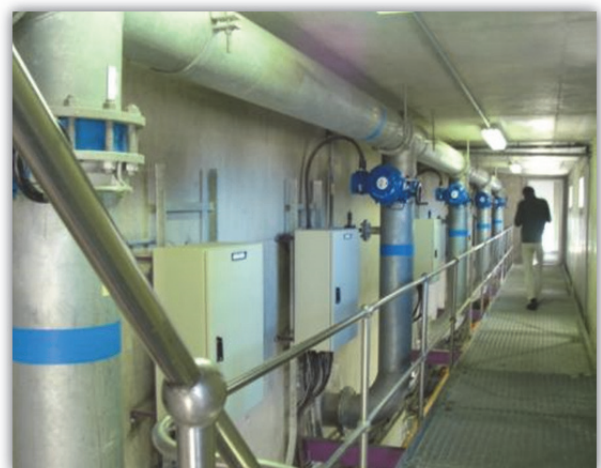
Maintenance floor: Backwash pumps & compressors
