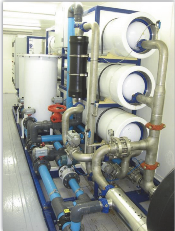
Pressure exchanger energy recovery system
