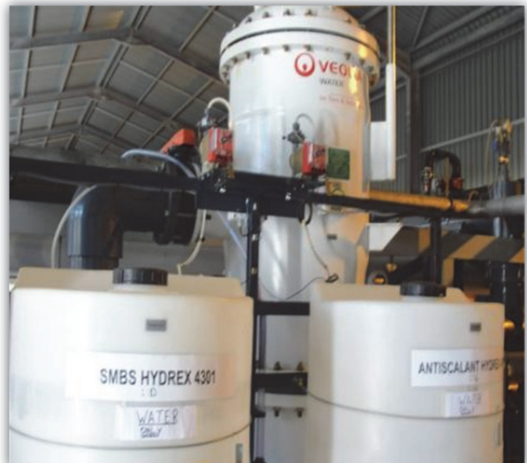
SMBS and Anti-scalant storage and dosing units
