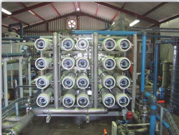
Single pass seawater reverse osmosis (1.4 Ml/d + 0.26 Ml/d)
