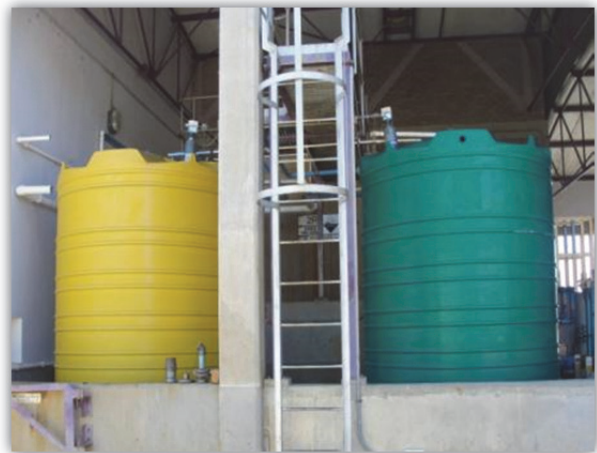
Ferric Chloride: day- and bulk tanks
