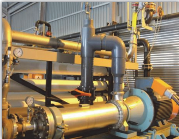
Remineralisation by soda ash & calcium chloride, disinfection by chlorination
