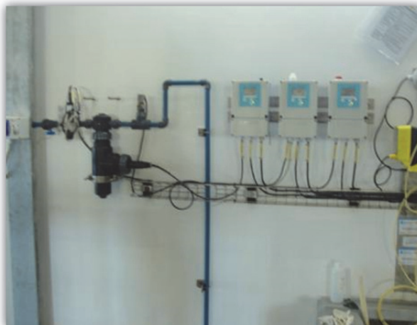
CIP unit for both UF and RO
