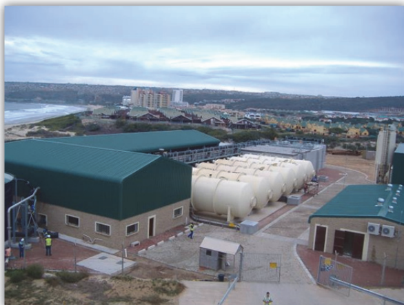
Chemical conditioning & multi-media filtration
