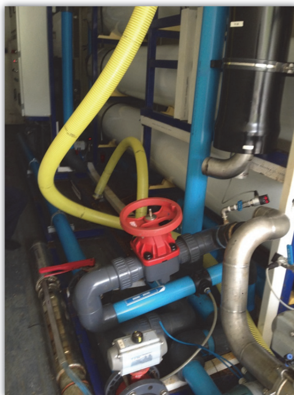
Pressure exchange recovery device
