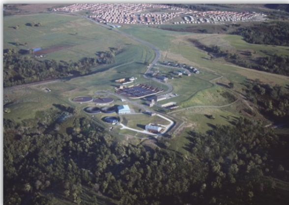
Aerial view of UF Plant
