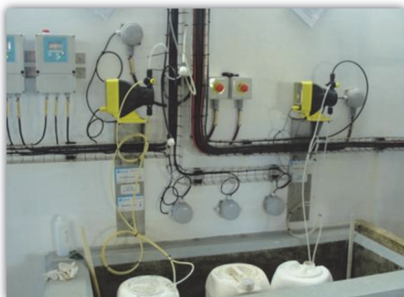
Second dosing equipment for dosing SMBS to neutralise biocide
