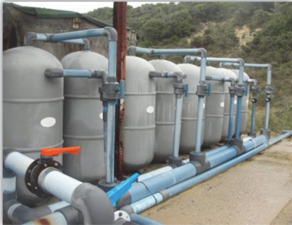
Single pass seawater reverse osmosis (1.4 Ml/d + 0.26 Ml/d)
