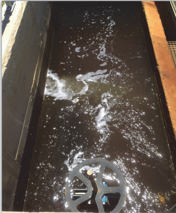
Raw water feed line to sand filters
