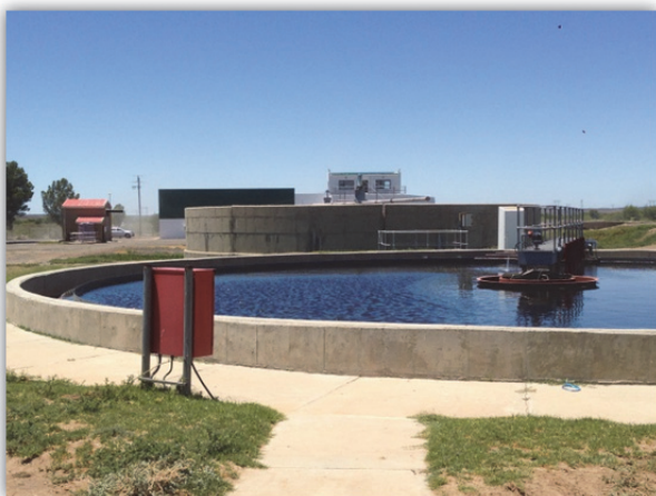
Final settling tanks
