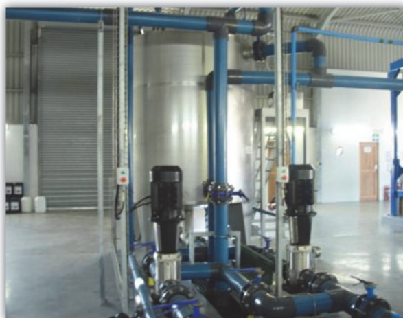
CIP unit for both UF and RO
