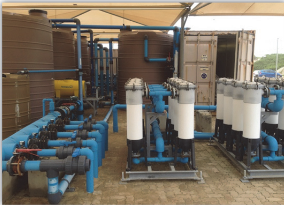
Cartridge filtration – Micro-filters (5 \mu\text{m} )
