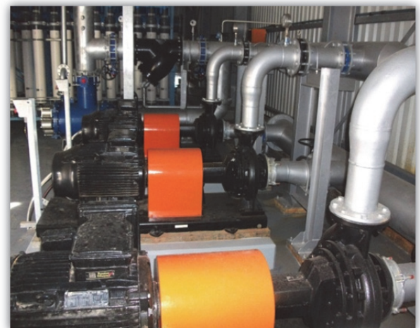
3 Pumps (2 duty and 1 standby) and piping to feed UF trains
