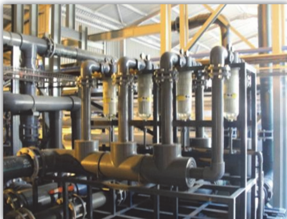
RO cartridge filters, pressure vessels and pipework
