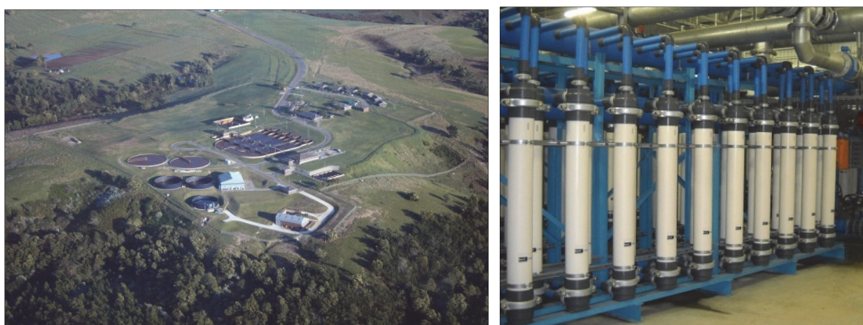
Figure 3.19: George water reclamation plant
