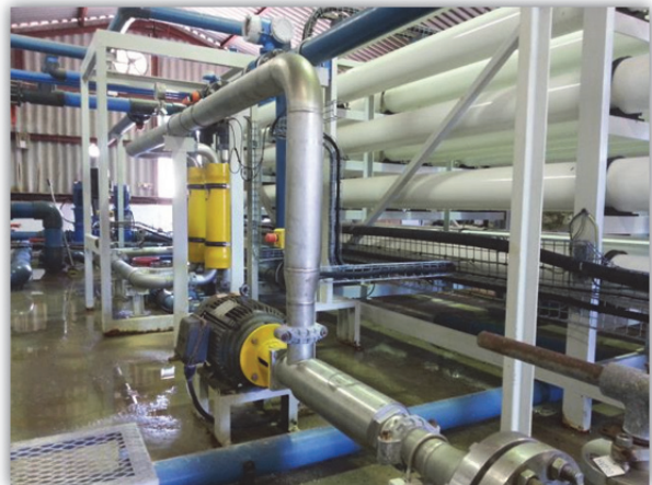
Pressure exchanger energy recovery system (part 80%)
