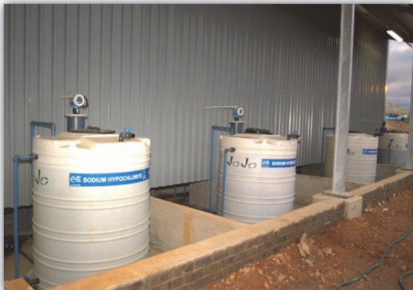
Chemical Dosing Tank Area
