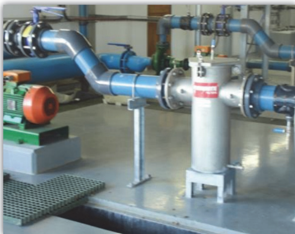
1 of 2 basket strainer housing units upfront the ultrafiltration units (UF)
