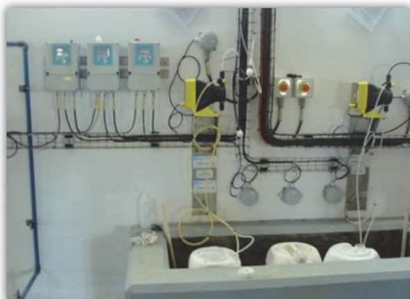
Second dosing equipment for dosing SMBS to neutralise biocide
