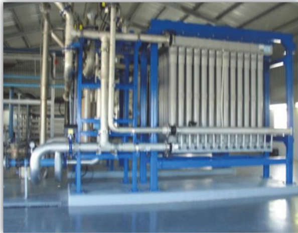
1 of 2 basket strainer housing units upfront the ultrafiltration units (UF)
