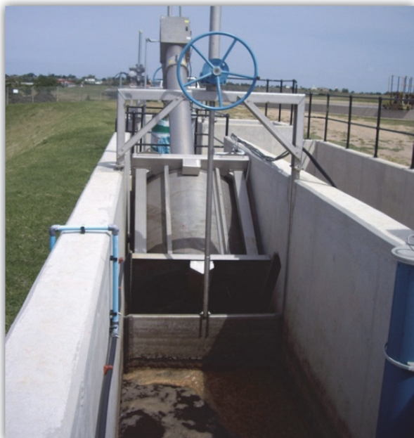
Screen Chamber (Feed from Secondary Settling Tanks)
