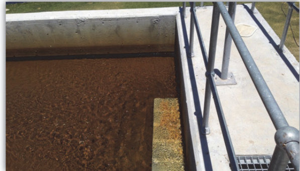
Rapid gravity sand filters
