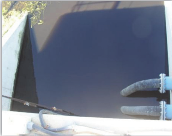
Uptake pipe work to coagulant unit process
