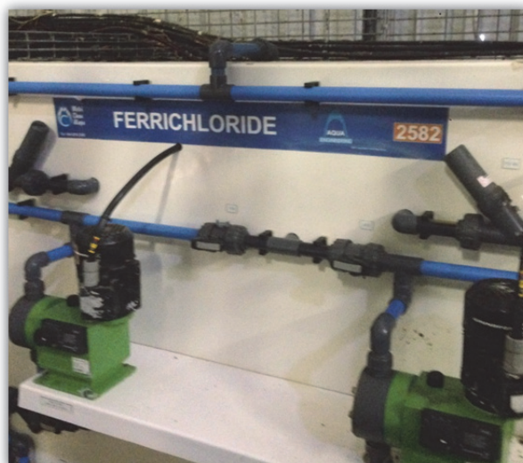
Chemical dosing system: Ferric Chloride
