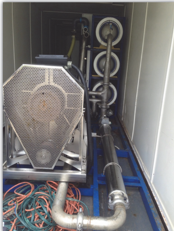
Pressure exchange recovery device
