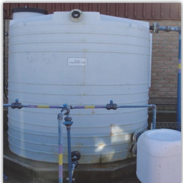
5000 l coagulant storage tank
