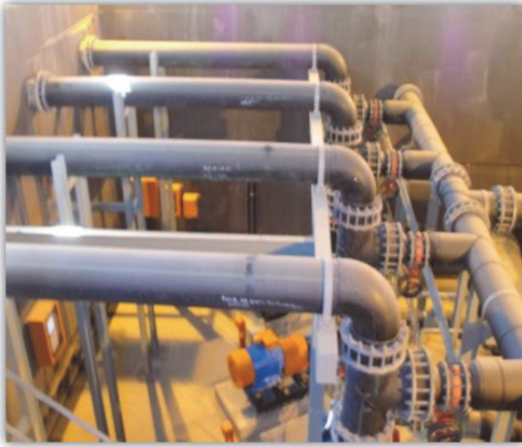
Turbo energy recovery system High pressure pump 40 bar
