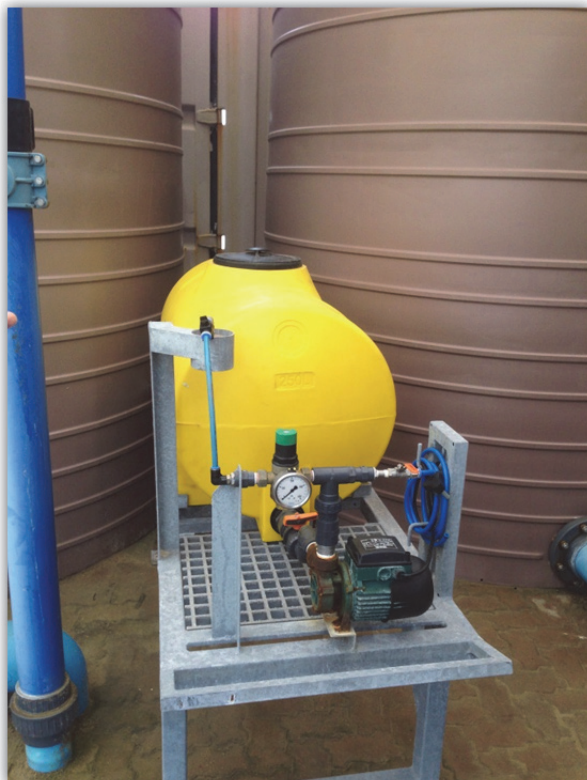
RO Train (2) with high pressure pump
