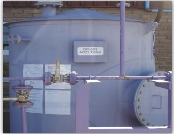
5000 l coagulant storage tank
