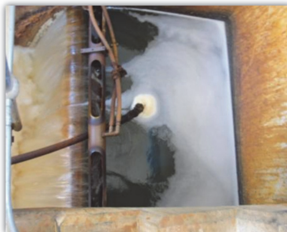
1 of 2 Hydraulic jump: Ozonation foaming
