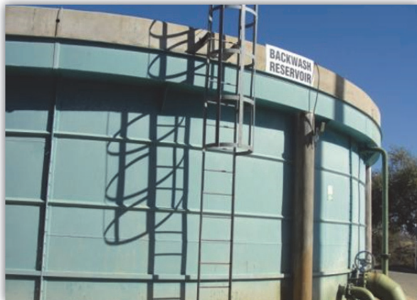
Backwash reservoir, water for cleaning the GAC, PAC and sand-filters
