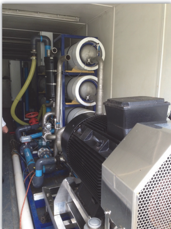
RO Train (2) with high pressure pump
