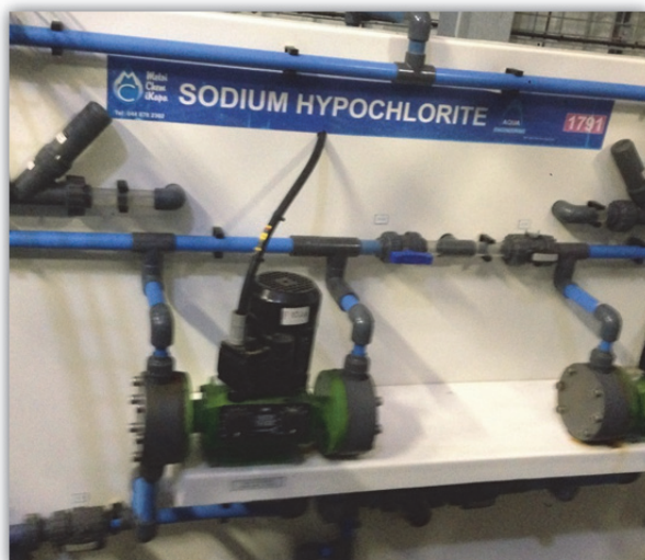
Chemical dosing system: Sodium Hypochlorite
