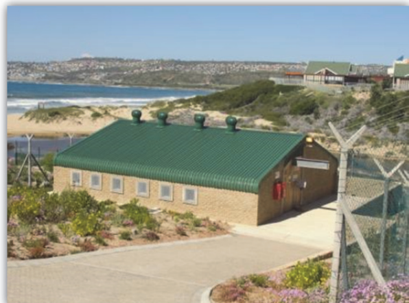
Seawater pump station (floor level 2 m+MSL)
