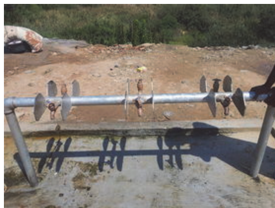
Figure 59 A Typical "Standpipe Unit" in Kya Sands Informal Settlement 73
