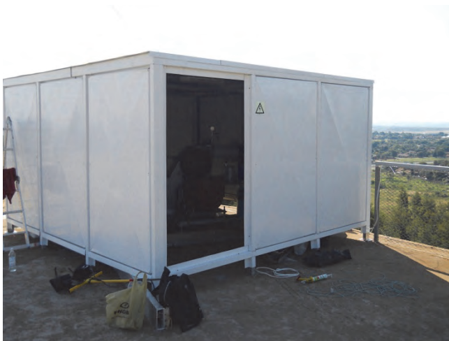
Figure 10-15: Pilot plant enclosure
