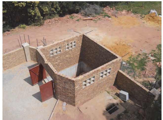
Figure 10-4: Nearly complete off take chamber (Pierre van Ryneveld Reservoir)
