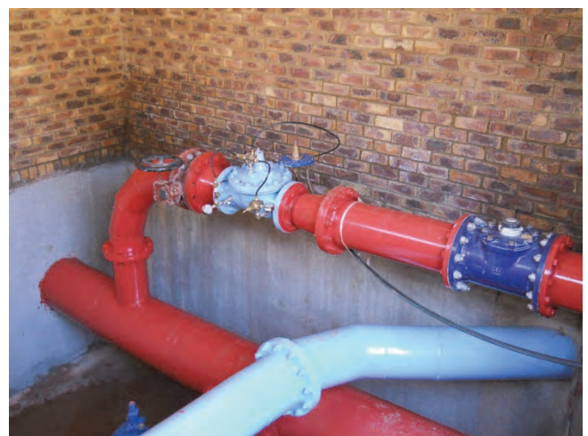
Figure 10-6: Completed off-take chamber pipework
