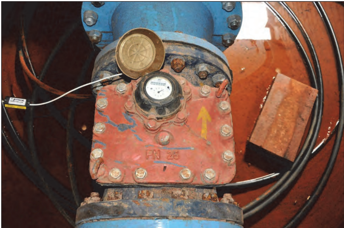
Figure 8-23: Flow measurement at Pierre van Ryneveld Reservoir
