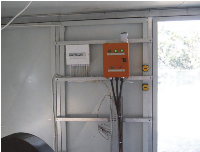
Figure 10-13: Electrical switch over (grid power or hydropower)
