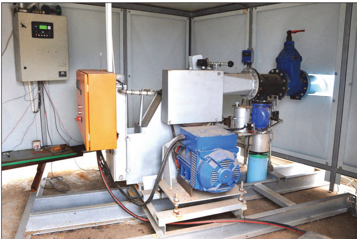
Figure 8-36: Completed turbine on steel-beam supports
