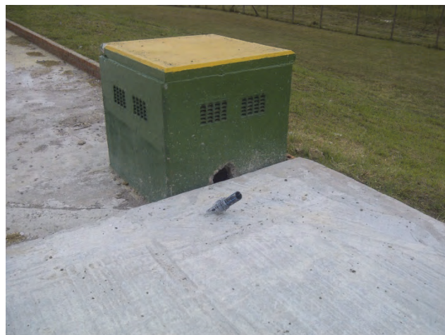
Figure 10-29: Turbine room foundation and connection point into reservoir
