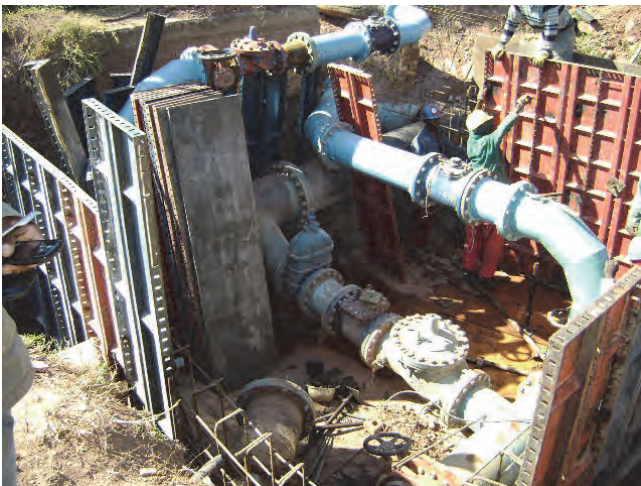
Figure 10-3: Constructing the off-take chamber
