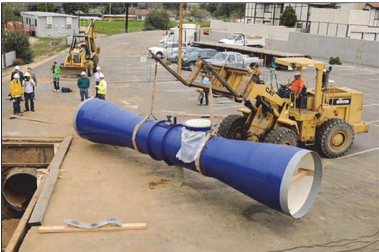
Figure 2-30: Installing the PowerPipe™
