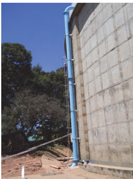
Figure 10-5: Completed turbine supply line on to top of reservoir
