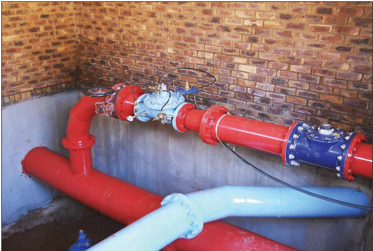
Figure 8-35: Completed off-take pipework
