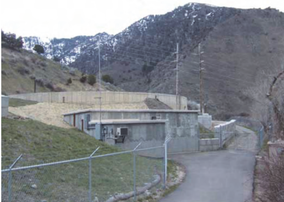
Figure 2-27: The pressure control vault houses the turbine and bypass PRV (White ,2011)
