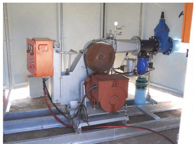
Figure 10-12: Completed installation of turbine, generator and electrical controls
