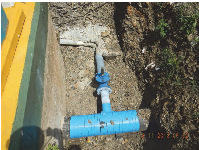
Figure 10-28: Connection point (off take from main supply)
