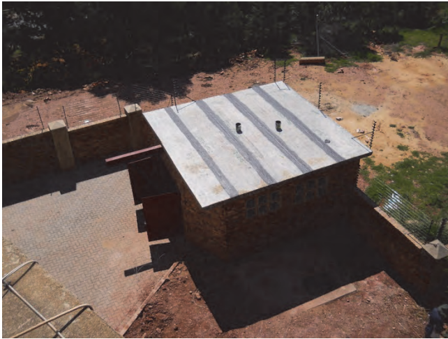
Figure 10-7: Completed off take chamber
