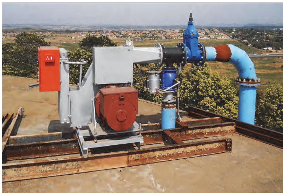
Figure 8-21: Existing Pierre van Ryneveld Reservoir hydropower installation
