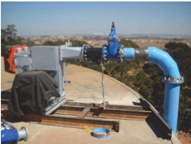
Figure 10-9: Crossflow turbine installation (connecting to supply line)
