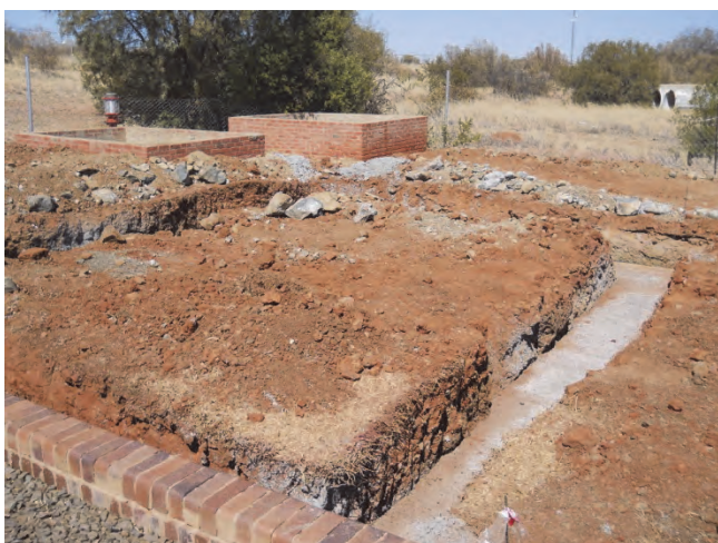
Figure 10-19: Turbine room foundation
