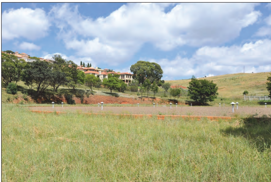
Figure 8-44: Waterkloof Reservoir roof
