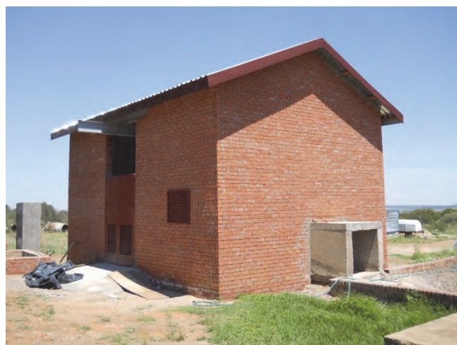
Figure 10-20: Turbine room almost complete
