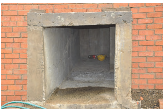
Figure 10-21: Outlet canal into reservoir
