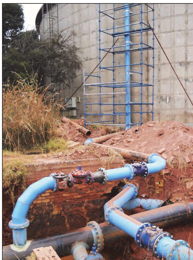
Figure 8-34: Pierre van Ryneveld off-take pipework under construction
