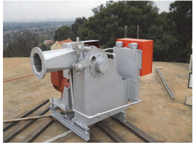
Figure 10-8: Crossflow turbine hoisted onto the reservoir roof
