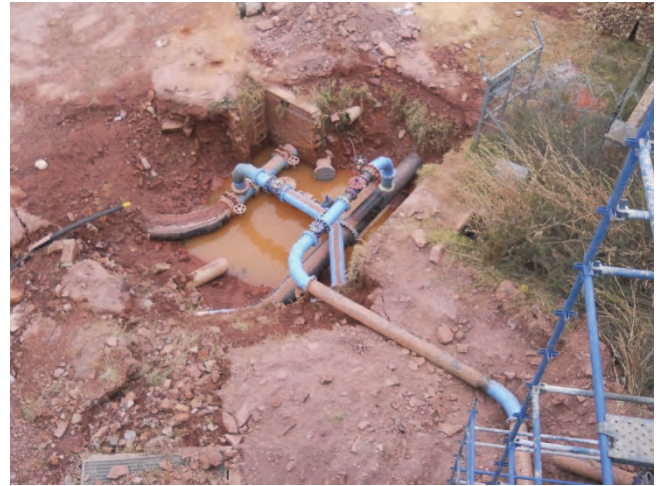
Figure 10-2: Plan view of off take pipework
