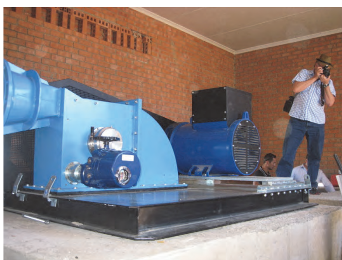
Figure 10-24: Turbine and generator in position
