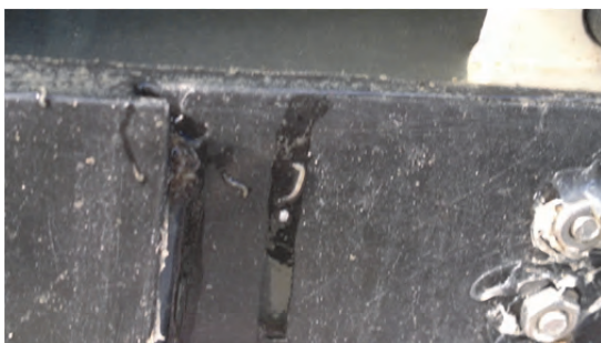
Figure 78: Worms in the RBC as a result of low flowrates (nuts on the right are 6 mm).
