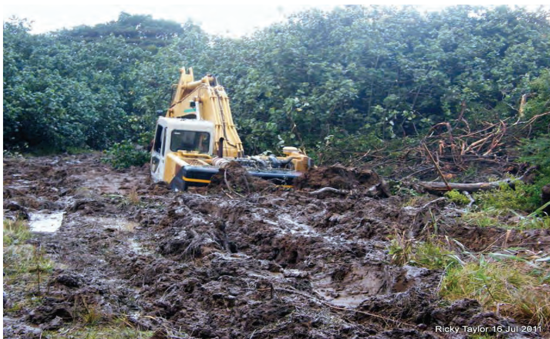
Figure 107: The long-boom excavator stuck in the silt while working on the additional outlet for the Back Channel. Its tracks are not visible as they are completely under the mud.
