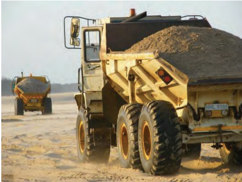
Figure 65: Tippers bringing sand to a stockpile area on the beach to be able to close the Mfolozi Mouth. (Photo R Taylor).
