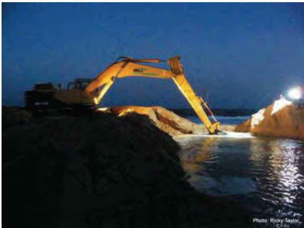
Figure 96. Breaching the Mfolozi estuary mouth on the evening of 14 May 2010.
