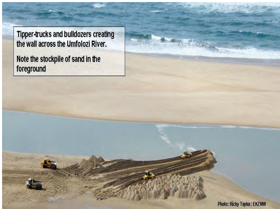
Figure 64. Closing the Mfolozi Mouth
