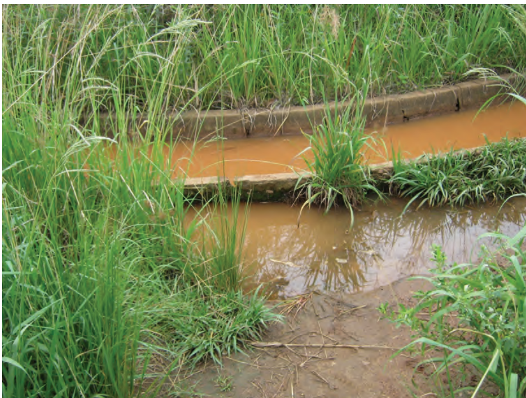
PLATE 3.4: An example of a ‘major leakage’ in the main canal of Dzindi
