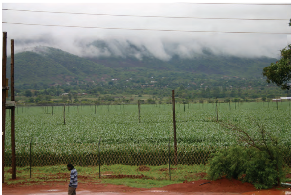
PLATE 2.1: Revitalisation of Tshiombo Block 1A replaced the secondary canals and concrete furrows that conveyed water to the edge of individual farmers' fields with a centrally operated floppy sprinkler system that covers the entire hydraulic unit
