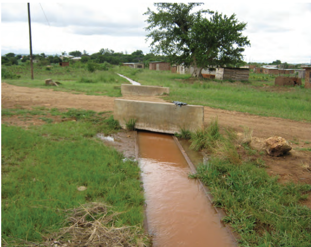
PLATE 3.10: This part of the canal was characterised by a thick layer of sediment, which appeared to be the cause of the overflowing that occurred
