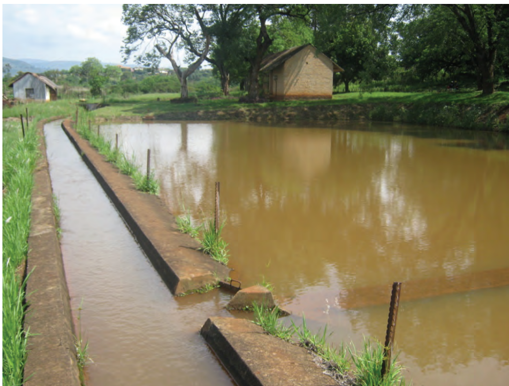
PLATE 3.12: The height of the water in the fish farming ponds at the Dzindi nature reserve are in perpetual equilibrium with the water level in the canal
