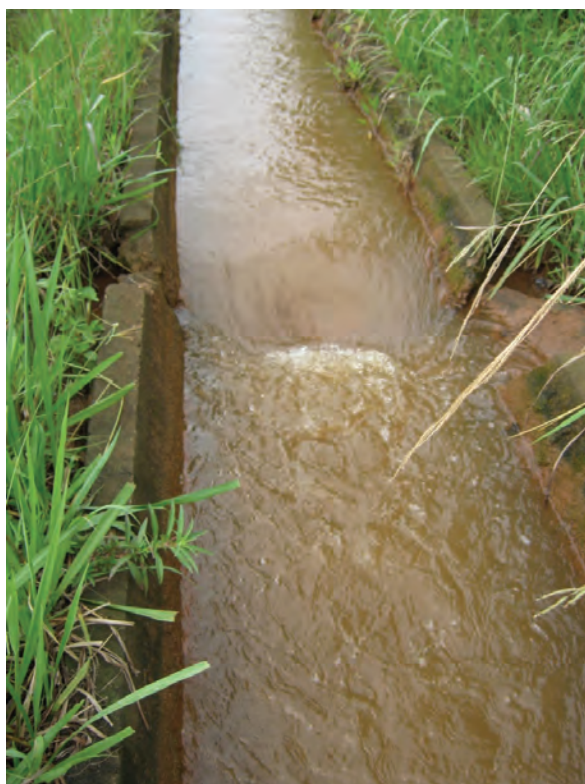
PLATE 3.11: A 'large' stone placed in the main canal increases the water level ahead of it and creates turbulence in the water flow behind it
