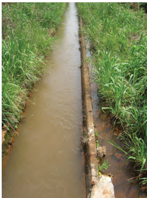
PLATE 3.3: Canal section in which more than 50% of right-hand side of the canal is affected by soil removal (high extent) and where in places the depth of soil removal exceeds 30 cm ('deep removal')
