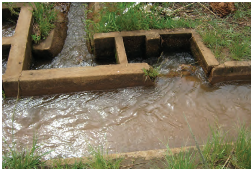
PLATE 3.16: The dysfunctional division box at Block 3
