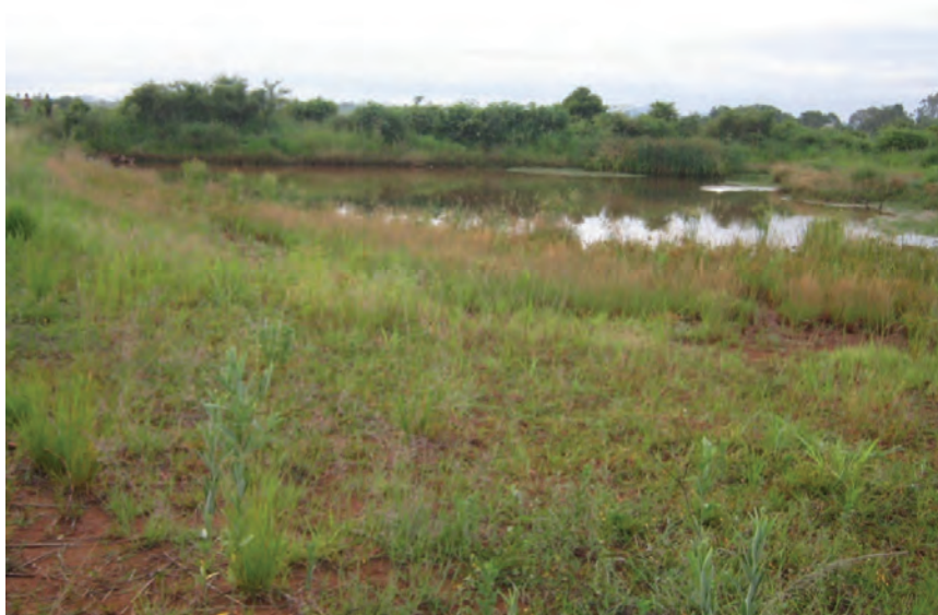
PLATE 3.18: The over-night storage dam at Block 1 is dysfunctional due to a missing outlet valve and urgently needs removal of sediments and plants
