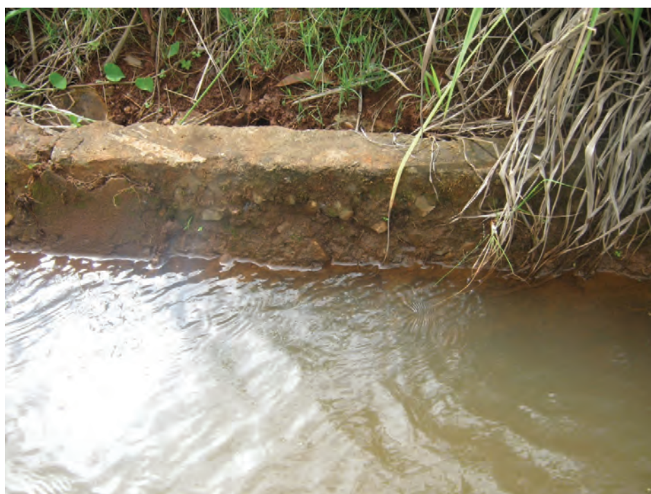
PLATE 3.1: Example of a 'severely roughened' canal lining surface
