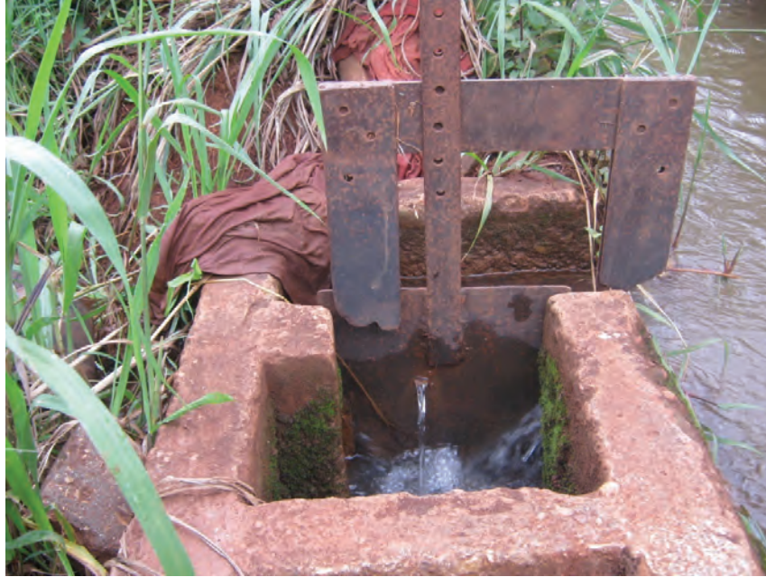
PLATE 3.17: Iron gates, which regulate the flow into the concrete furrows and close off the flow when the furrow is not in use, are either missing or in poor condition
