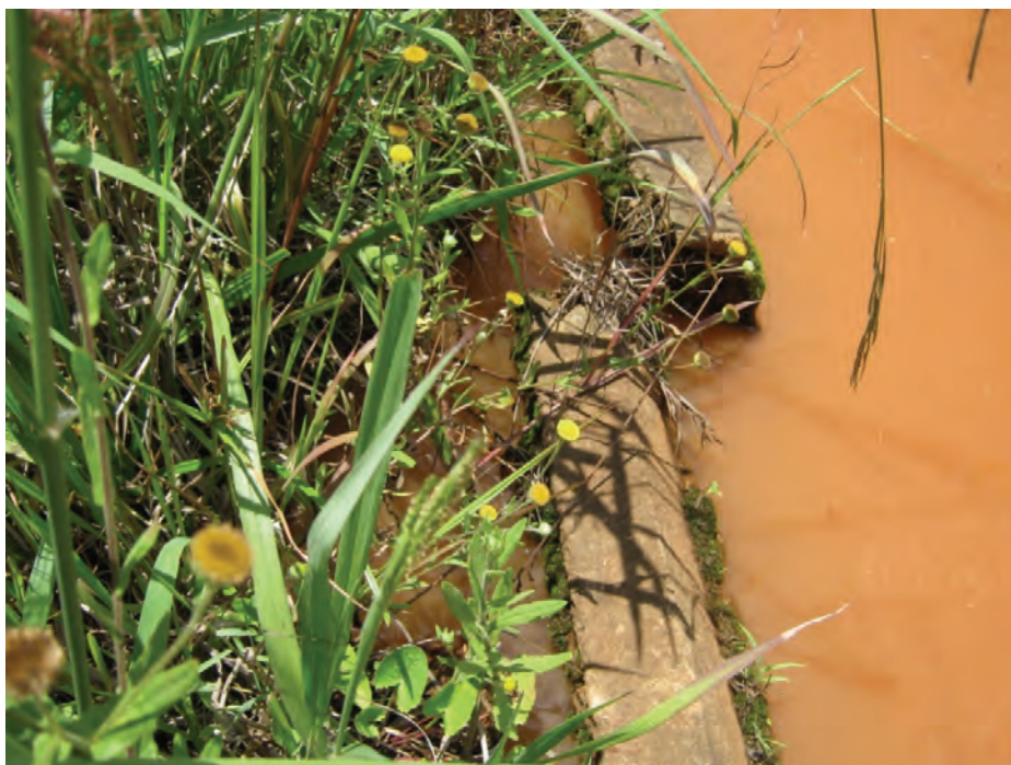
PLATE 3.5: Two canal segments that are no longer aligned
