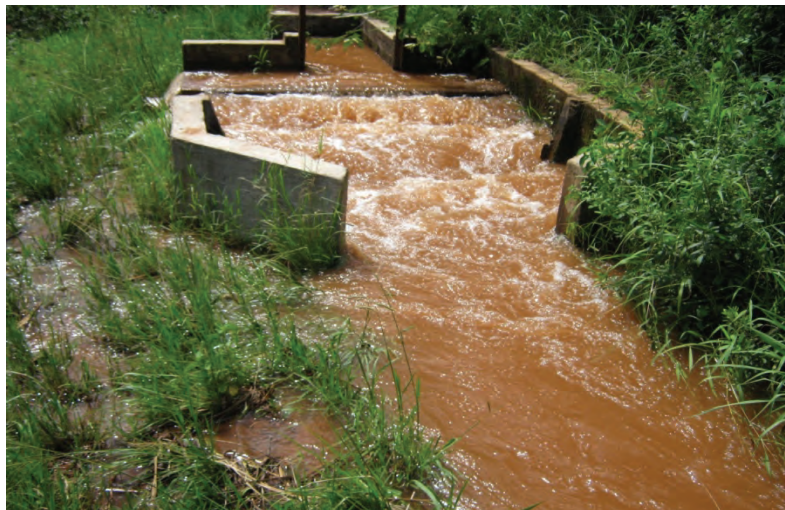
PLATE 3.15: The dysfunctional Chipoletti weir located about 50 m below the river diversion causes the water level in the canal to be too high during periods of high rainfall and strong river flow
