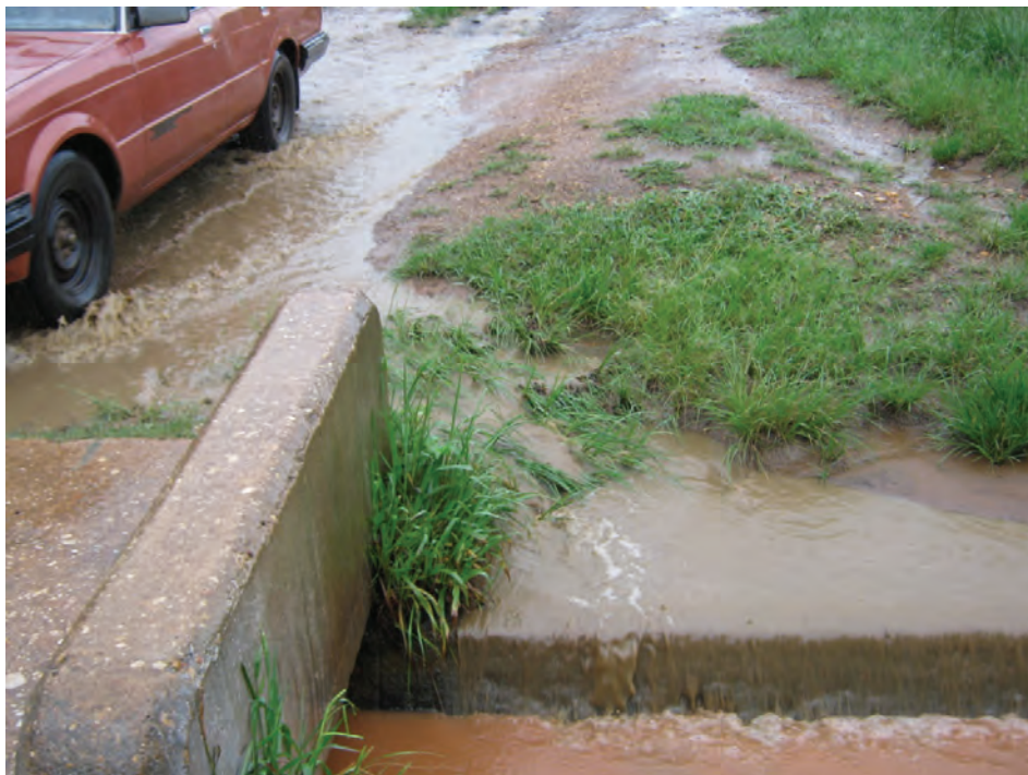
PLATE 3.19: Rain water carrying sediment enters the canal
