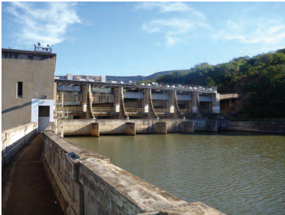
The sluice-gates at Nagle Dam which, when closed, reduce downstream flows and affect the rights of downstream users (Penny Rees)
