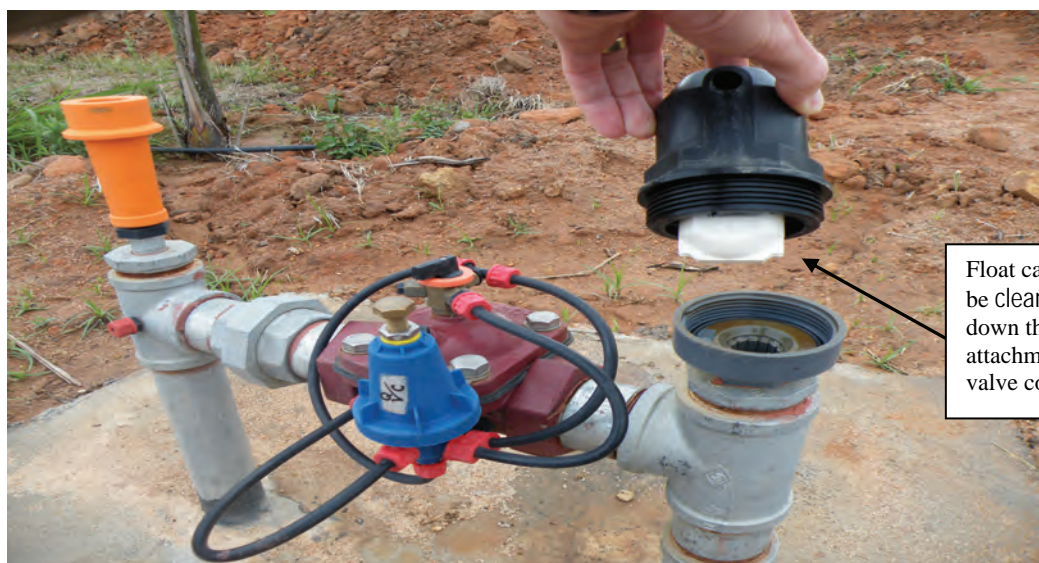
Figure 9. Opening a 25 mm plastic air valve to clean
