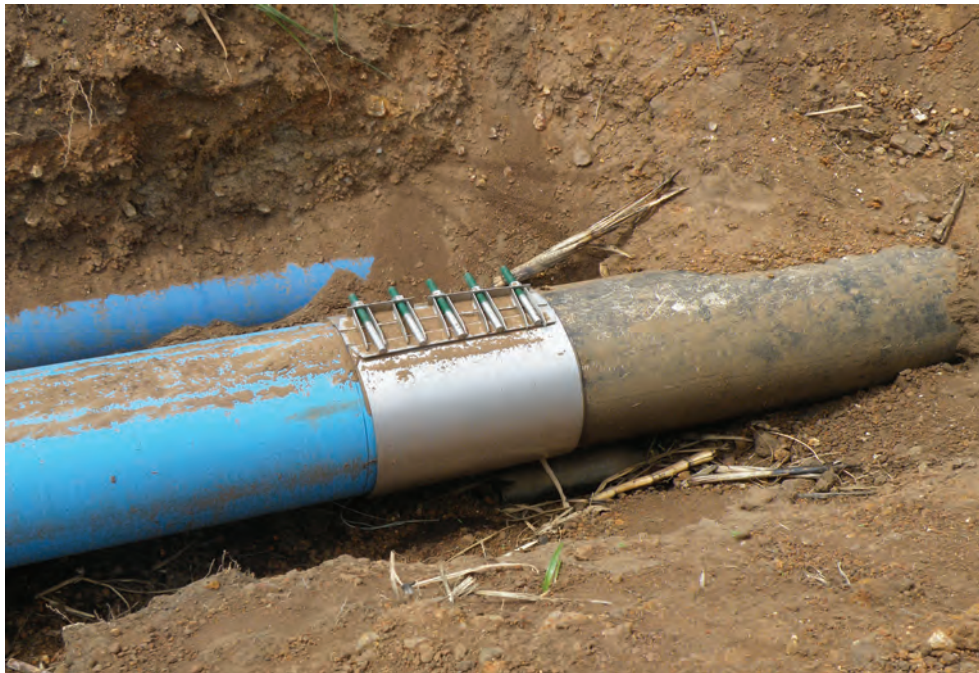
Figure 2. PVC and asbestos pipe coupled with cascade clamp
