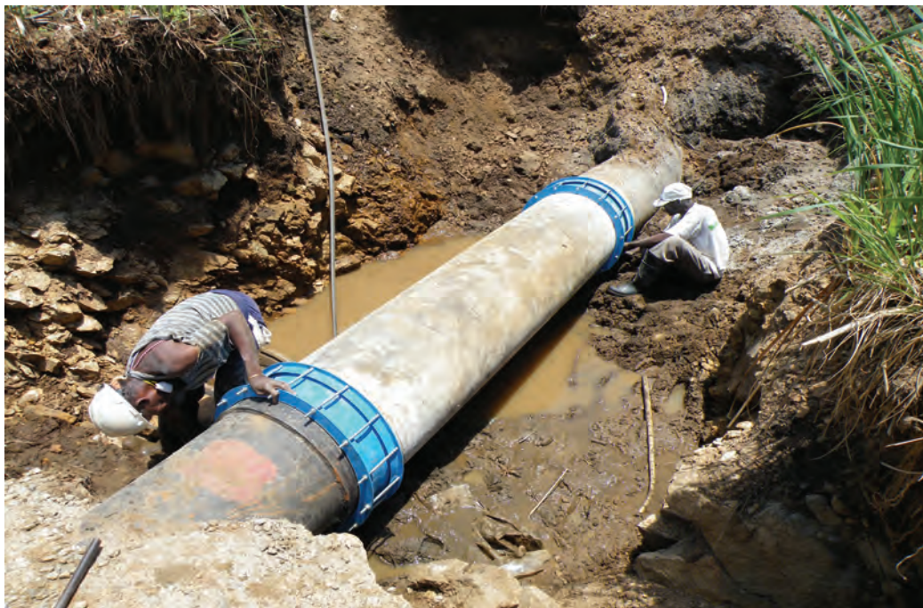
Figure 1. Concrete pipes being repaired with VJ couplings
